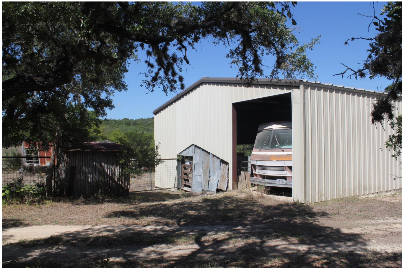
Photo 50. Camera facing Northwest Barn
