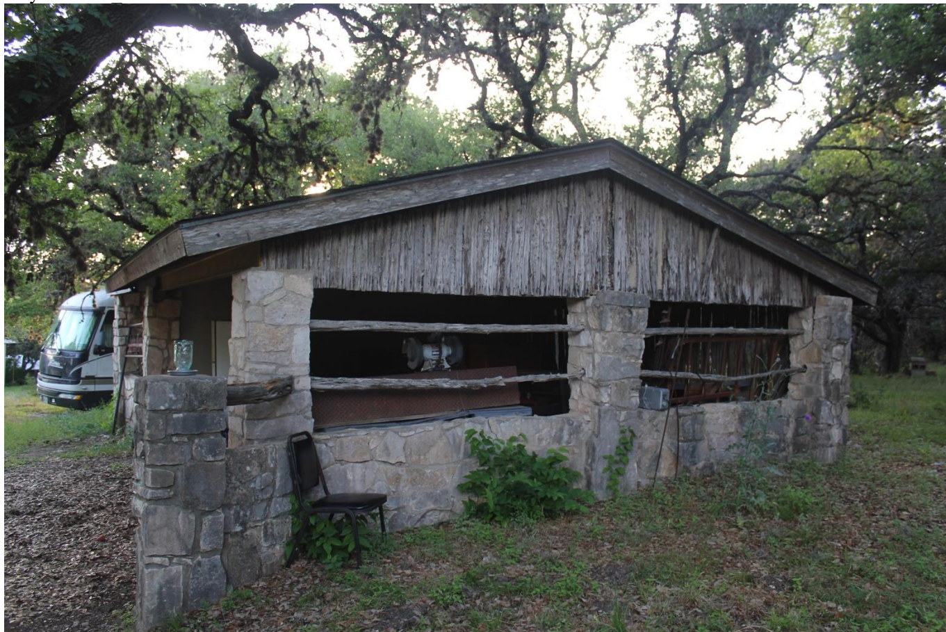
Photo 36. Camera facing West Guy's House East elevation
