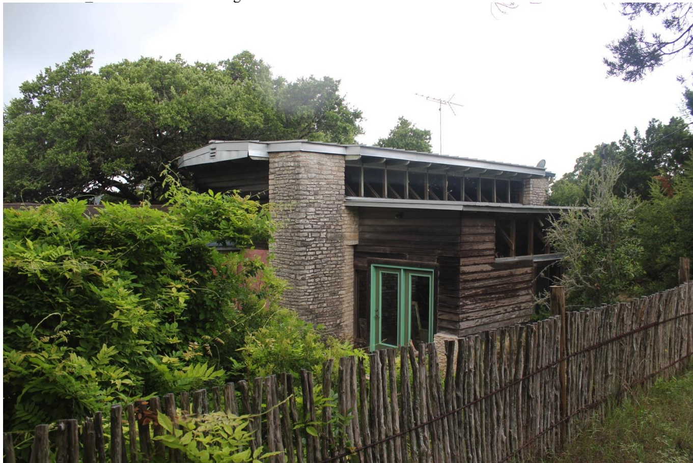
Photo 4. Camera facing Southwest Studio-House_North elevation showing studio levels
