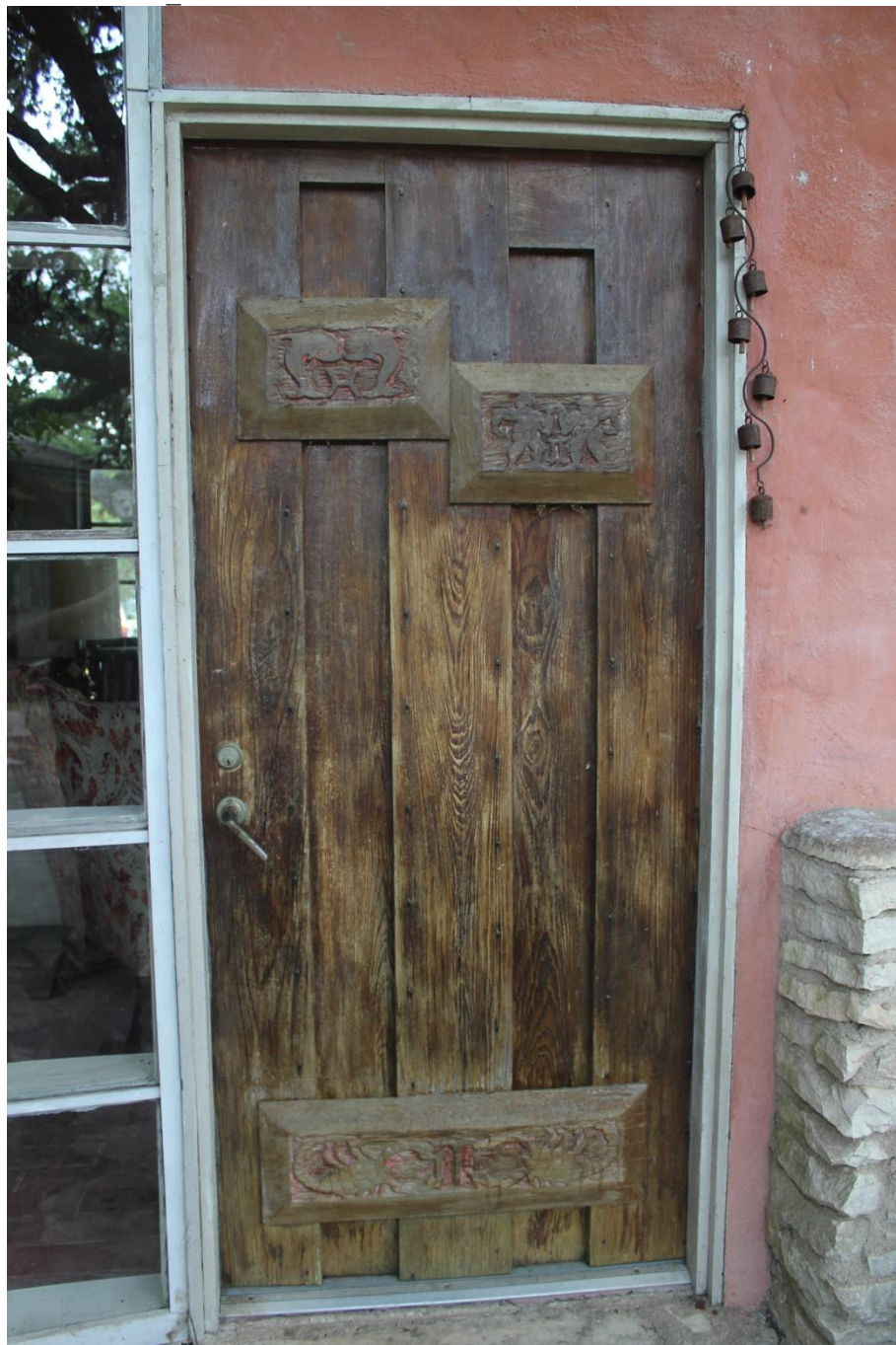
Photo 10. Camera facing East Studio-House Carved door
