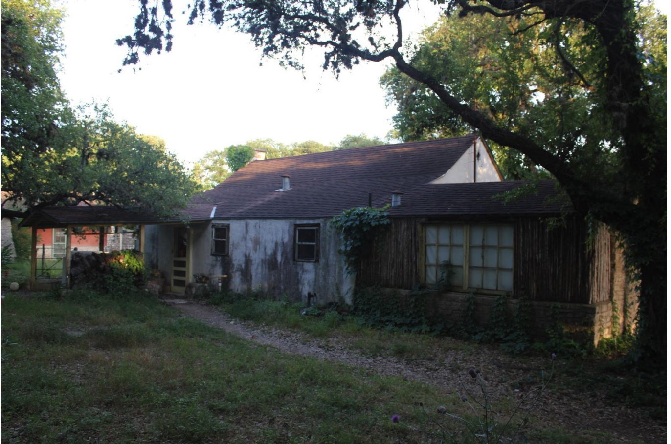
Photo 31. Camera facing Southeast Pierce House_ Northwest corner
