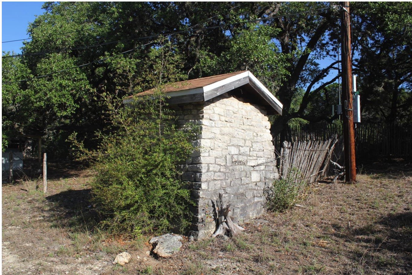
Photo 42. Camera facing Northwest Well House
