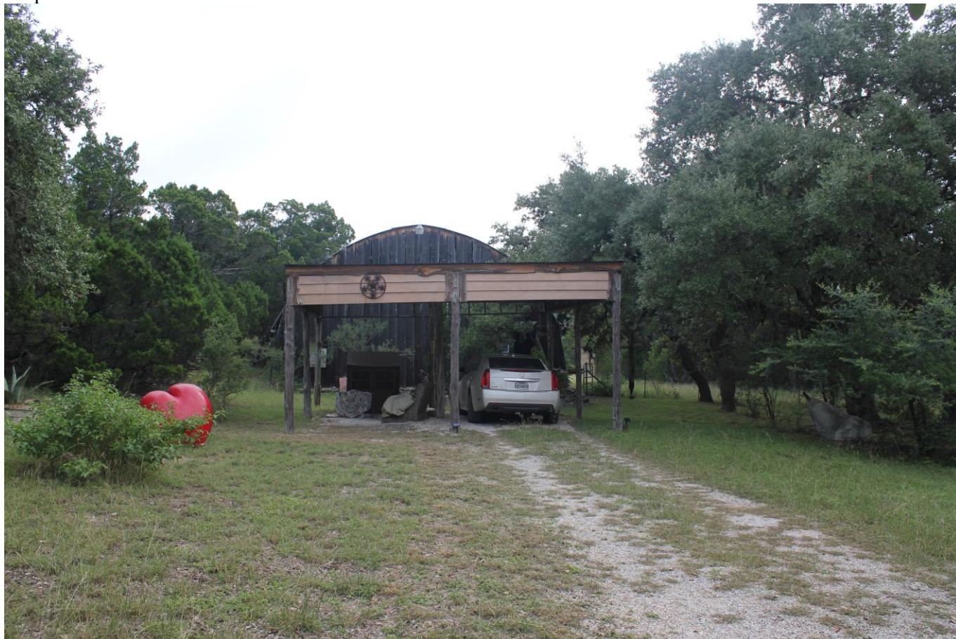
Photo 44. Camera facing East Carport
