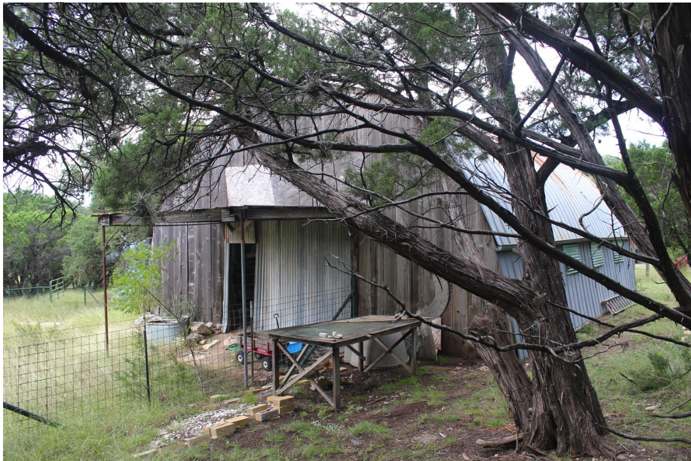
Photo 24. Camera facing Southwest Studio B Northeast corner
