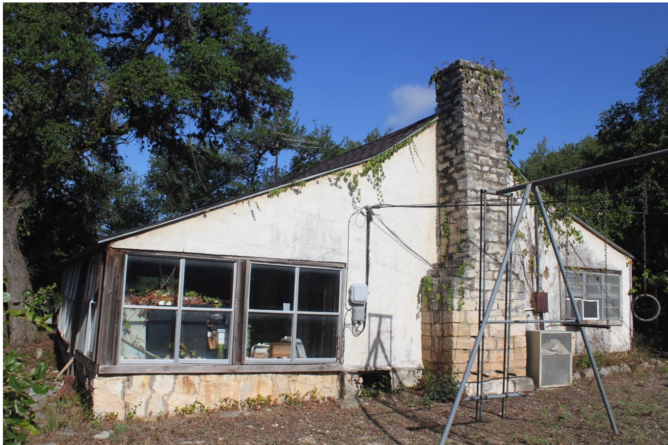
Photo 28. Camera facing West Pierce House East elevation
