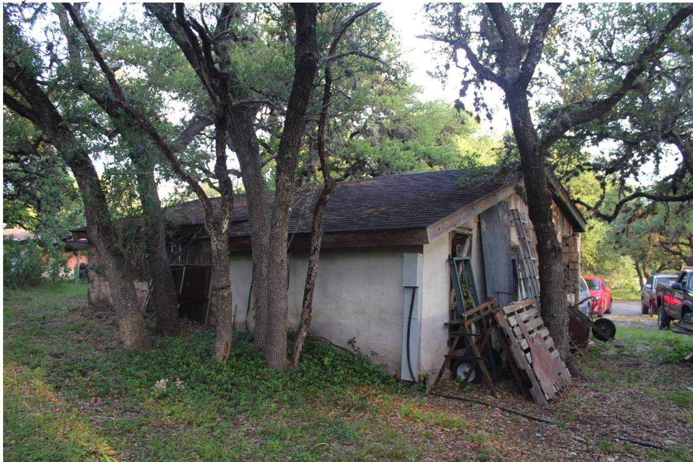
Photo 39. Camera facing Southeast Guy's House Northwest corner
