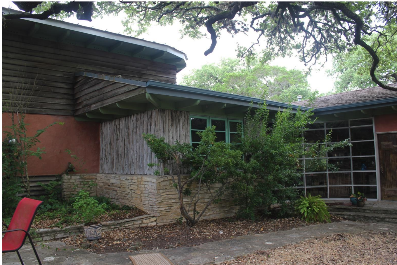
Photo 8. Camera facing Northeast Studio-House Courtyard east wing
