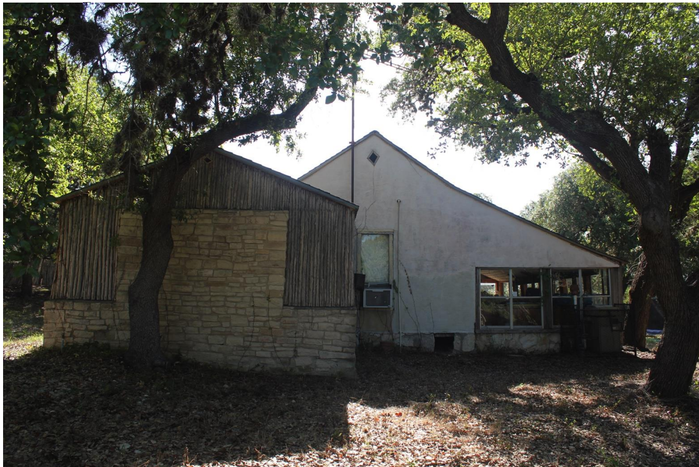
Photo 32. Camera facing East Pierce House West elevation
