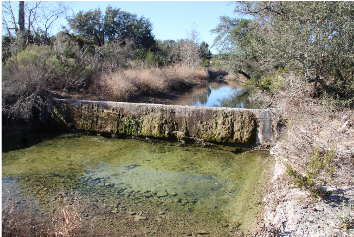
Photo 52. Camera facing Southwest Dam
