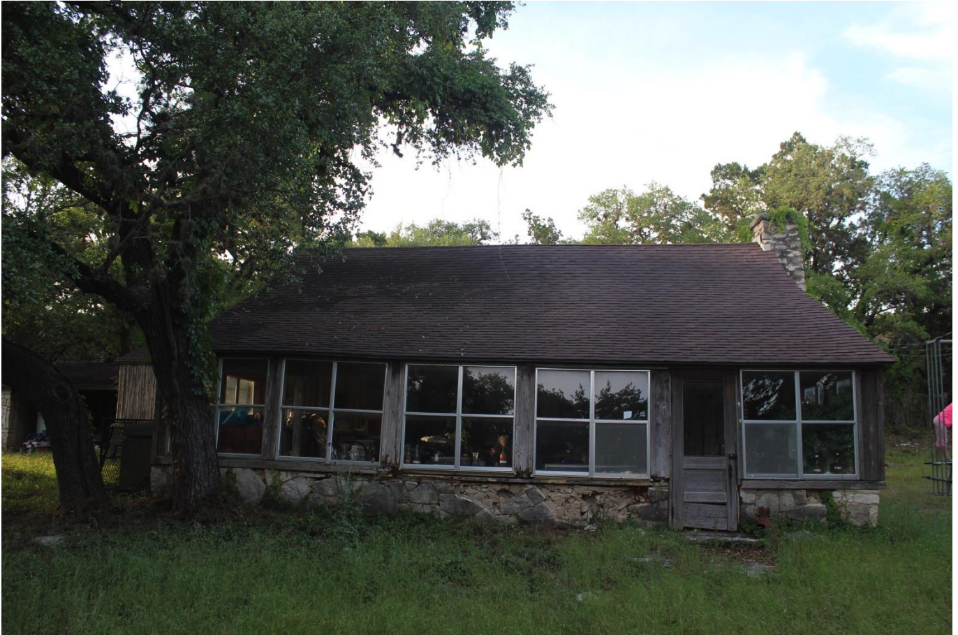
Photo 26. Camera facing North Pierce House South elevation
