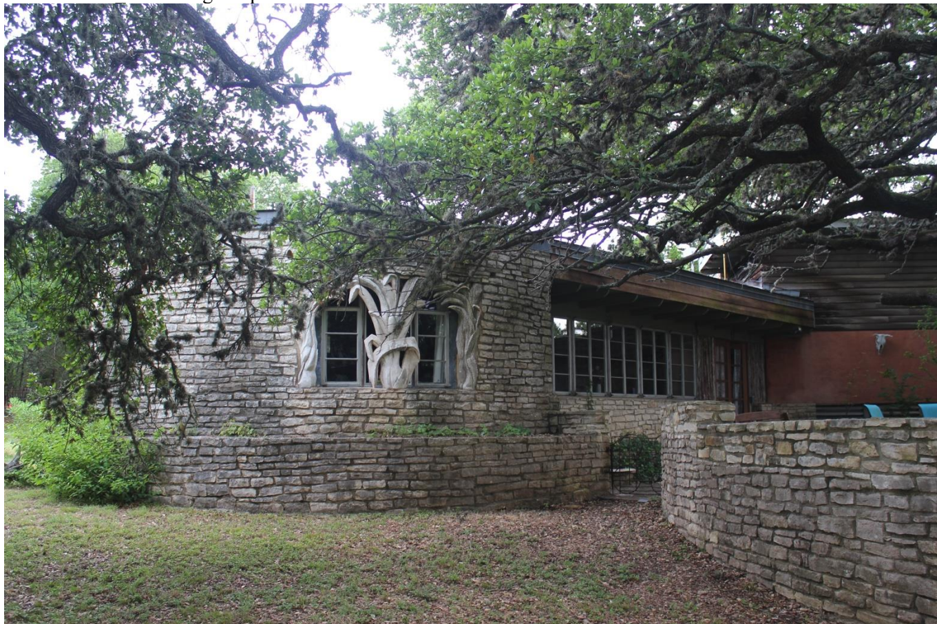
Photo 6. Camera facing Northwest Studio-House West wing sculpted window
