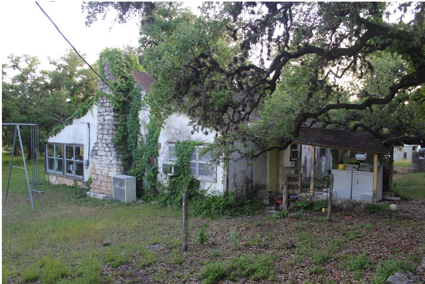
Photo 29. Camera facing Southwest Pierce House_Northeast corner
