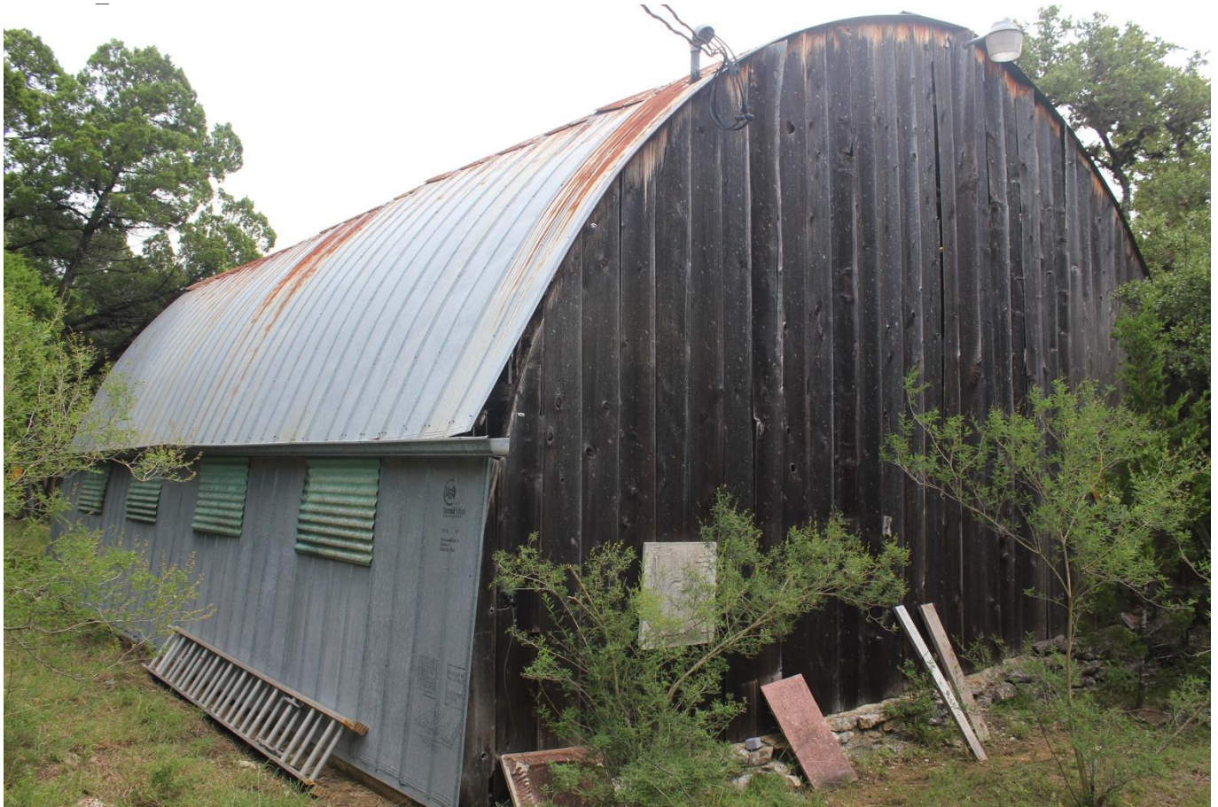
Photo 23. Camera facing Southeast Studio B_ Northwest corner
