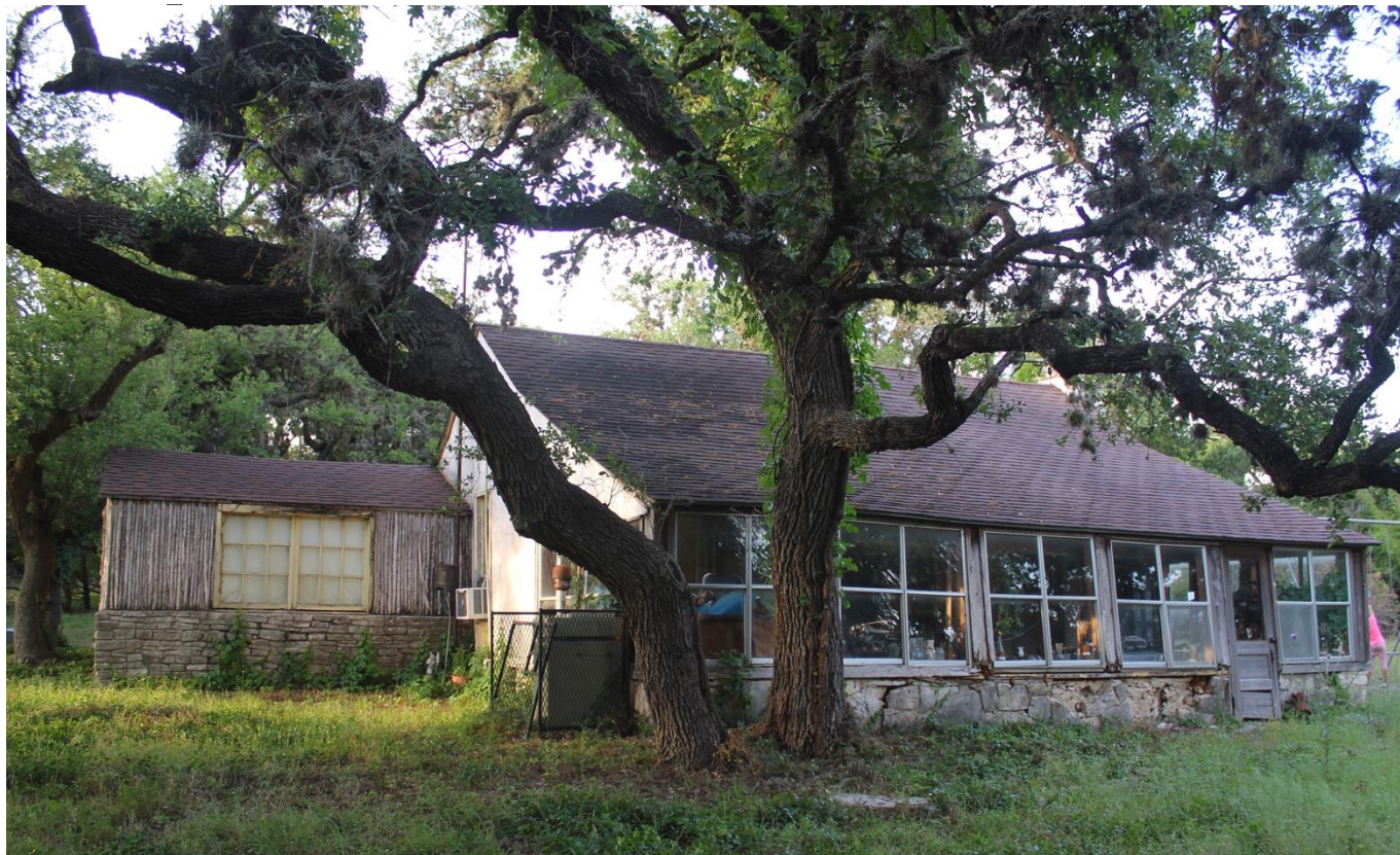
Photo 27. Camera facing Northeast Pierce House Southwest corner
