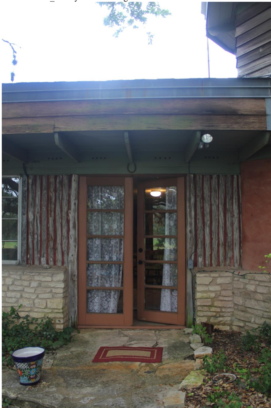
Photo 7. Camera facing Northwest Studio-House_Courtyard west wing
