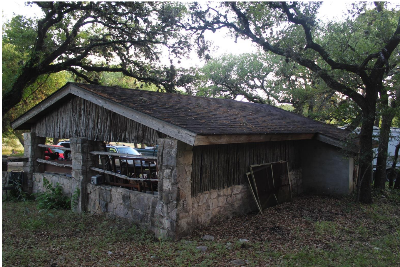
Photo 37. Camera facing Southwest Guy's House_Northeast corner
