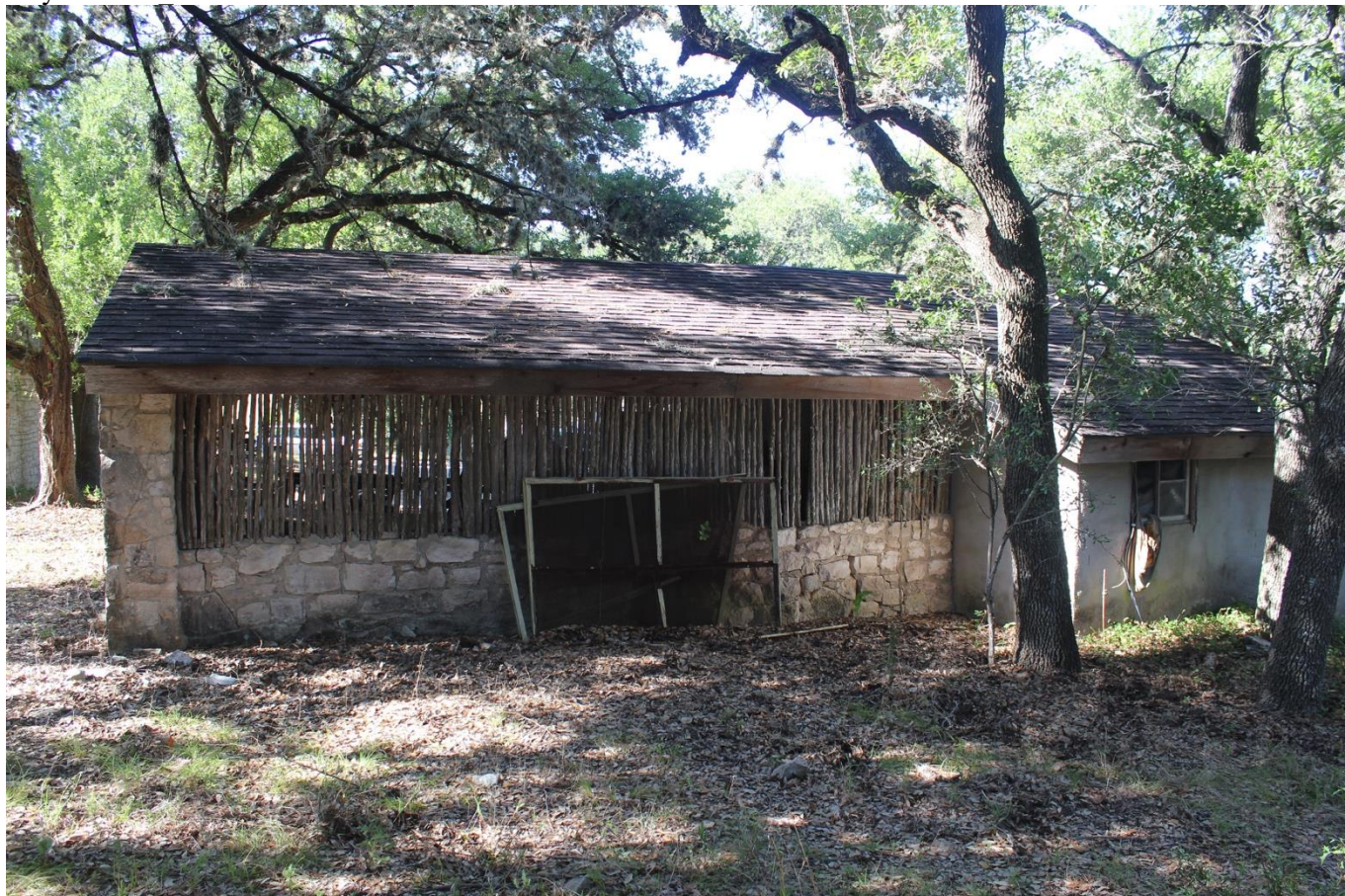
Photo 38. Camera facing South Guy's House North elevation
