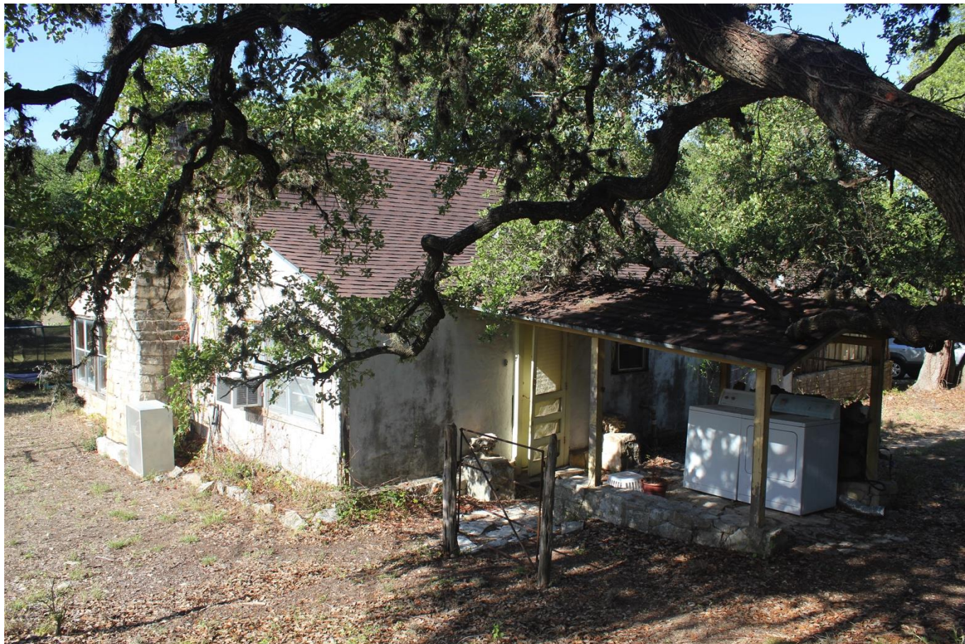
Photo 30. Camera facing Southwest Pierce House Back porch
