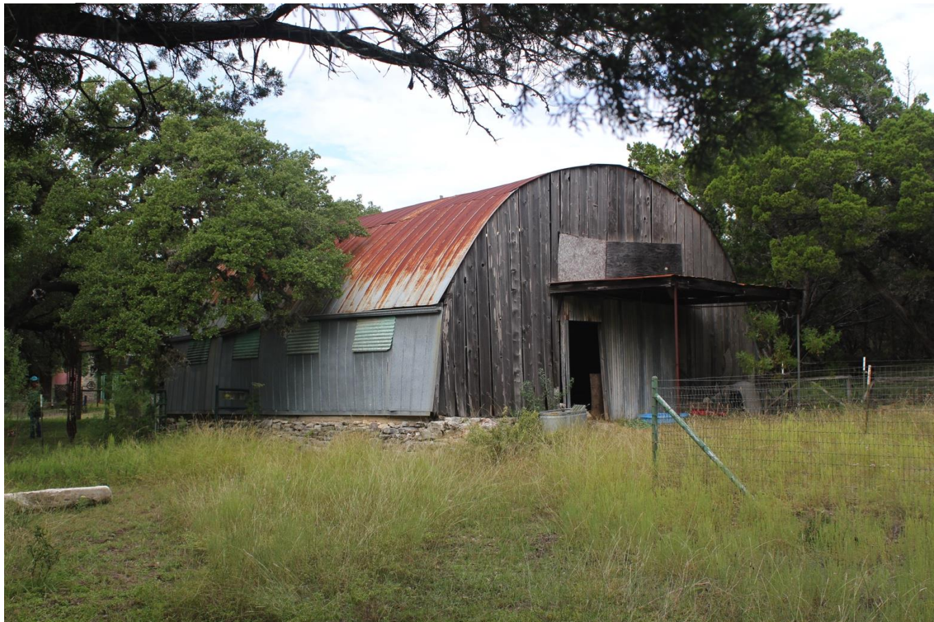
Photo 25. Camera facing Northeast Studio B Southeast corner
