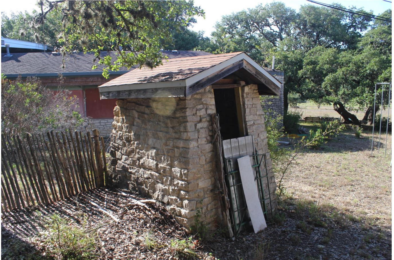
Photo 41. Camera facing Southeast Well House
