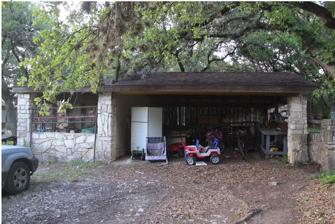
Photo 35. Camera facing North Guy's House South elevation
