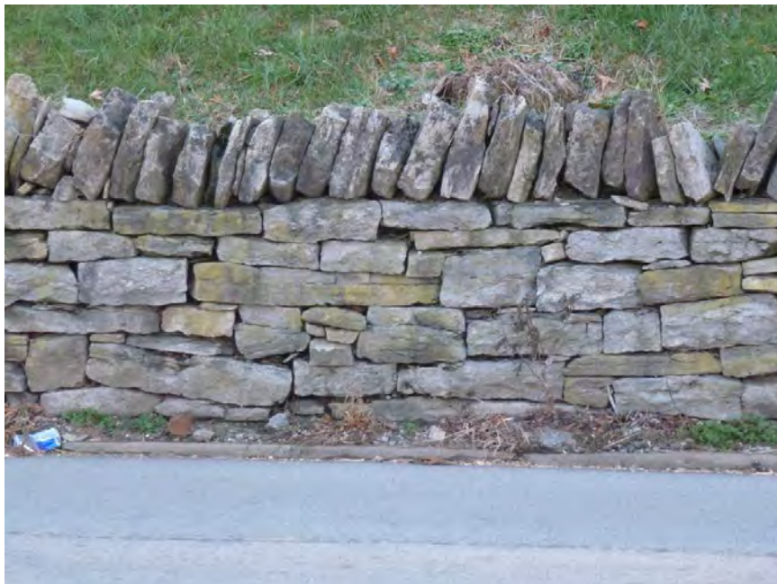
Photo 8: Stone retaining wall
