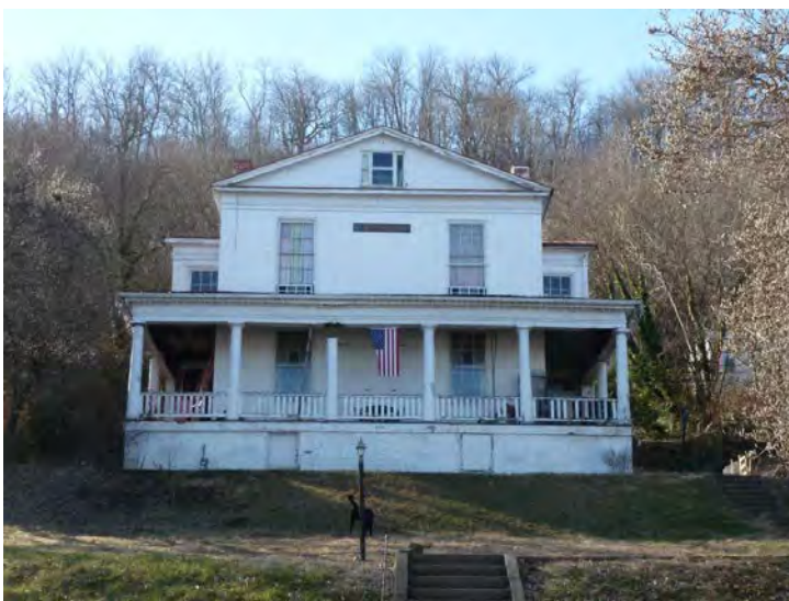
Greek Revival Example, Photo 11
