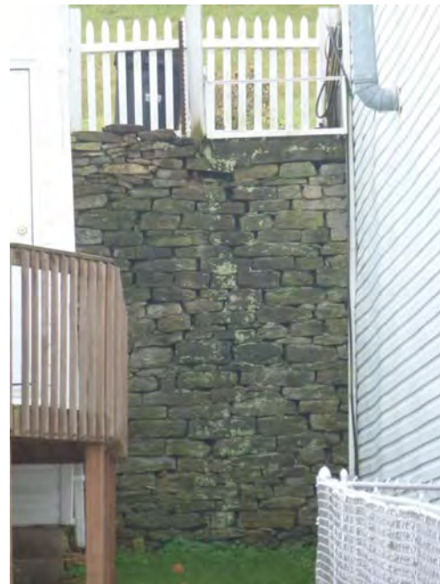
Photo 9: Stone retaining wall
