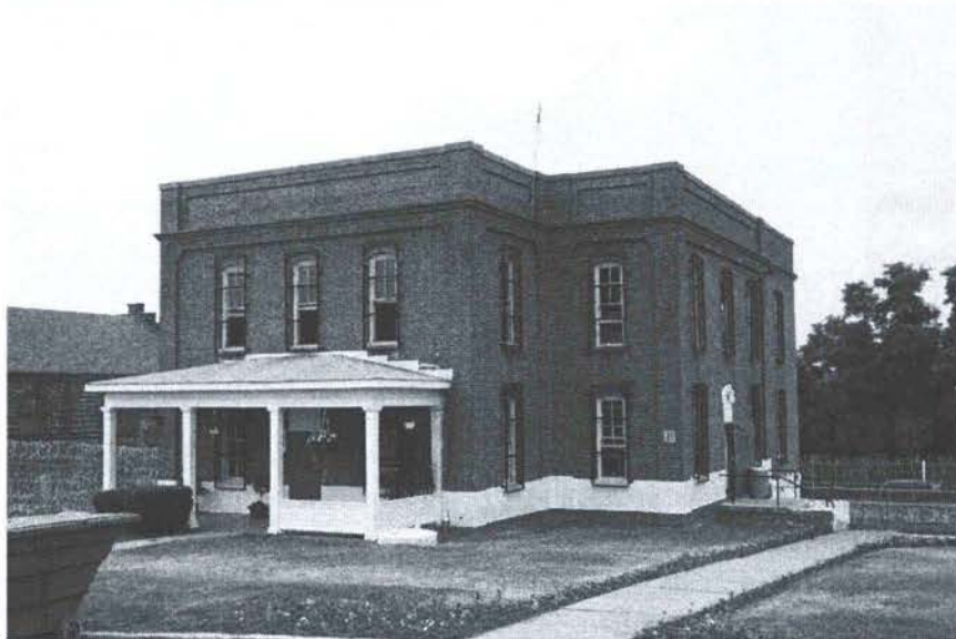
Southeastern Correctional Institution: Hocking Cottage, now B Dormitory, built ca. 1880.
