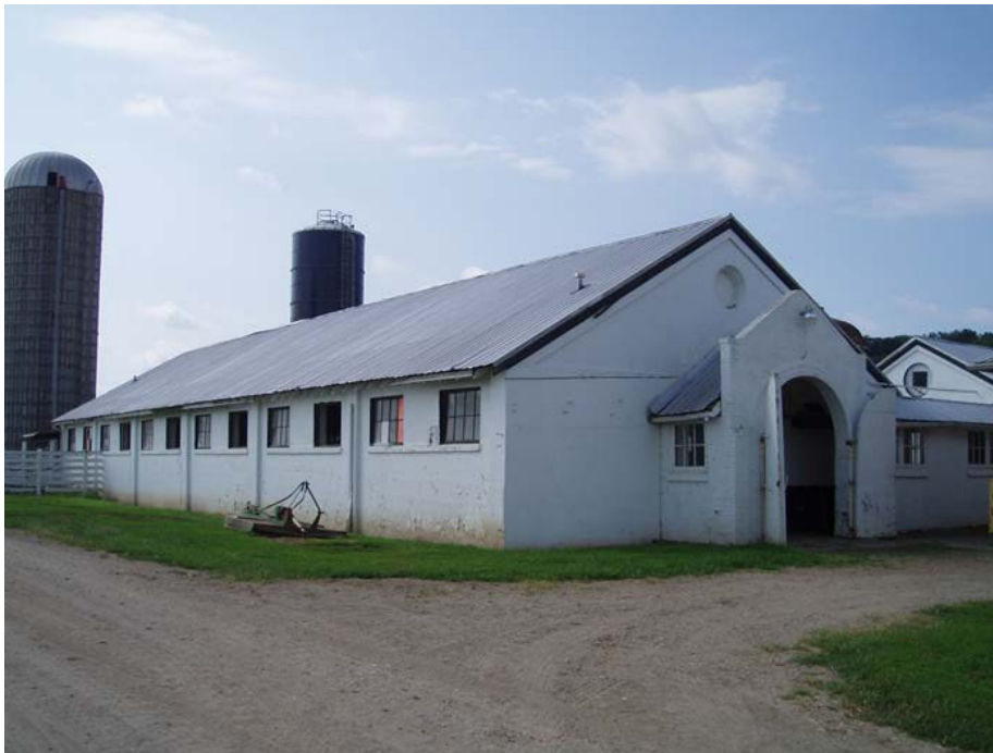
Chillicothe Correctional Institution: One of the barns at the dairy barn complex.
