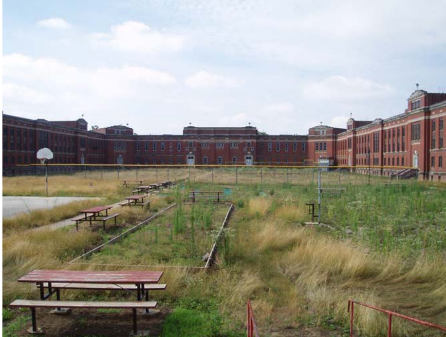
Lima Correctional Institution: Center courtyard, view north.
