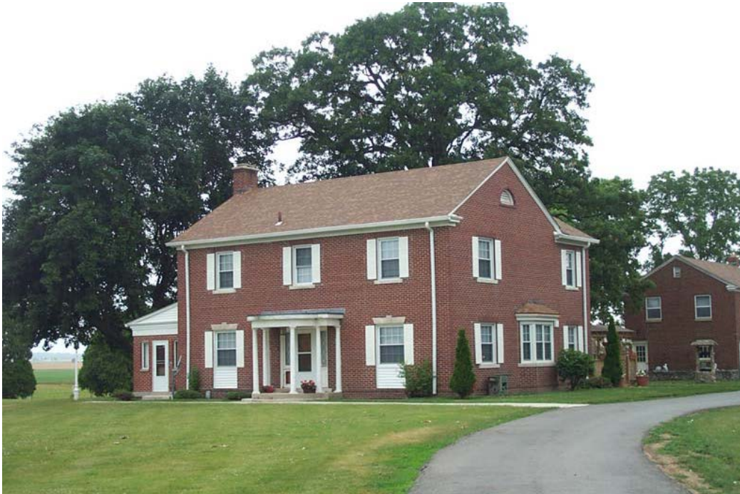
London Correctional Institution: Warden's house.
