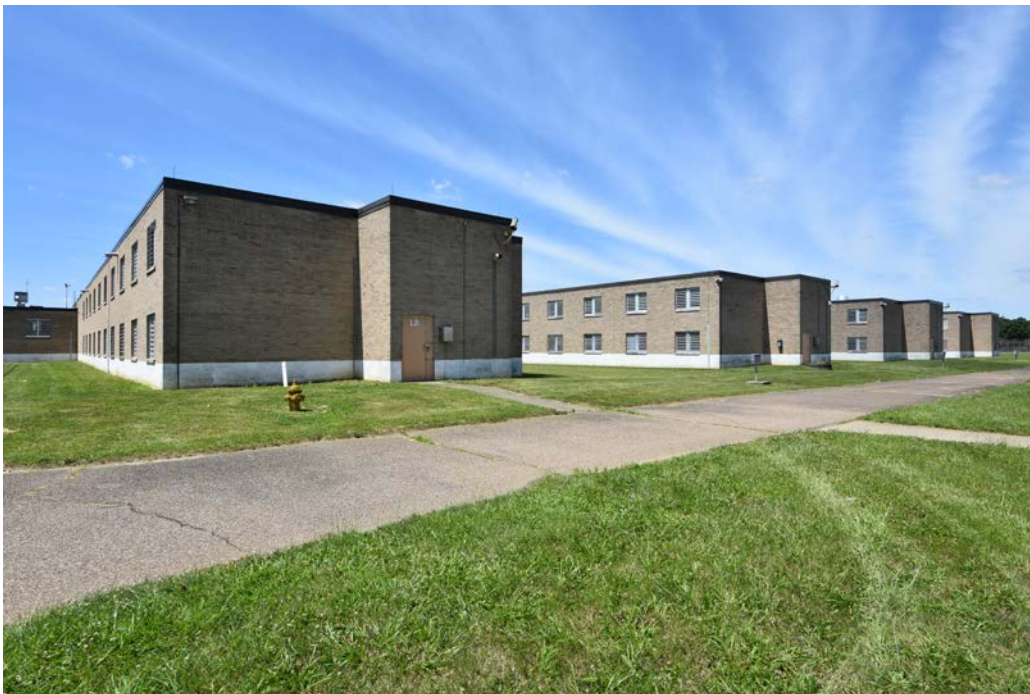
Southern Ohio Correctional Facility, typical cell blocks.
