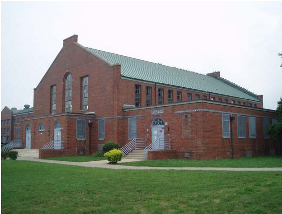
Chillicothe Correctional Institution: Main dining hall.
