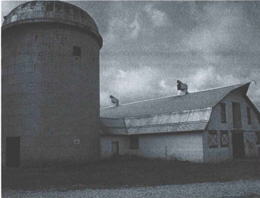
Chillicothe Correctional Institution: Mule barn and hay keeper.
