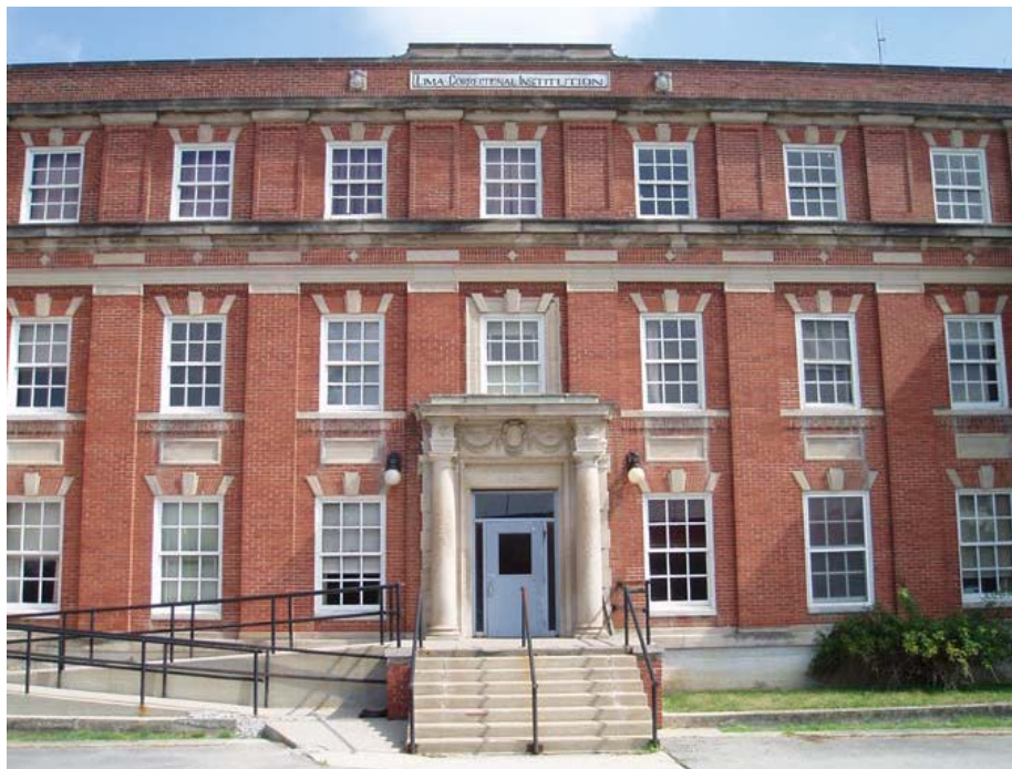
Lima Correctional Institution: Center portion of north facade, administration wing.
