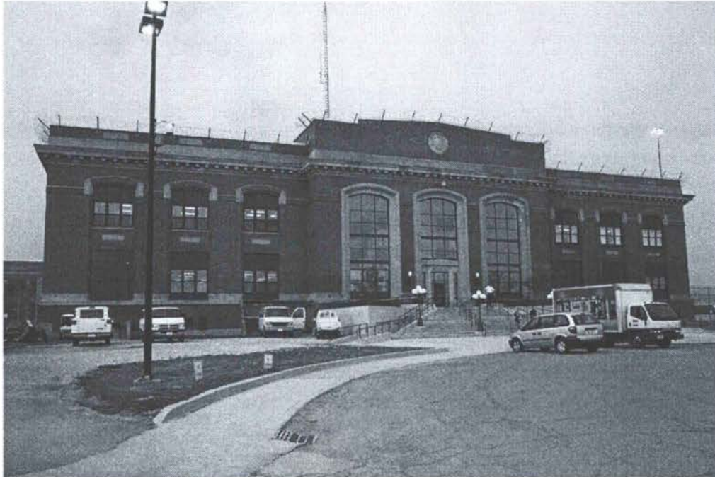
London Correctional Institution: Facade of administration building.
