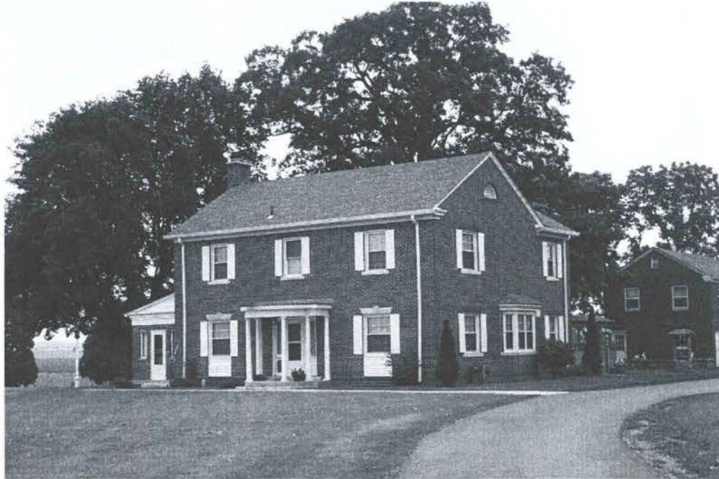
London Correctional Institution: Warden's house.
