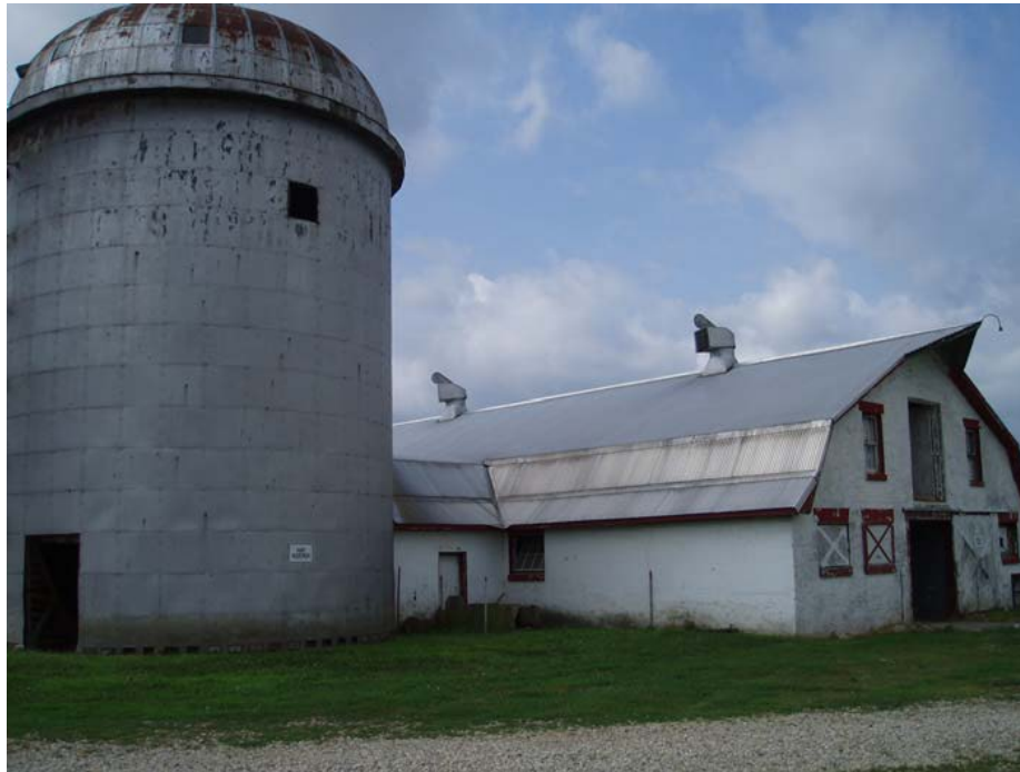
Chillicothe Correctional Institution: hay keeper (non-extant) and mule barn.
