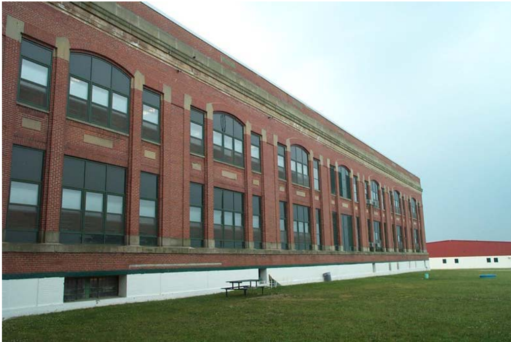
London Correctional Institution: Northwest cross wing of administration building.
