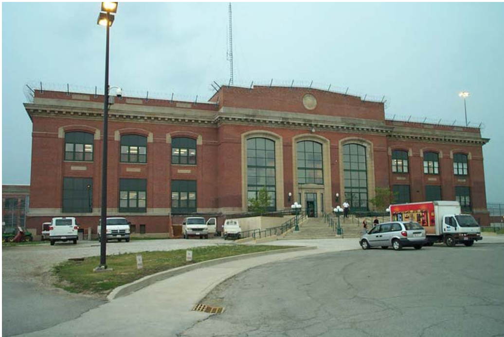
London Correctional Institution: Facade of administration building.
