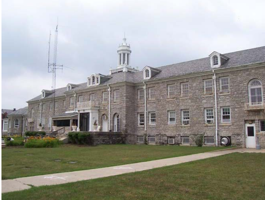
Ohio Reformatory for Women: Main facade of Harmon Building.
