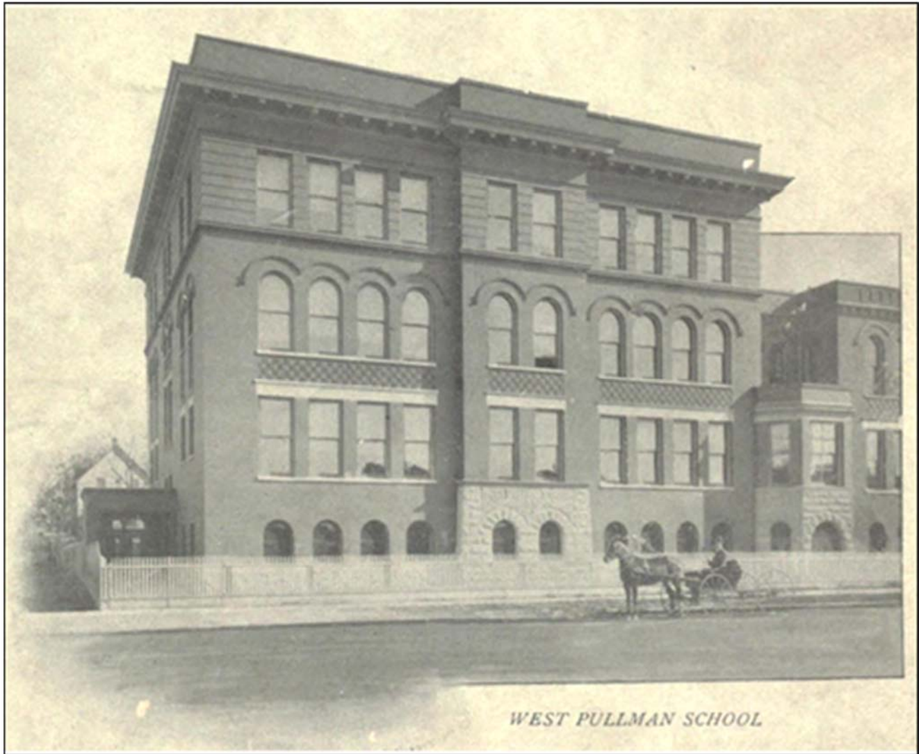
Figure 2: c. 1900 rendering of the West Pullman School Source: West Pullman Land Association, 1900, cover.
