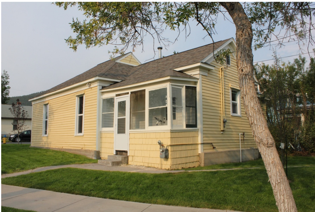
Haight - Bridgewater House, east and north elevations. View to southwest. 0003 of 0007.
