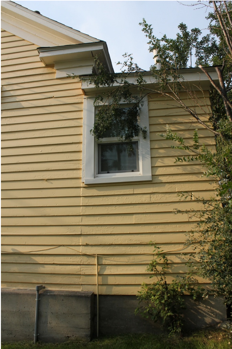
Haight - Bridgewater House, west side of north (rear) elevation. Bathroom addition. View to south.
