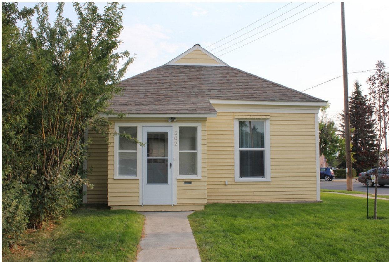
Haight - Bridgewater House, south (front) elevation. View to north. 0001 of 0007.
