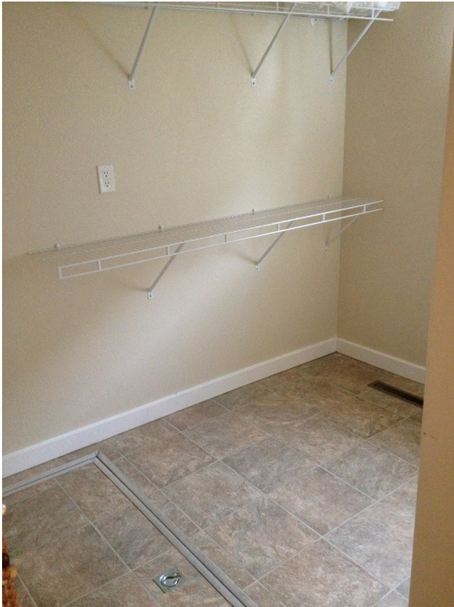
Haight - Bridgewater House utility room view to southeast.
