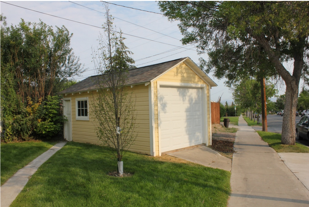
Haight - Bridgewater House garage, south and west elevations. View to northeast. 0006 of 0007.
