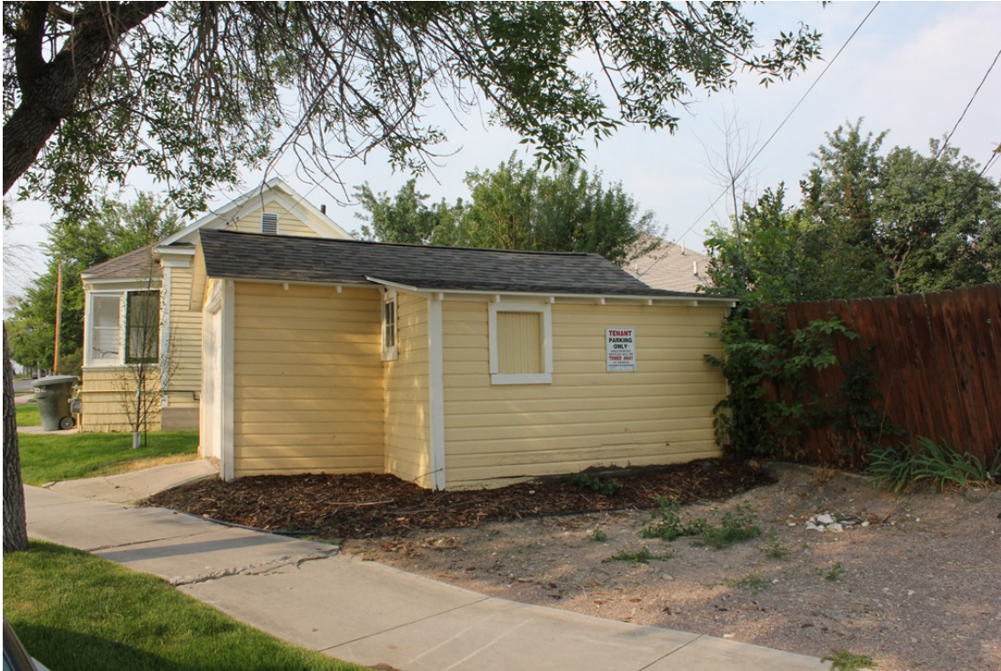
Haight - Bridgewater House garage, north elevation. View to south-southeast. 0007 of 0007.
