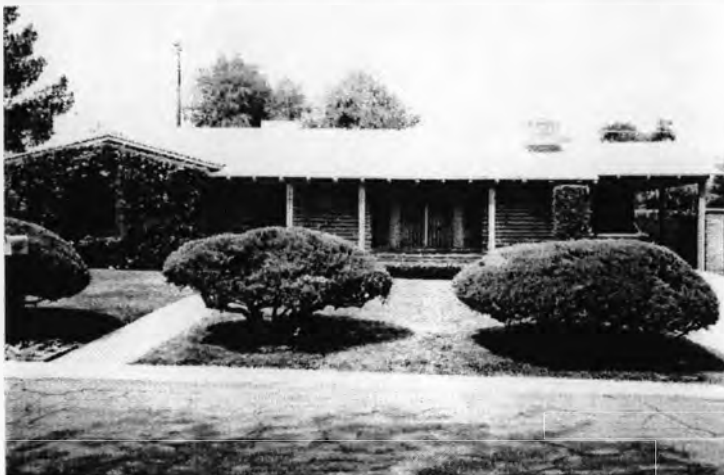
Traditional Ranch with burnt adobe walls (Site 262)
