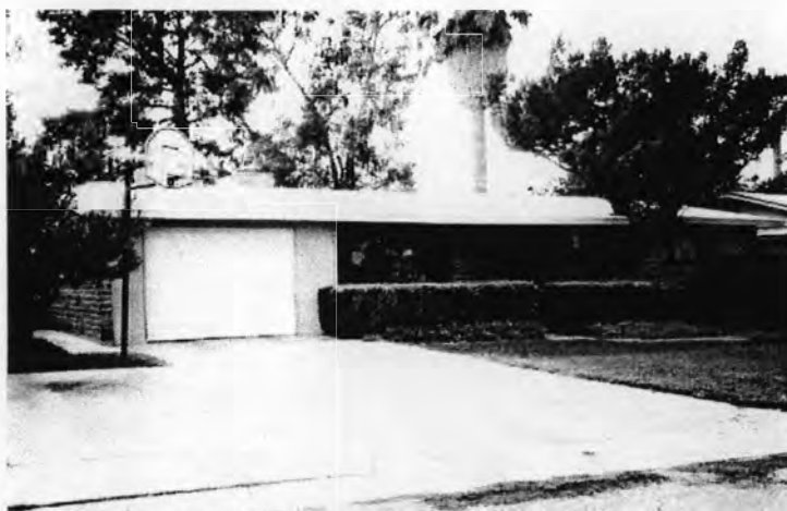
Incompatible Conversion of Carport into Garage (Site 186)
