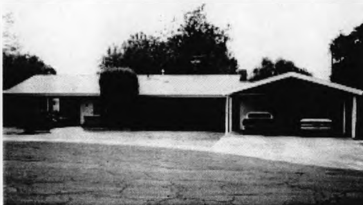
Incompatible Carport Enclosure and Extension (Site 97)
