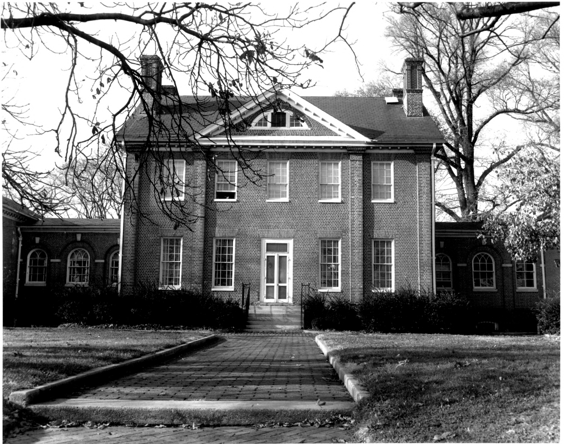
Mount Clare, Baltimore, Maryland - East (rear) elevation.
