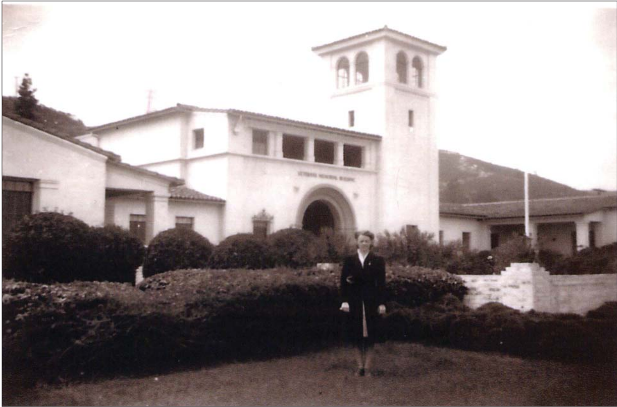
Main facade, view looking southwest, n.d.
