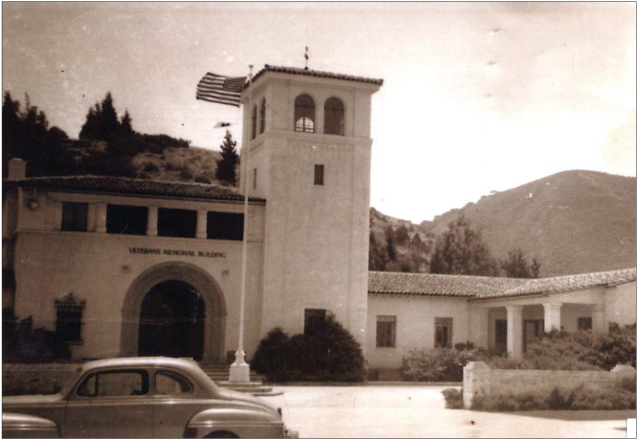
Main facade, view looking southwest, n.d.
