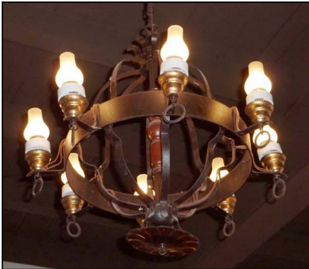
Incandescent lamps in this Lobby chandelier have been replaced with fluorescent bulbs.
