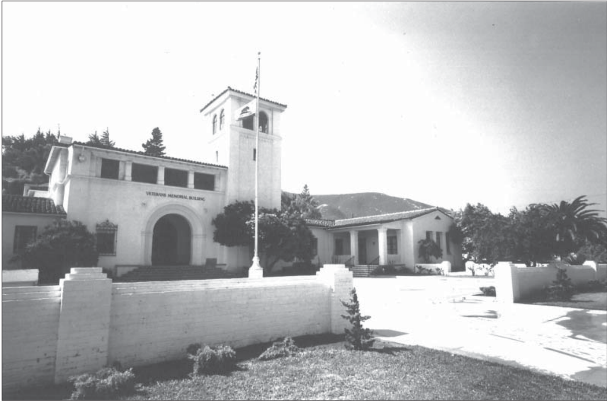
Main facade, view looking southwest, n.d.
