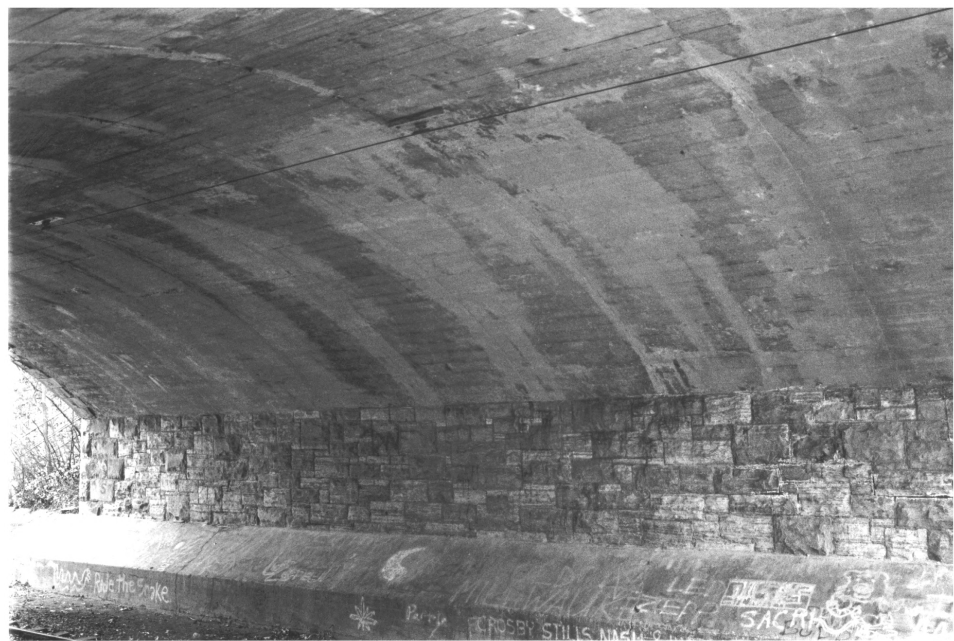
BRIDGE NO. L-9328 HENNEPIN CO., MN PHOTO I.D. 09740 # 22
