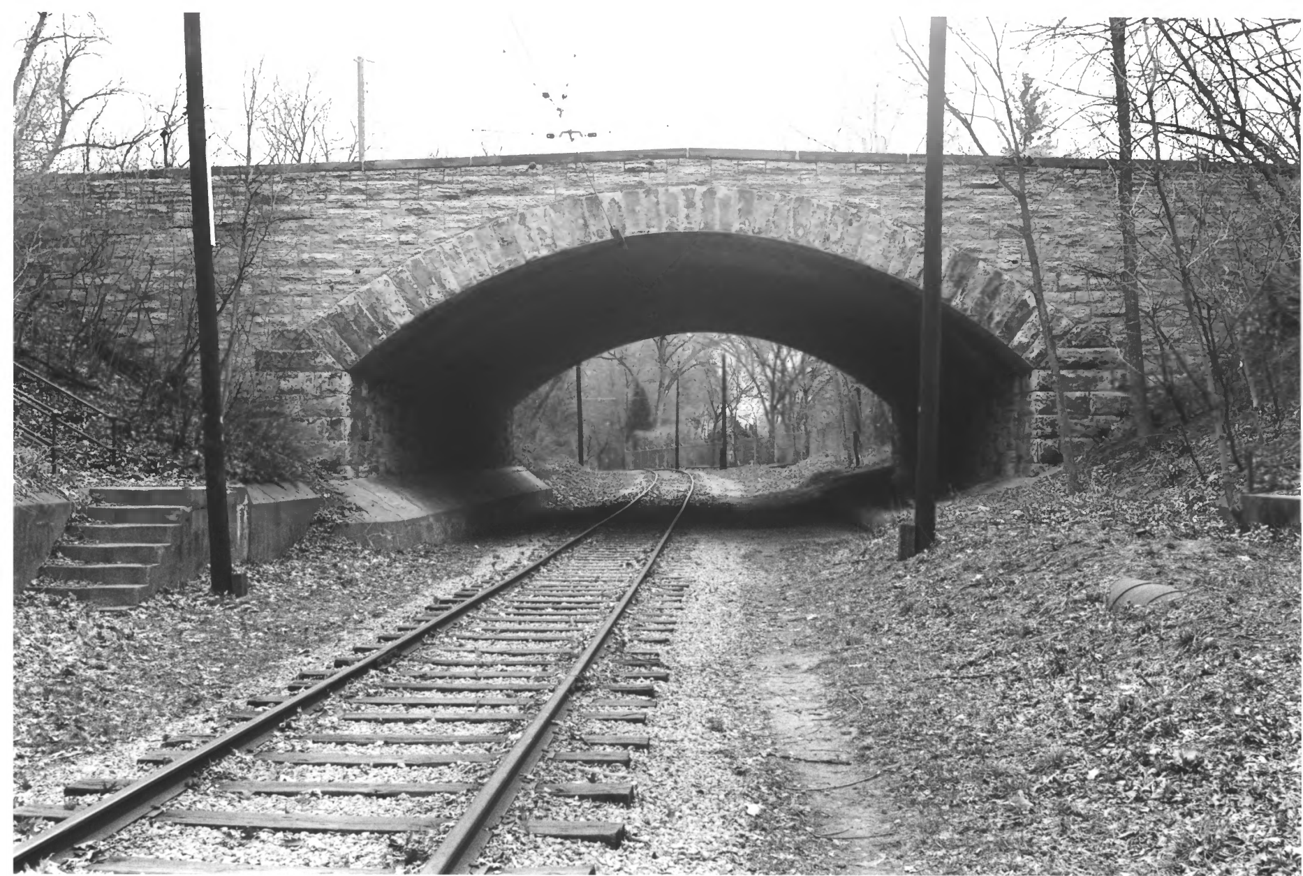
BRIDGE NO. L-9328 HENNEDIN CO. MN PHOTO I.D. 09740 # 20
