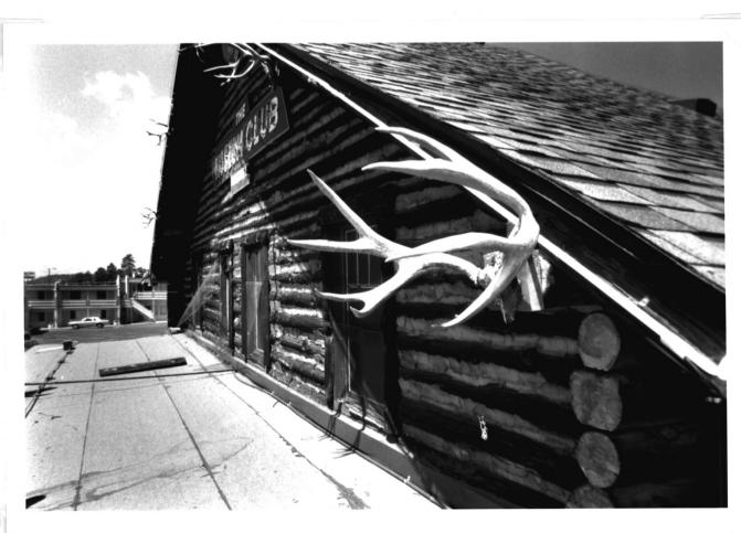
Log construction is visible throughout the interior. Corners frequently show the saddle notches used to stack the logs.
