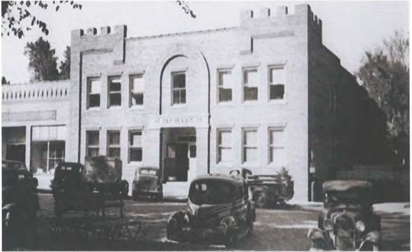
Figure 3: Villisca National Guard Armory, 1930's (Source Unknown)
