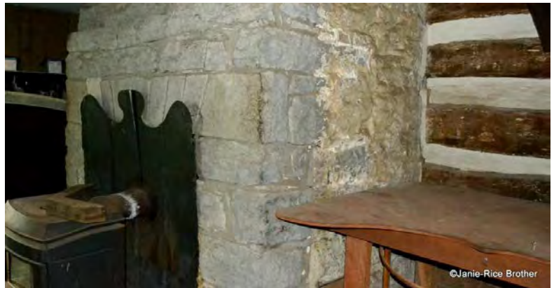
Stone chimney stack in East pen (photo 10)
