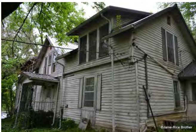
Main façade (photo 4)
