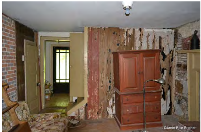
Stair to upper level (photo 12)
