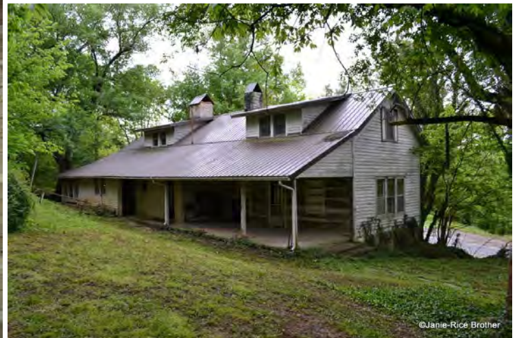
Rear and west elevations (Photo 2)
