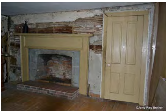
Montgomery-Sandidge House, Photo 11
