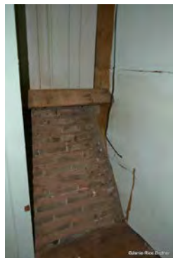
Chimney-stack shoulder
