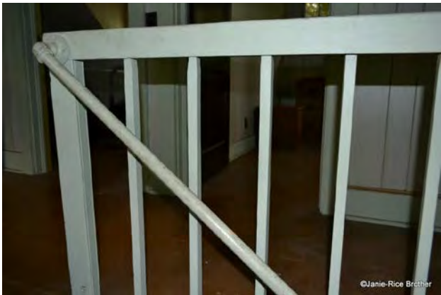
Federal-era balusters, West pen (photo 14)
