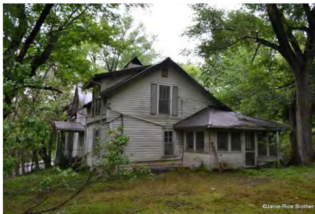
East elevation, enclosed porch and milk chiller area (Photo 5)
