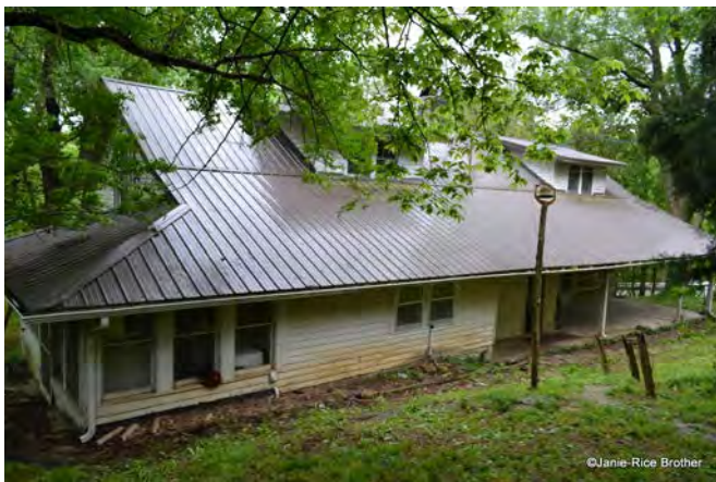
Rear/North Elevation (Photo 6)
