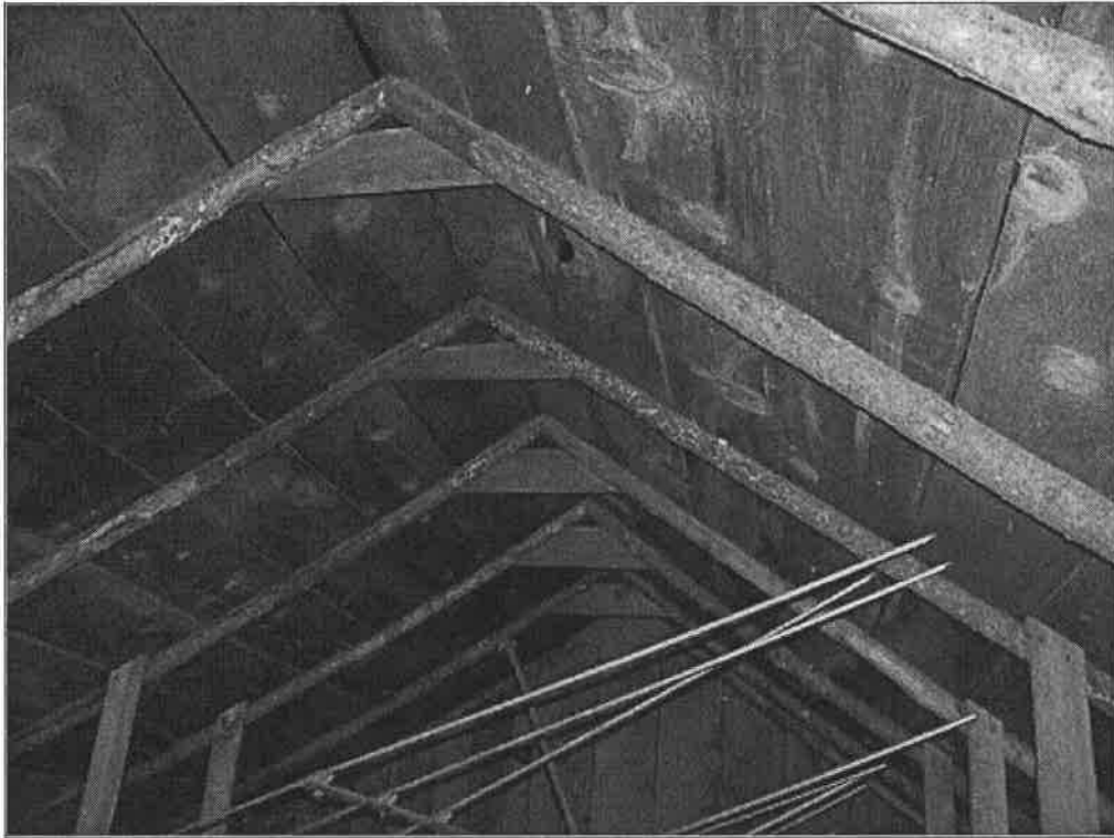
Photo 9 of 20: Attic of Main Cabin, looking east.
