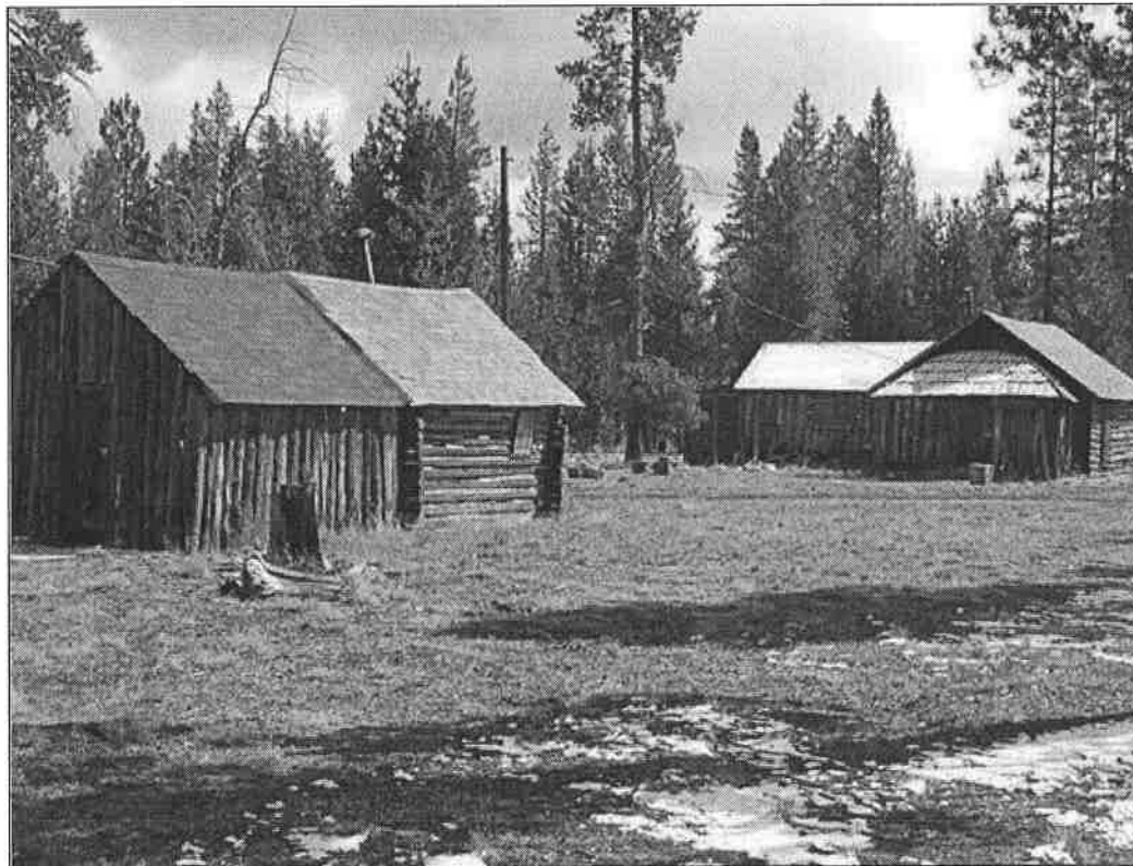
Photo 2 of 20: Woodshed at the rear of the guest cabin in the foreground and the rear of the main cabin in the background, looking northeast.
