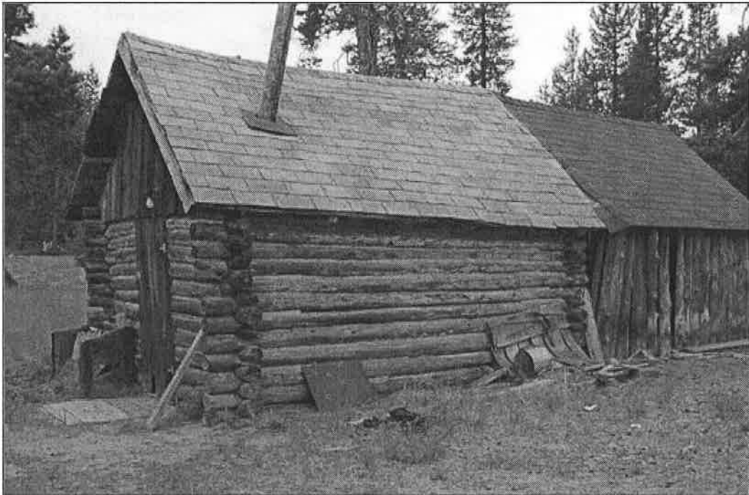
Photo 11 of 20: Guest Cabin, looking southwest.
