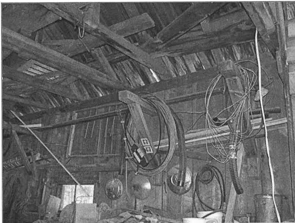
Photo 16 of 20: Interior of Garage, looking northwest.
