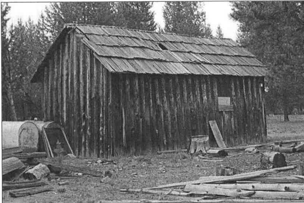
Photo 15 of 20: Rear and south side of Garage, looking northeast.
