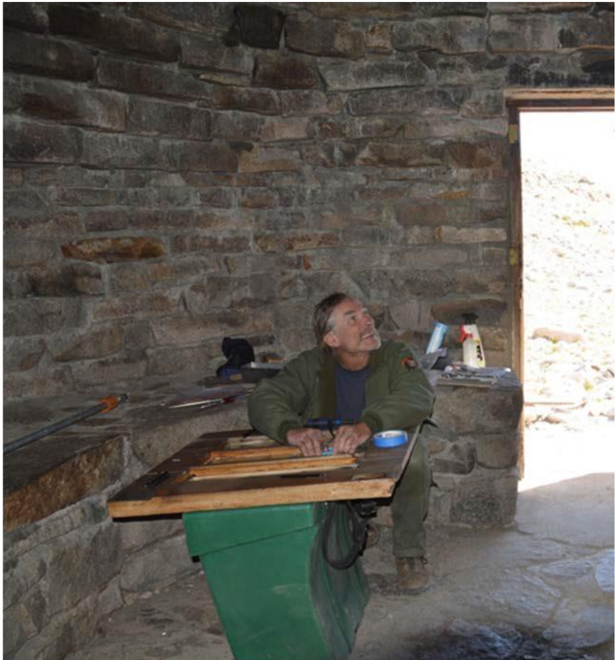
Photo 7. NPS Preservation Crew Leader Thor Rikshiem restoring entry door, July 2014.
