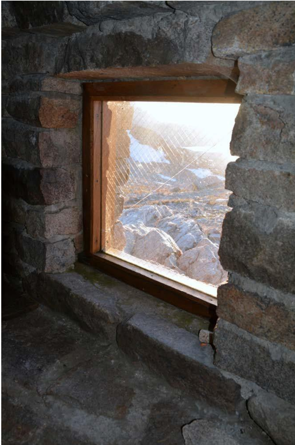
Photo 8. Fixed wireglass window pane and viewshed from shelter, 2015.
