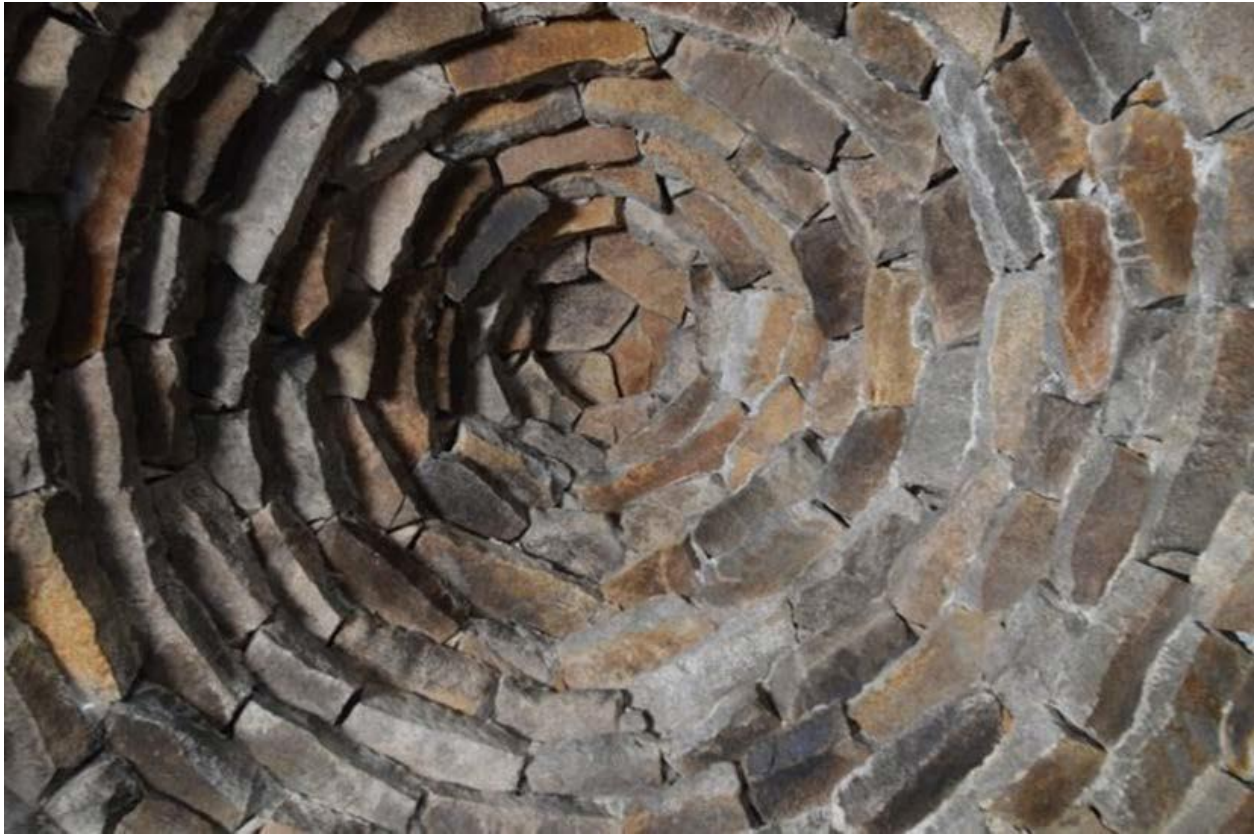
Photo 6. Corbelled granite conical ceiling detail, 2015.
