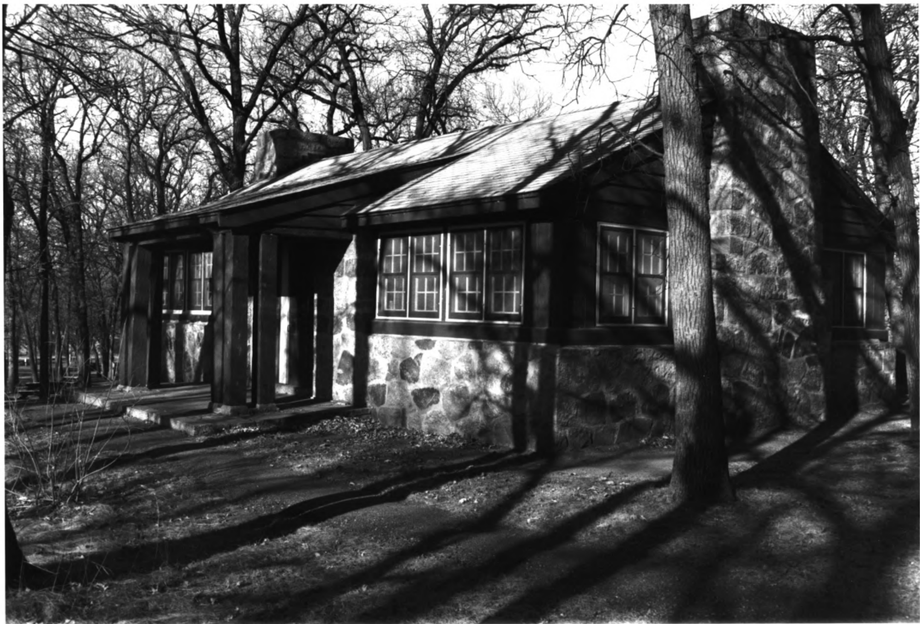
SIBLEY STATE PARK, CAMPGROUND SHELTER KANDIYOHI CO., MN BLDG # 9 PHOTO I.D. 09124#15
