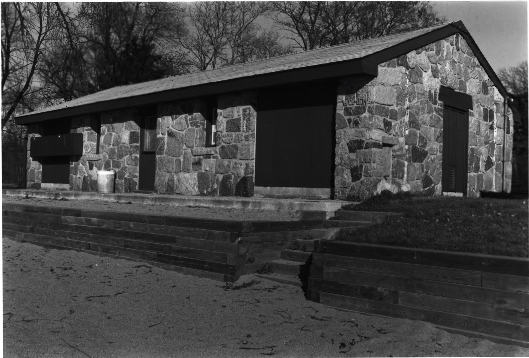
SIBLEY STATE PARK, Bath House KANDIYOHI CO., MN BLDG # 6 PHOTO I.D. 09124# 23
