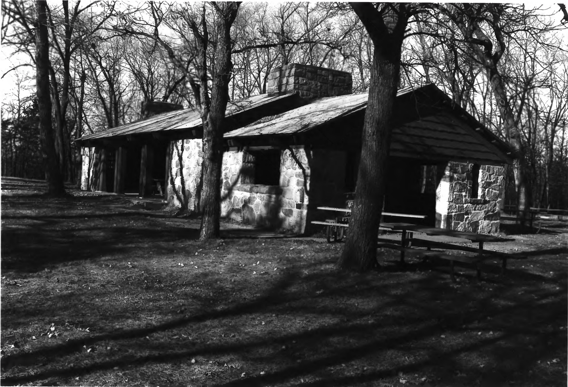
SIBLEY STATE PARK, SHELTER PAVILION KANDIYOHI CO., MN BLDG # 1 PHOTO I.D. 09123 # 4
