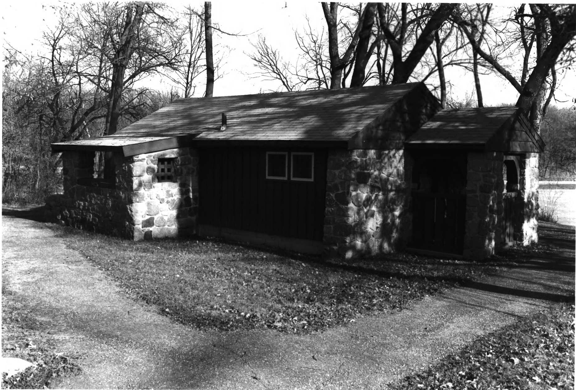
SIBLEY STATE PARK, LATRINE KANDIYOHI CO., MN BLDG # 3 PHOTO # 09123 # 8
