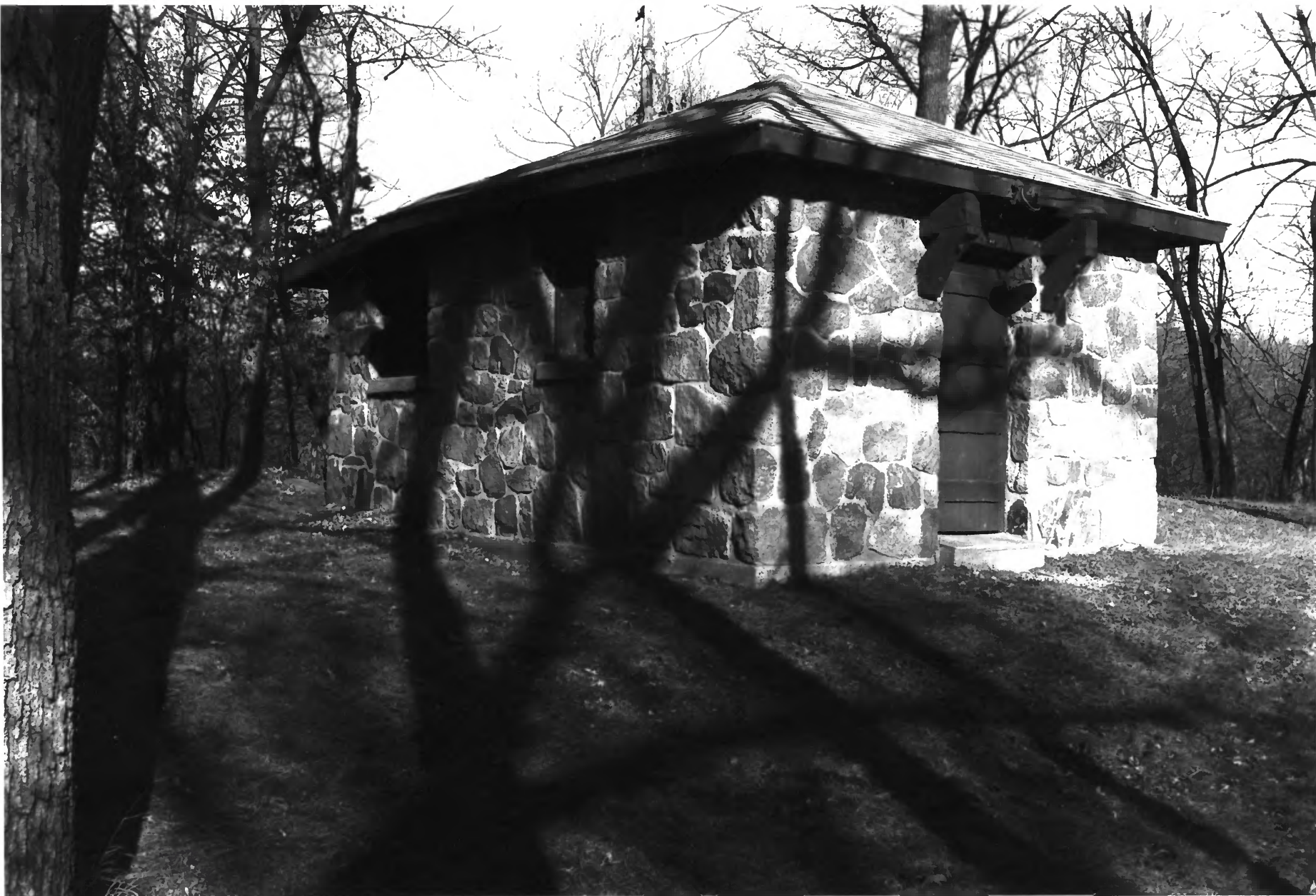
SIBLEY STATE PARK, Pump House KANDIYOHI CO., MN BLDG # 2 PHOTO I.D. 09123 #6
