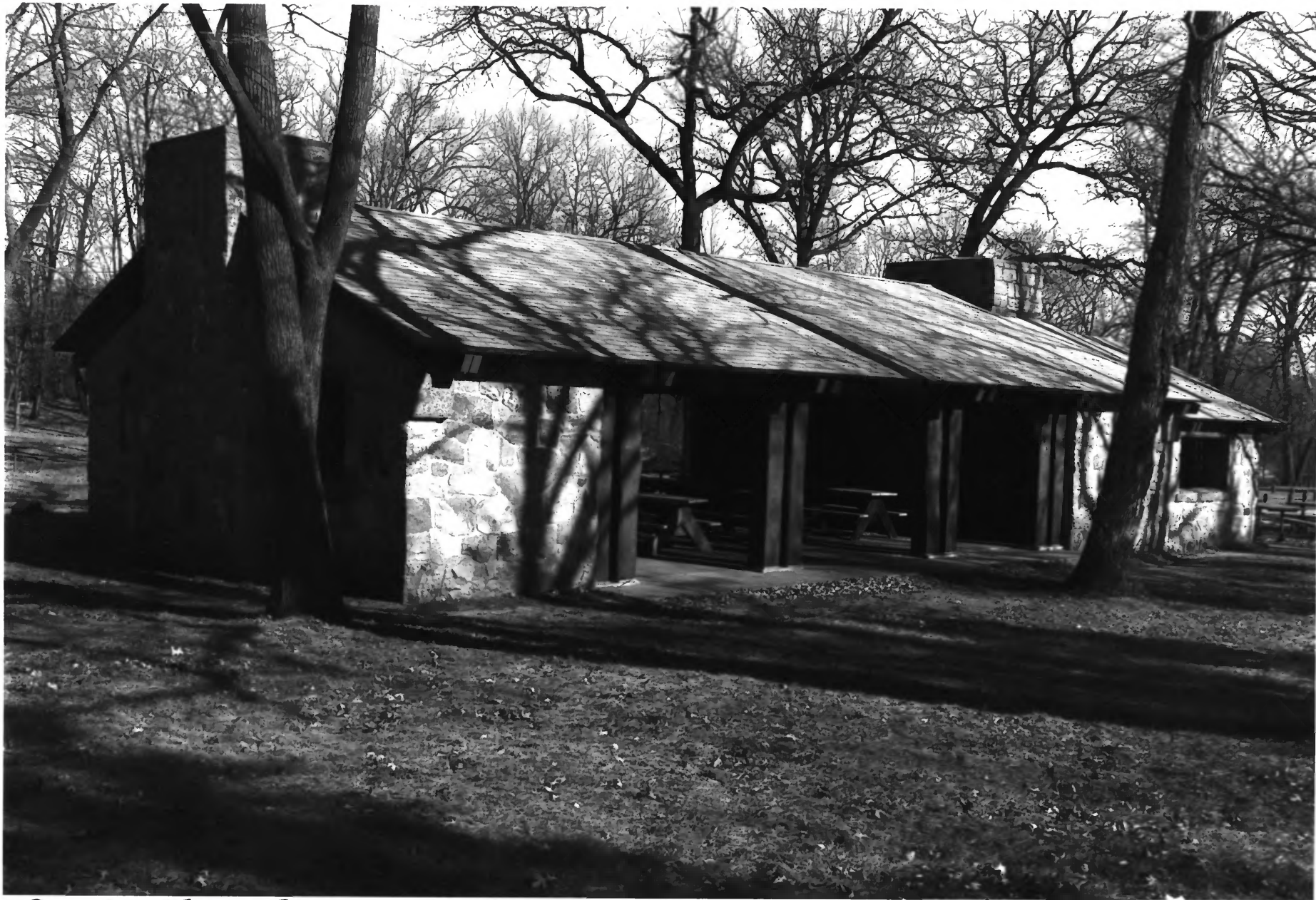
SIBLEY STATE PARK, SHELTER PAVILION KANDIYOHKI CO., MN BLDG #1 PHOTO I.D. 09123#5
