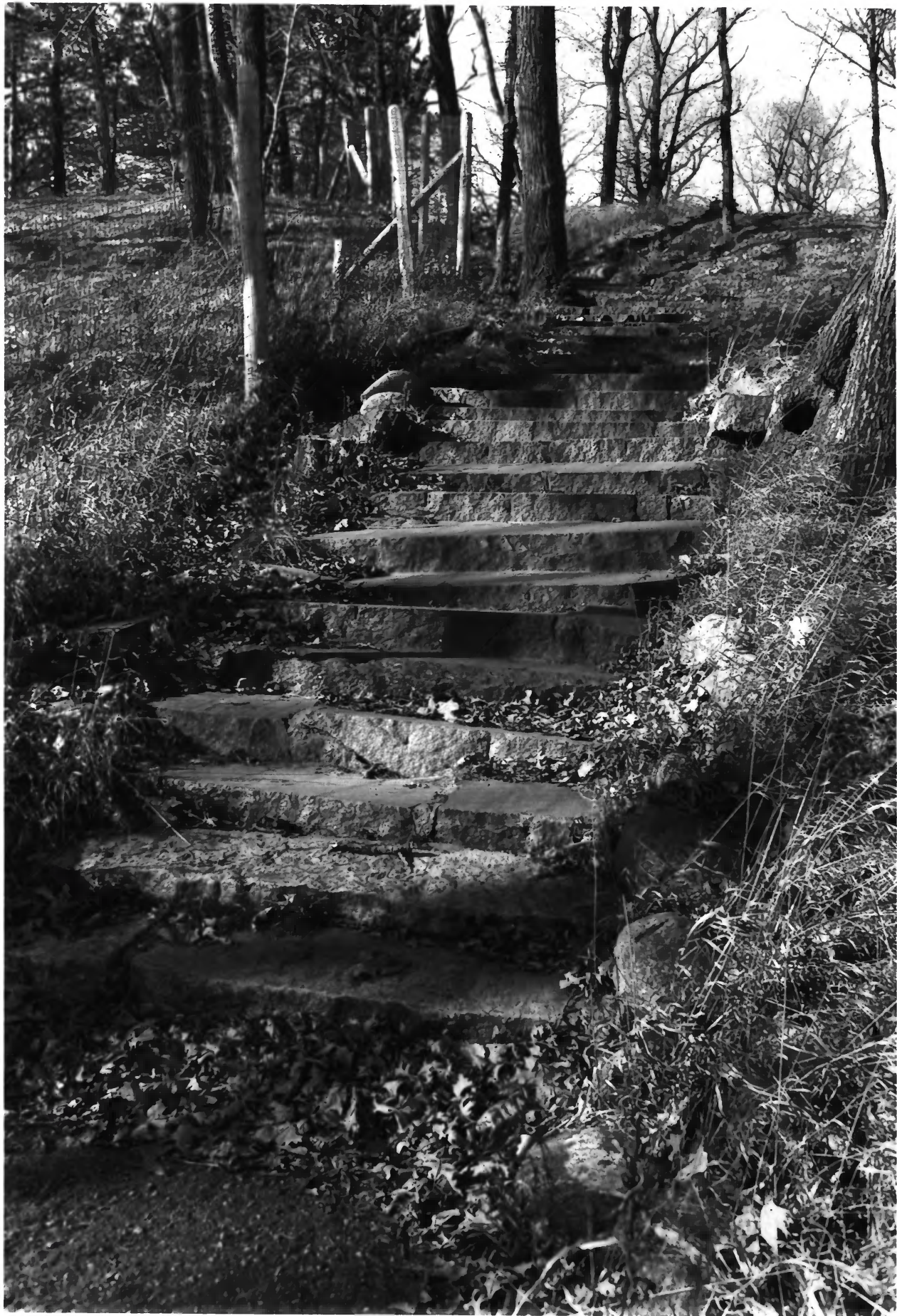
SIBLEY STATE PARK, STONE STEPS KANDIYOHKI CO. MN STRUCTURE # 5 PHOTO I.D. 09123#1
