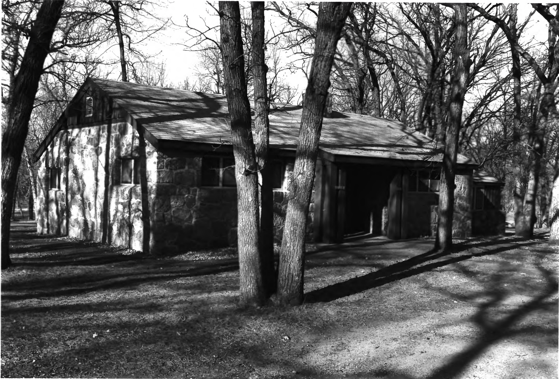
SIBLEY STATE PARK, Combination Building KANDIYOHKI CO., MN BLDG # 10 PHOTO I.D. 09124#21
