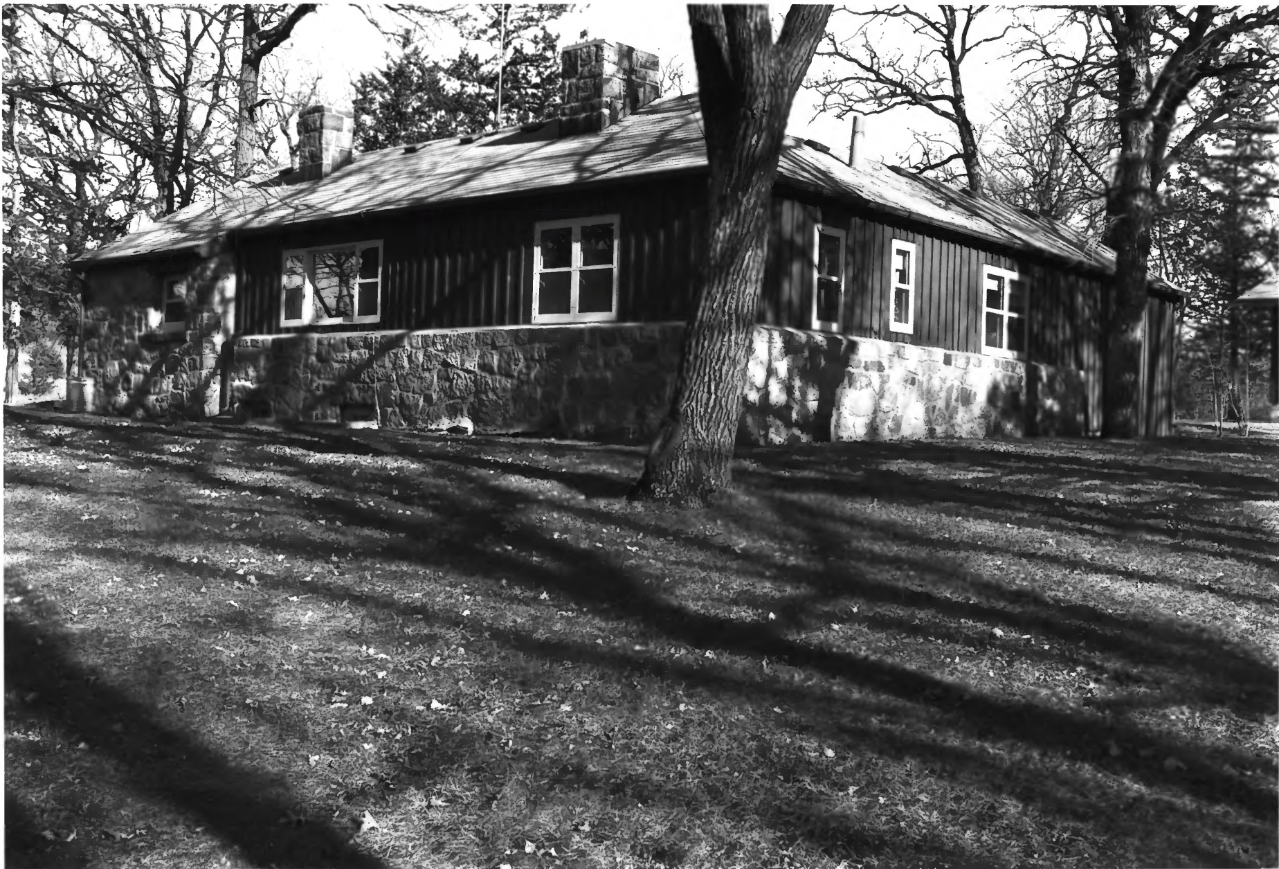
SIBLEY STATE PARK, CUSTODIANS CABIN KANDIYOHI CO., MN BLDG # 12 PHOTO I.D. 09123#12
