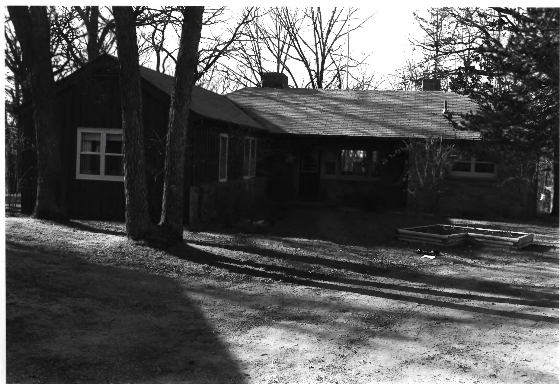
SIBLEY STATE PARK, CUSTODIAN'S CABIN KANDIYOHI CO., MN BLDG # 12 PHOTO I.D. 09123 # 13
