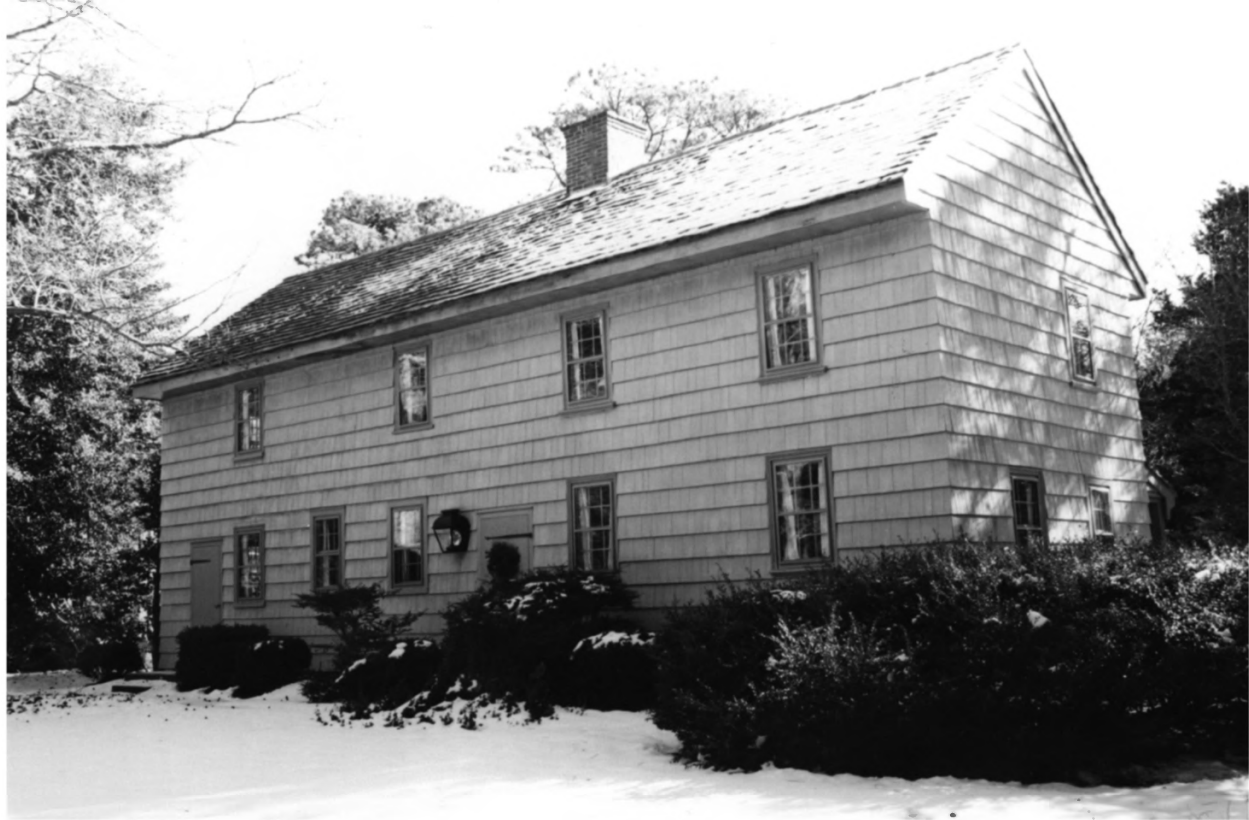
Revere-Iszard-Godfrey House Cape May Co., NJ
