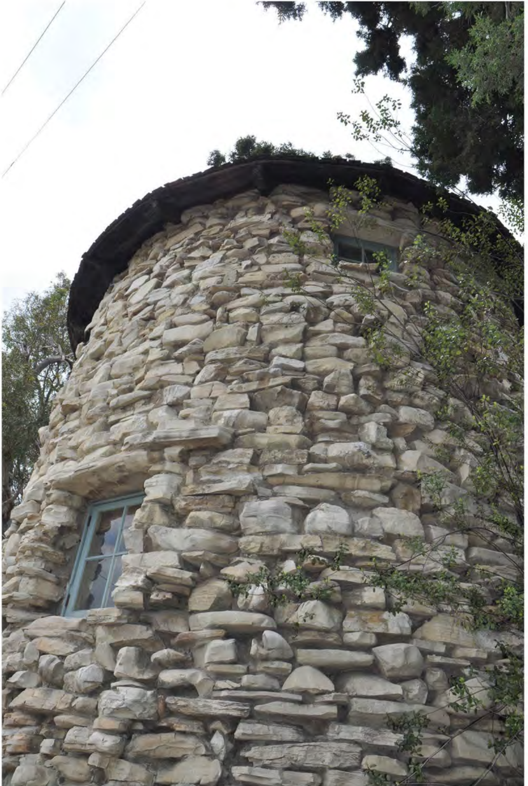
CA_Los Angeles County_Mirlo Gate Lodge Tower_0008
