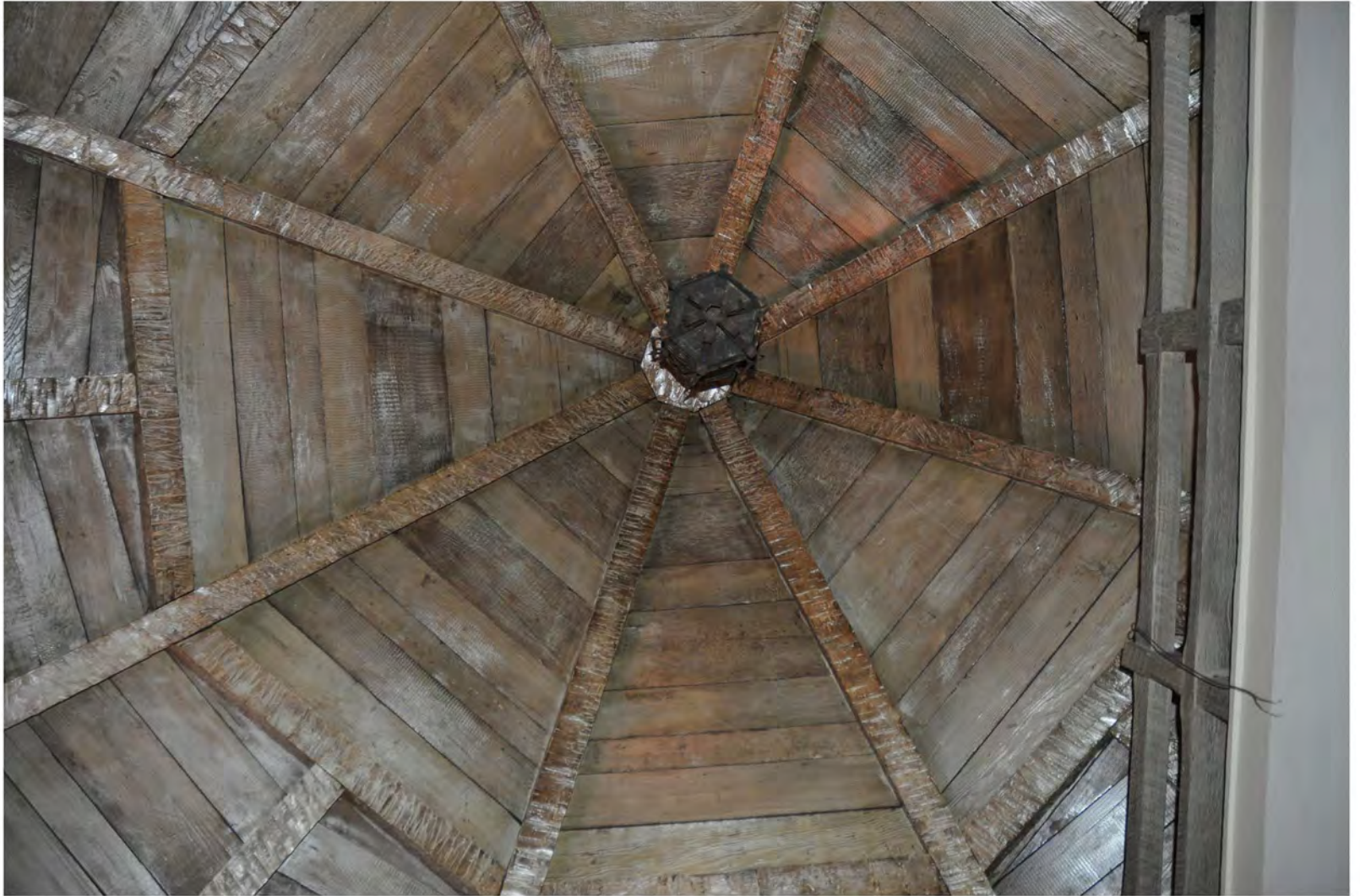
CA_Los Angeles County_Mirlo Gate Lodge Tower_0018
