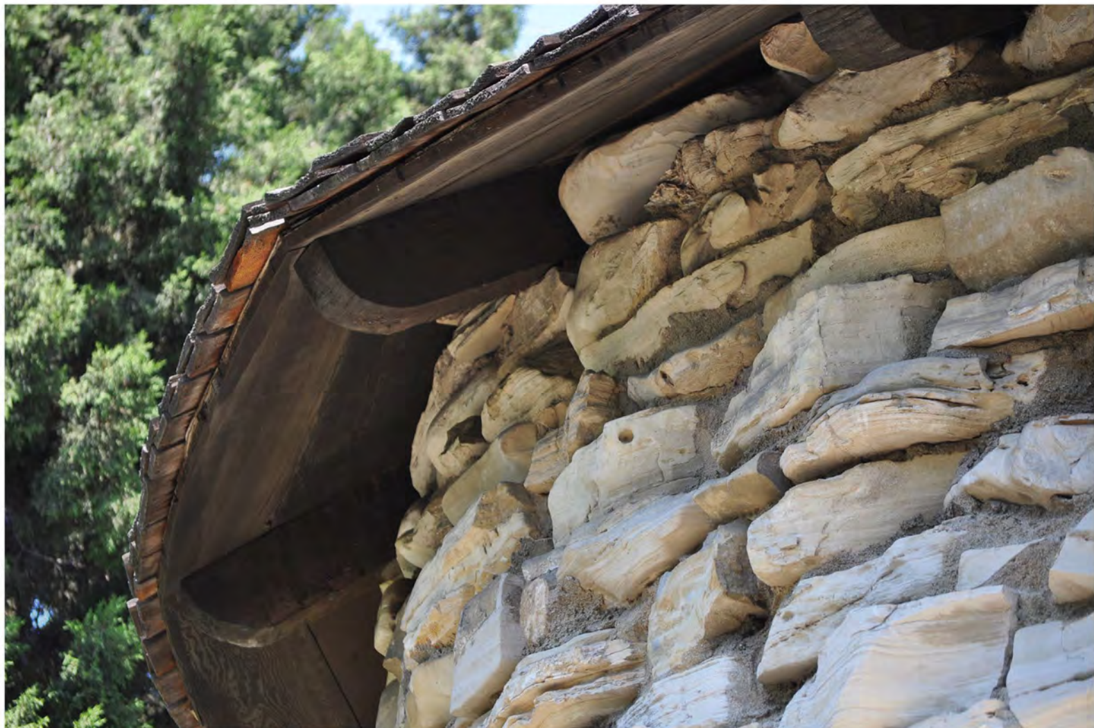
CA_Los Angeles County_Mirlo Gate Lodge Tower_0010
