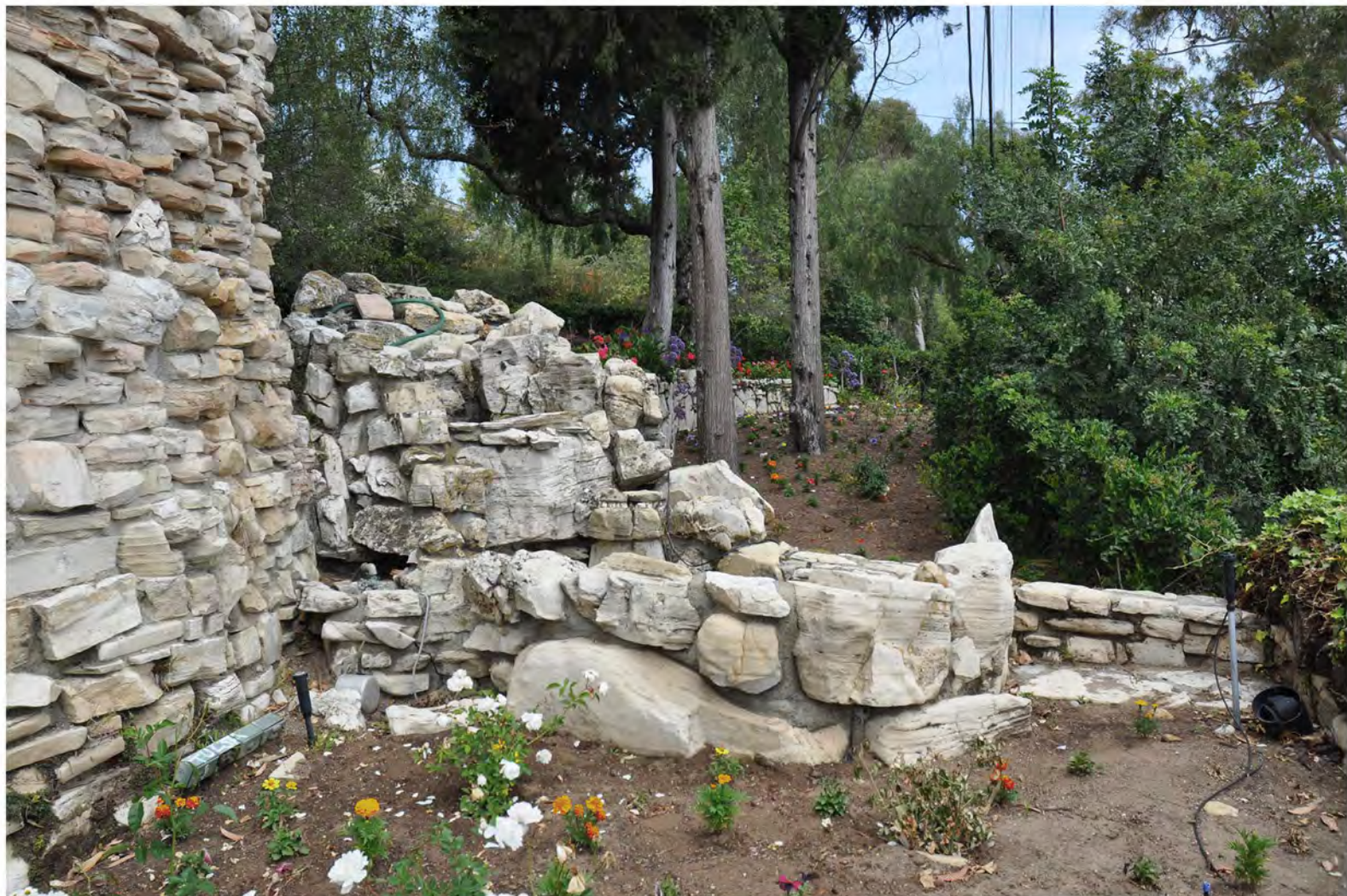
CA_Los Angeles County_Mirlo Gate Lodge Tower_0009
