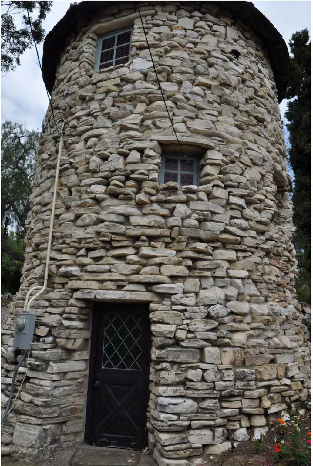
CA_Los Angeles County_Mirlo Gate Lodge Tower_0007
