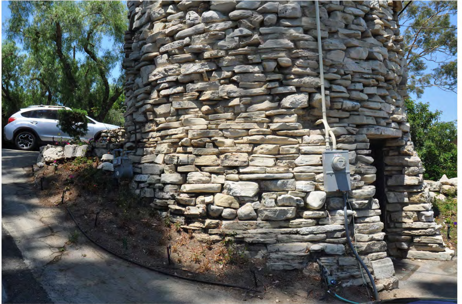
CA_Los Angeles County_Mirlo Gate Lodge Tower_0006
