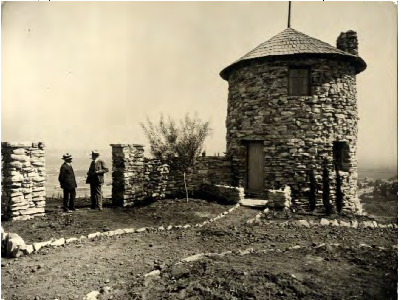
Mirlo Gate Lodge Tower, 1925
