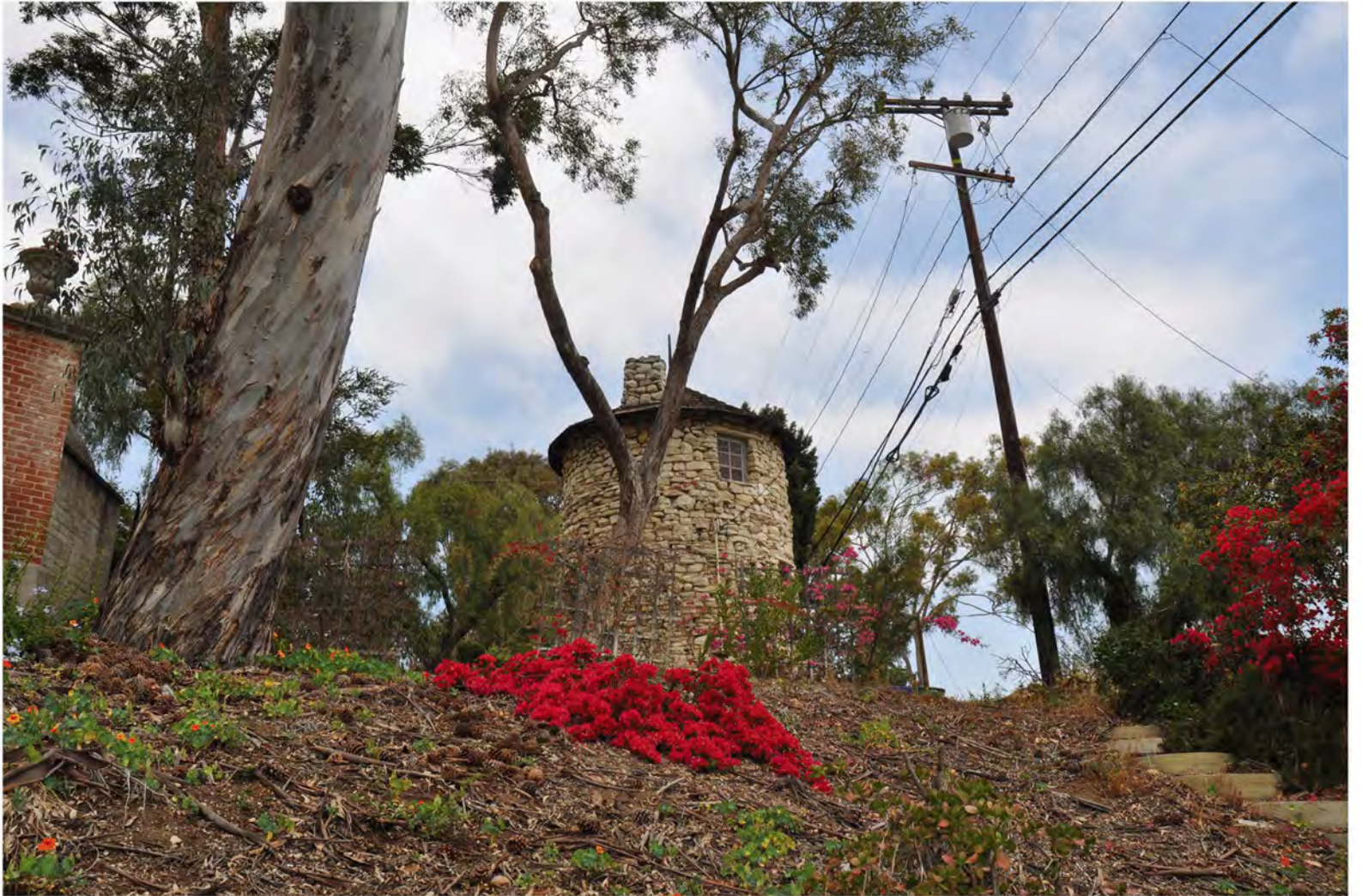
CA_Los Angeles County_Mirlo Gate Lodge Tower_0011
