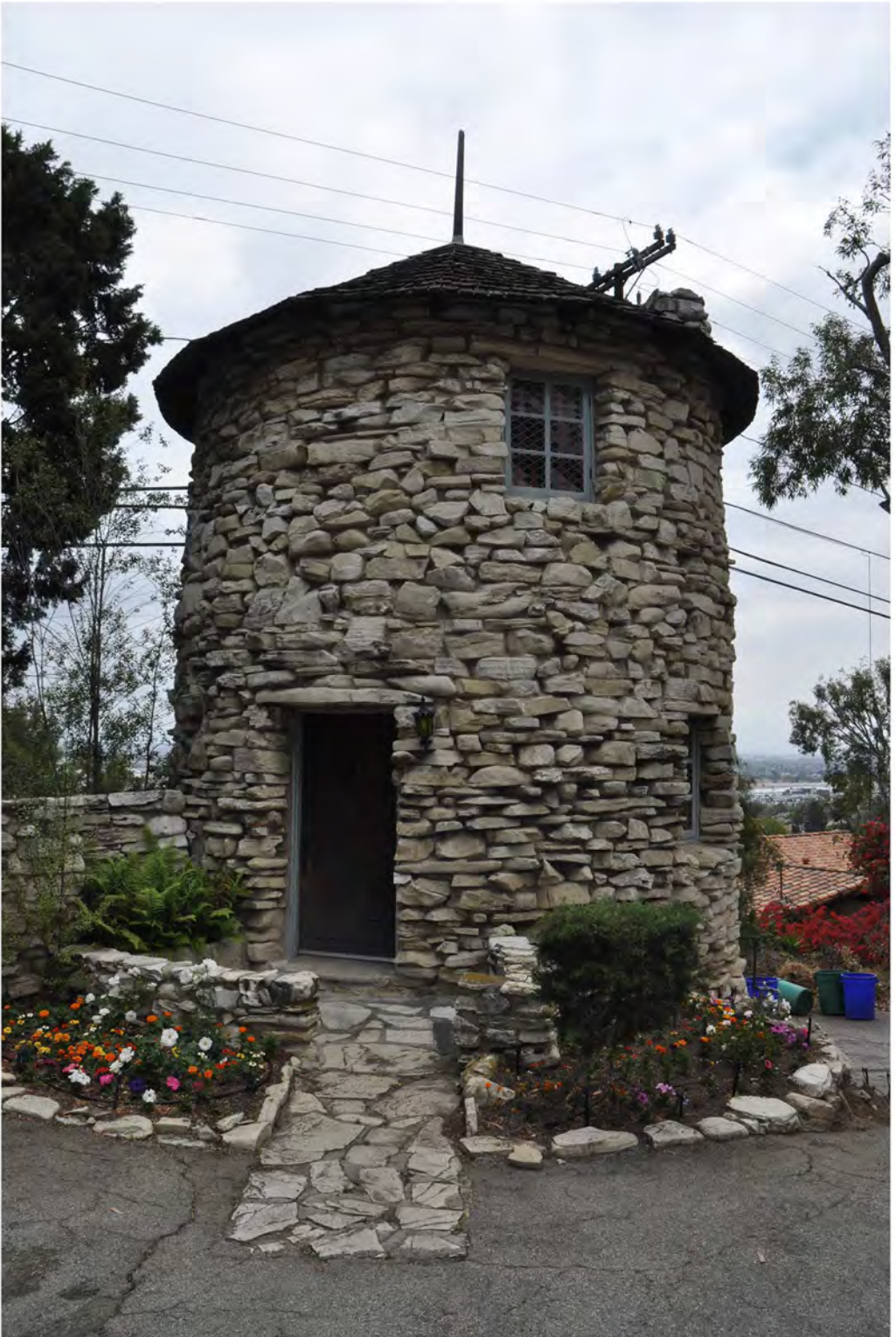
CA_Los Angeles County_Mirlo Gate Lodge Tower_0002
