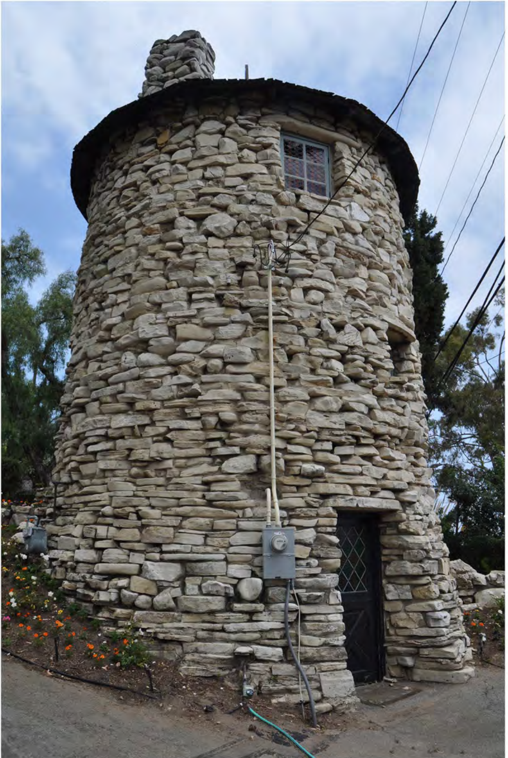
CA_Los Angeles County_Mirlo Gate Lodge Tower_0005
