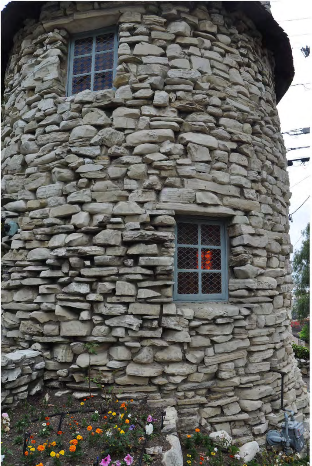
CA_Los Angeles County_Mirlo Gate Lodge Tower_0004
