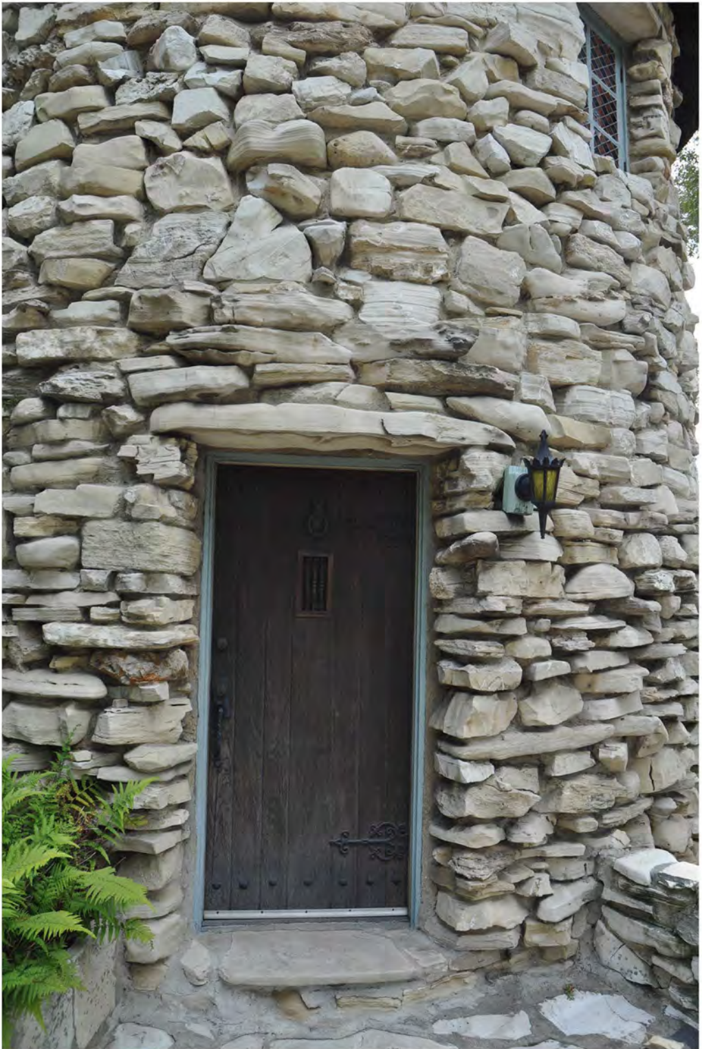
CA_Los Angeles County_Mirlo Gate Lodge Tower_0003
