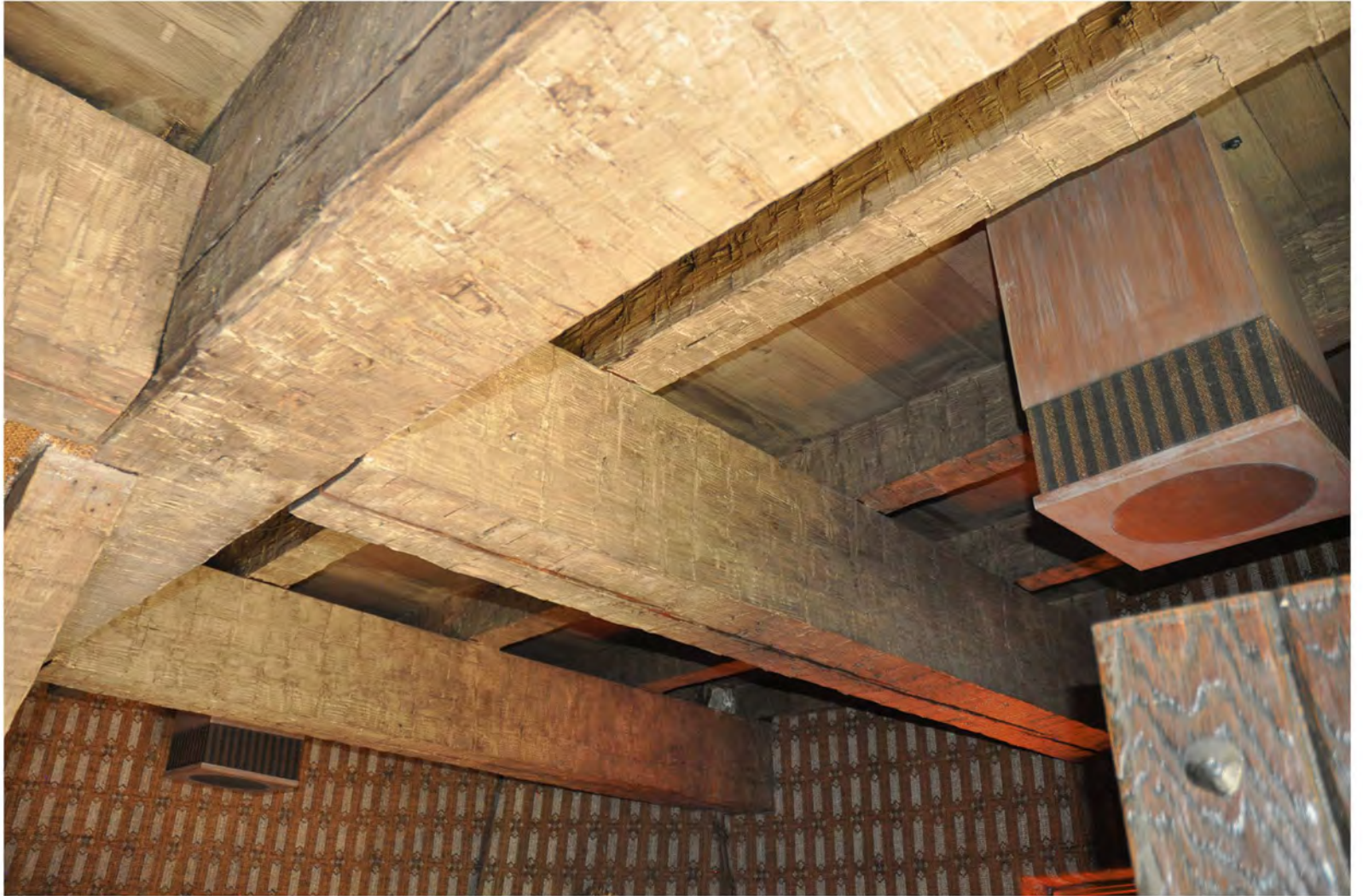
CA_Los Angeles County_Mirlo Gate Lodge Tower_0016
