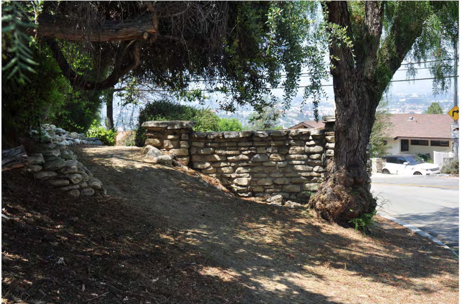
CA_Los Angeles County_Mirlo Gate Lodge Tower_0013
