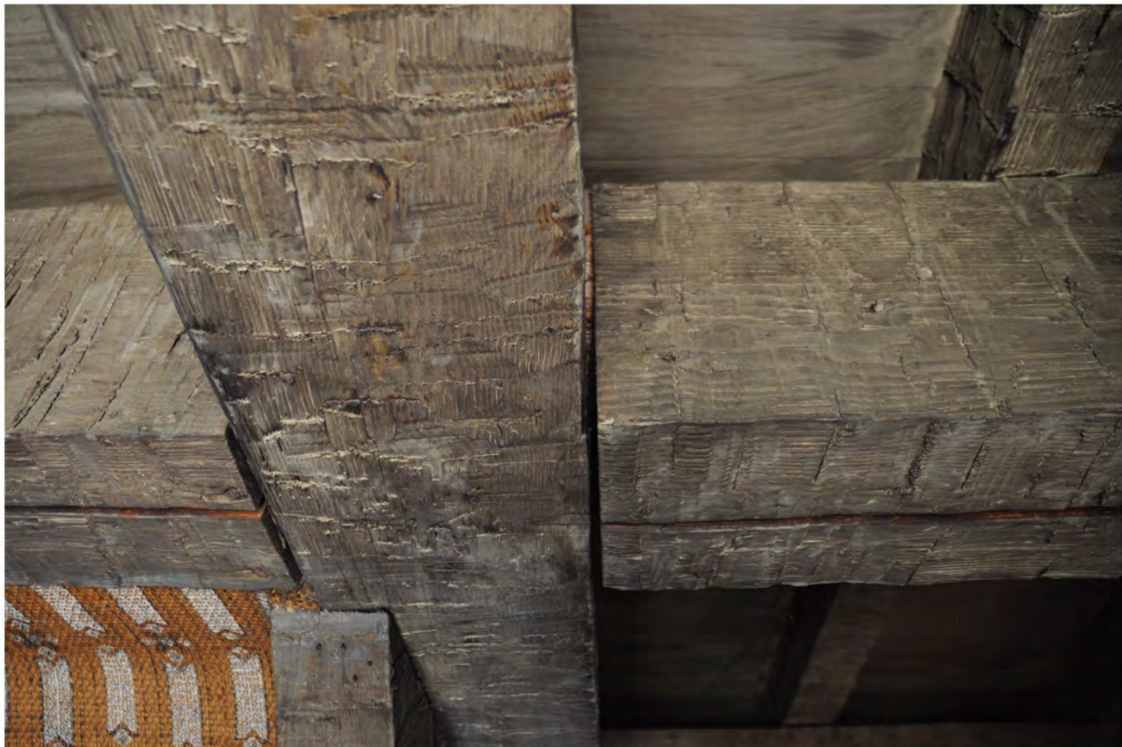
CA_Los Angeles County_Mirlo Gate Lodge Tower_0017
