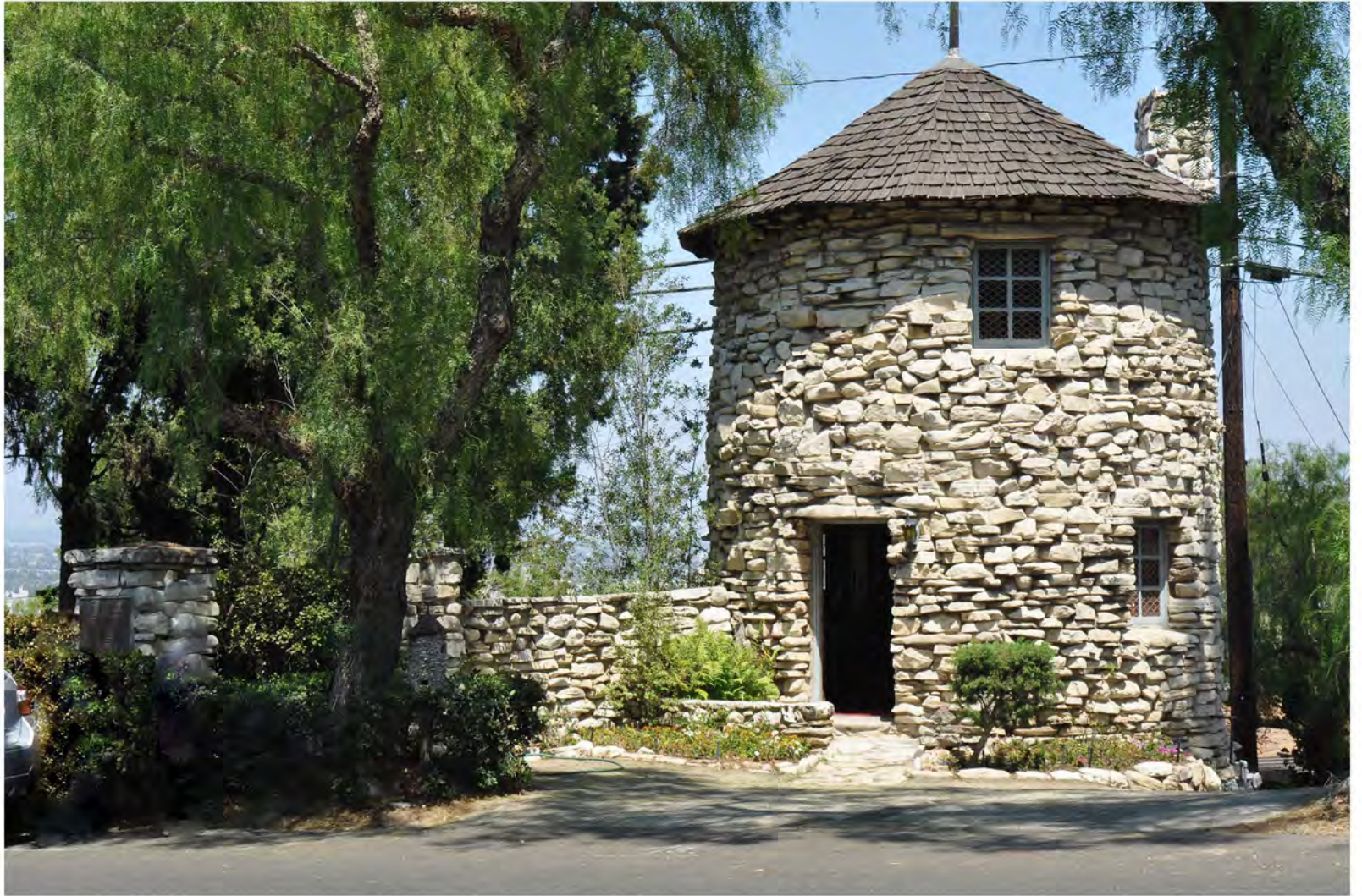
CA_Los Angeles County_Mirlo Gate Lodge Tower_0001
