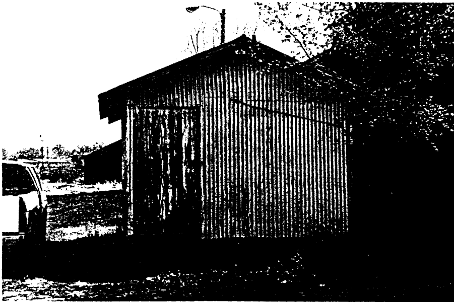
Figure 8. Building 6-1-4. View east.
