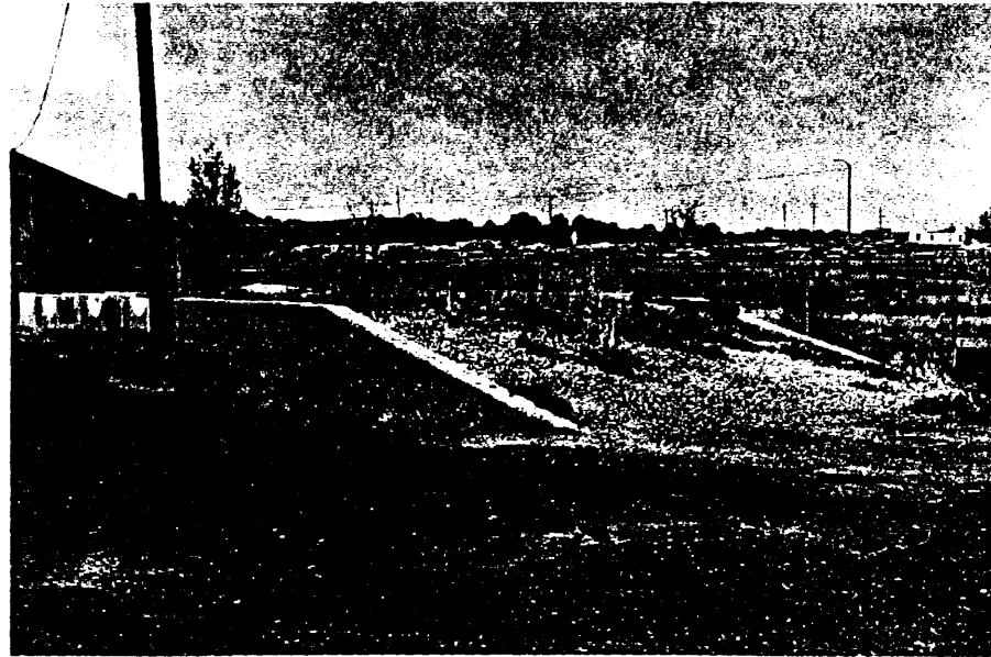
Figure 14. Structure 6-1-D. View northwest.
