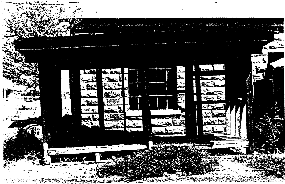
Figure 11. Building 6-1-11. View north.
