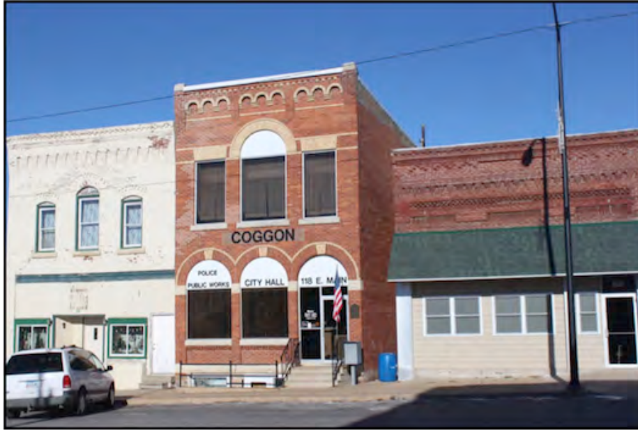
Figure 15. Coggon Bank, 118 East Main Street.
