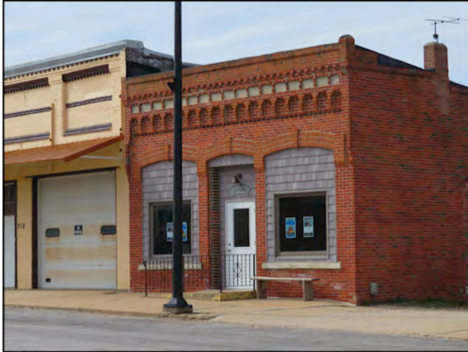
Figure 38. Coggon Monitor Building, 216 East Main Street.
