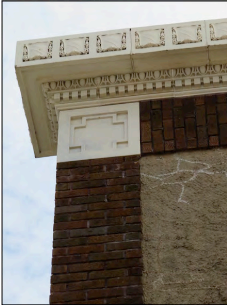
Figure 50. Upper corner detail, Coggon Opera House, 209 East Main Street.
