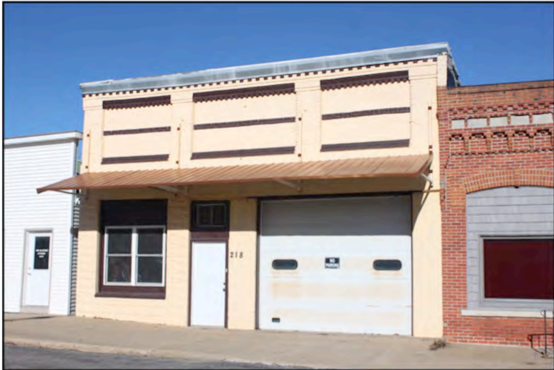
Figure 37. Tom Donnelly Service Station and Garage, 218 East Main Street.
