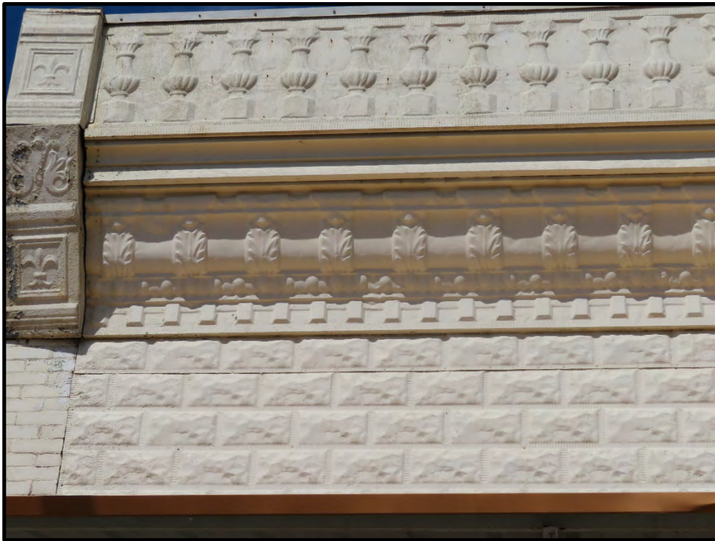
Figure 34. Detail of decorative pressed metal, 202 East Main Street.
