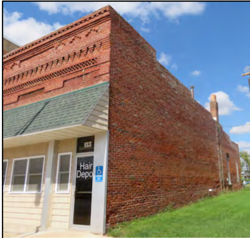
Figure 19. East side of John Campbell Hardware Store, 122 East Main Street.
