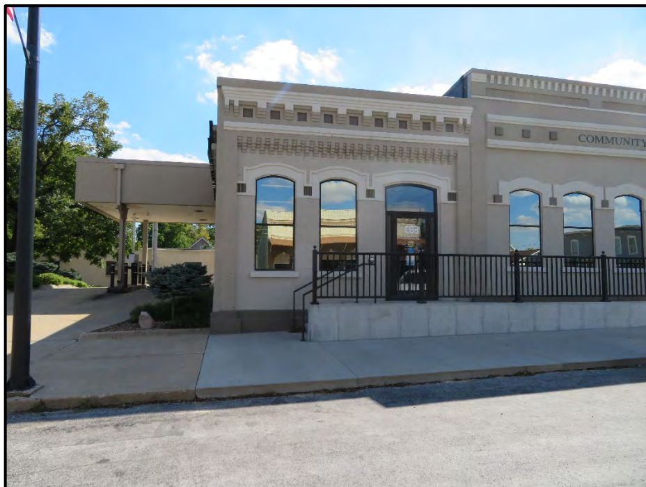
Figure 45. East portion of 201-203 East Main Street, Coggon State Bank/Lindahli Grocery Store.
