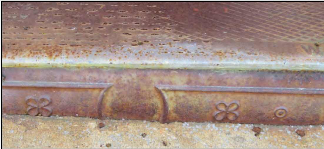
Figure 28. Metal step detail, 123 East Main Street.
