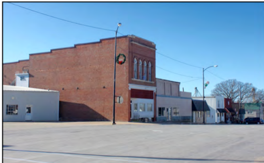
Figure 23. Overview of East Main Street, 100 block, south side.
