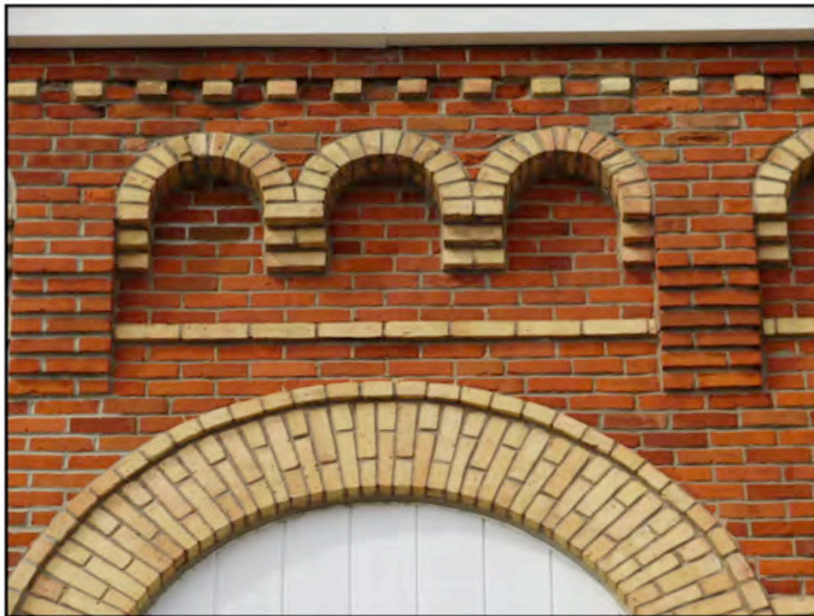
Figure 16. Detail of brickwork, 118 East Main Street.
