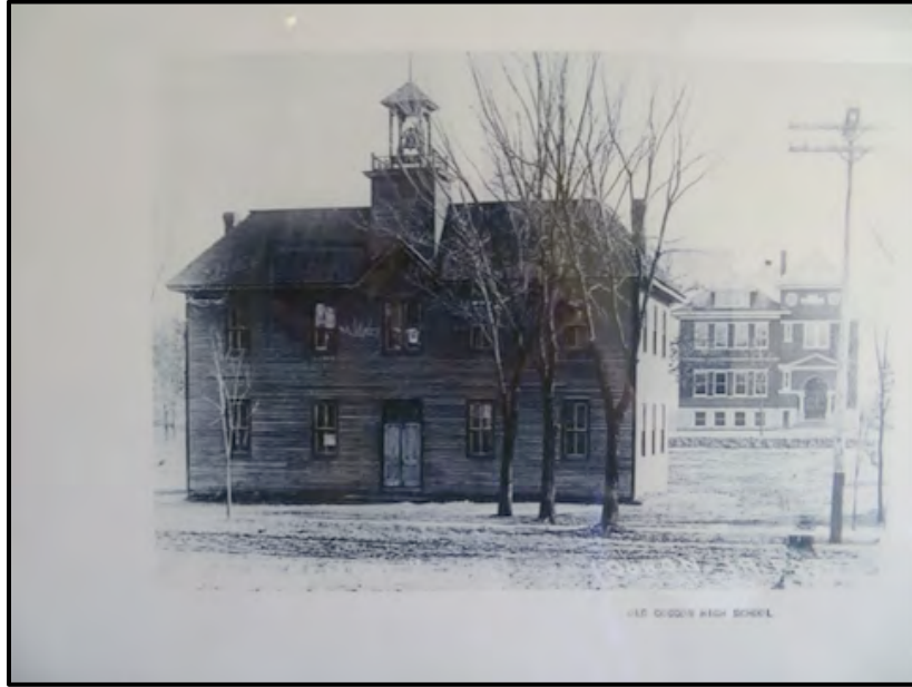
Figure 8. Circa 1909 photograph showing 1890 school building with the 1909 Coggon Public School Building under construction in the background. Source: Coggon Historical Society.
