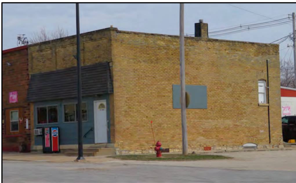
Figure 25. Winfield Scott Barber Shop, 101 East Main Street.
