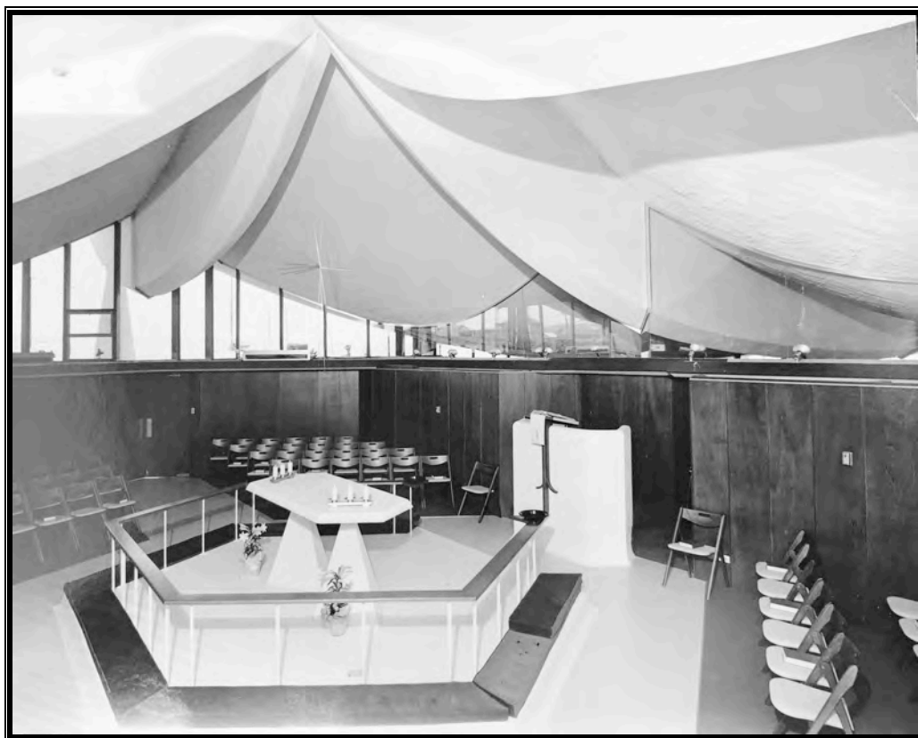
HP-8: Sanctuary Interior, Circa 1964-1965 (Courtesy of Joel Haertling)
