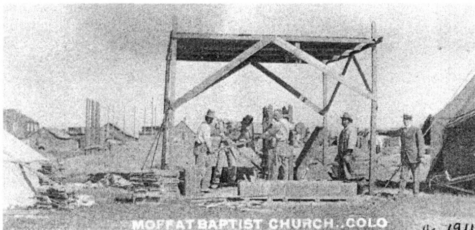
This circa 1911 photograph shows a four-man crew using a concrete block press for the Moffat church. Source: Jones, Historic Structure Assessment, 2003.
