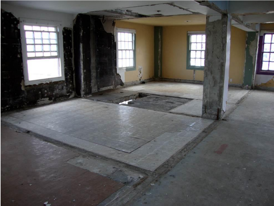
24 Typical floor plate showing evidence of room divisions and original wall finishes and trim.
