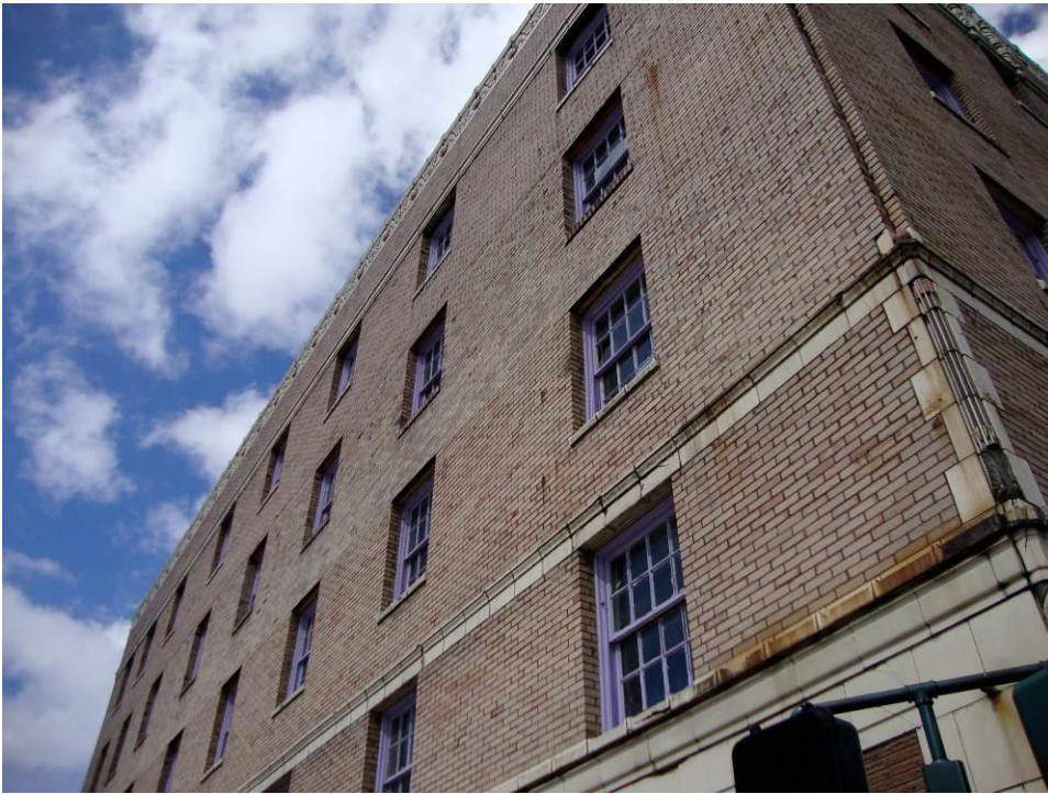
6 Detail of southeast corner showing brick and terra cotta.
