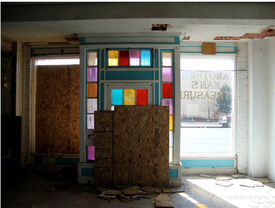
17 Interior view of original W Heron St. storefront.
