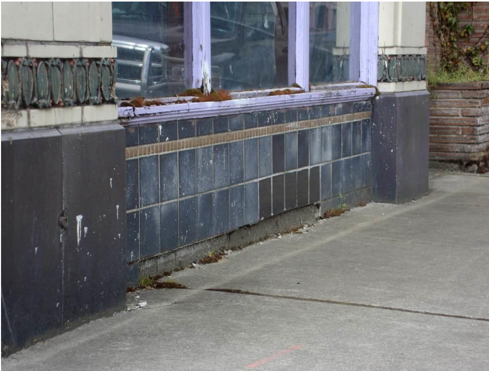
12 Detail of storefront bulkhead.
