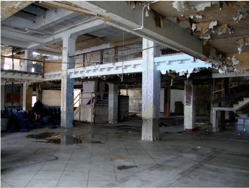
14 Main lobby space showing skylight.
