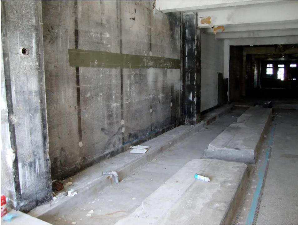
20 Former soda fountain area showing counter layout area and terrazzo floor.
