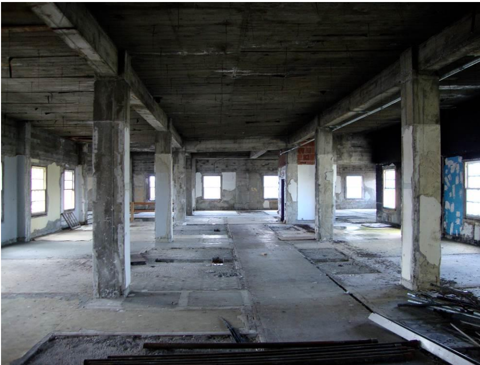
25 Typical floor plate showing evidence of hallway and room divisions.
