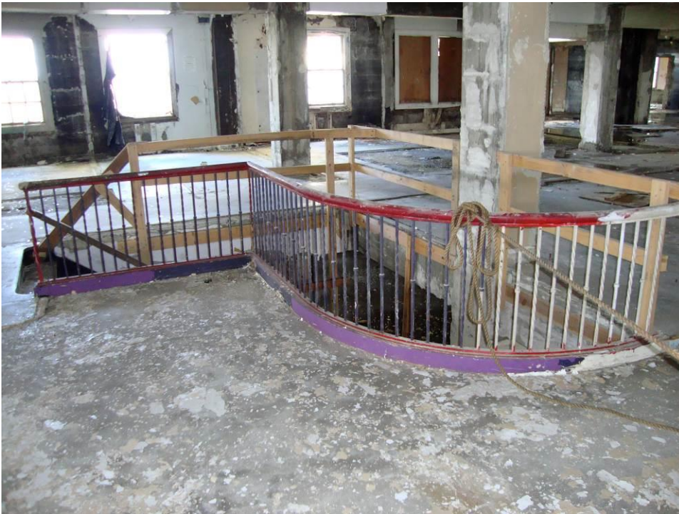
26 Detail of mezzanine level stairwell railing.
