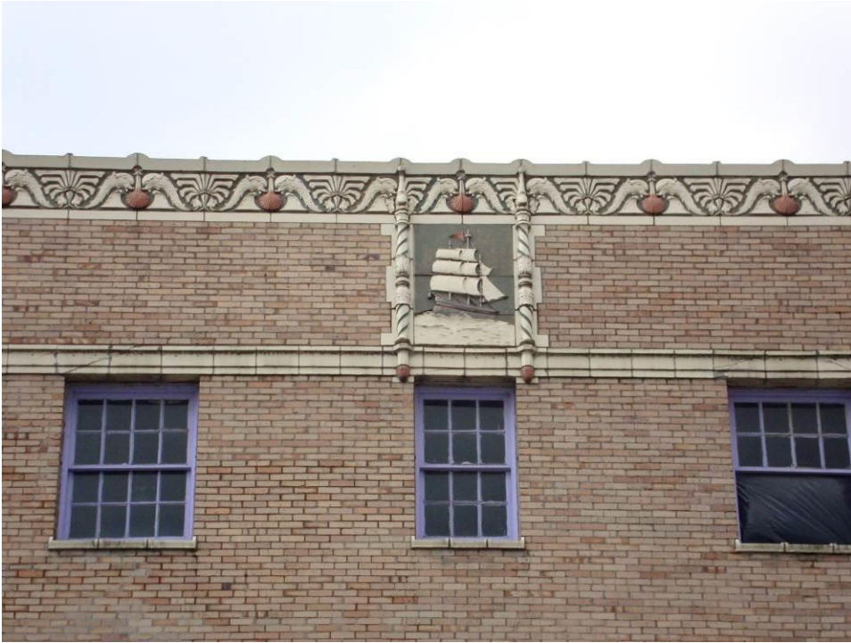
10 Decorative cornice detail above skylight on main façade.
