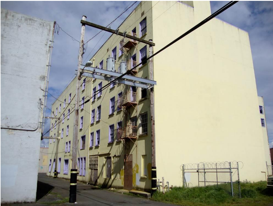
4 Northwest corner showing rear wing; camera facing southwest
