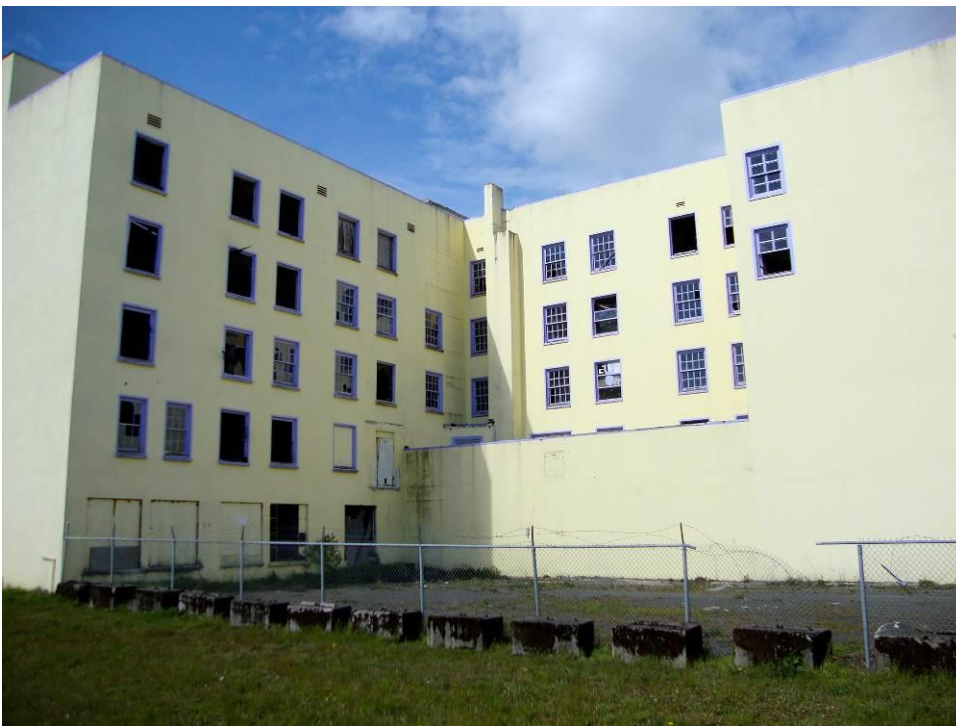
5 Rear façade; camera facing west.
