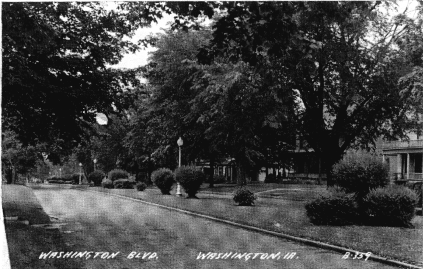
Figure 27. Historic view of the 500 block of W. Washington Blvd in the 1930s, depicting the brick street with boulevard, growing shrubs, and historic light fixtures (Washington County Historical Society).
