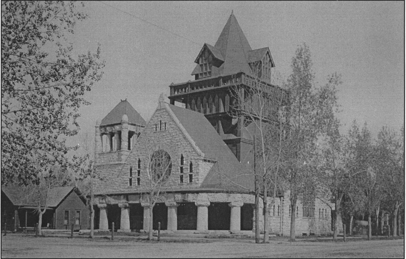
Figure 5. This undated, circa 1890s, view (northwest) shows the church with its ornate lantern-tower. SOURCE: Hook Photo, First Congregational Church archives.
