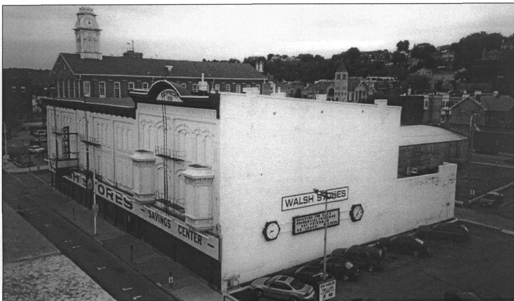
Figure 19: Both buildings, view to the southwest
