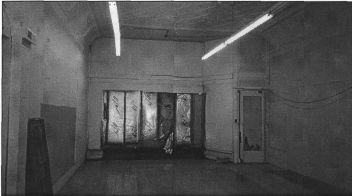
Figure 7: metal ceiling and cove molding, southern half of plan, view north
