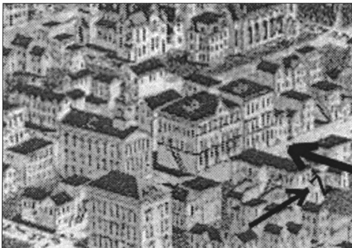
Figure 25: Wellge, Perspective Map of Dubuque, 1889 The arrow points to the new Ziepprecht Block.
