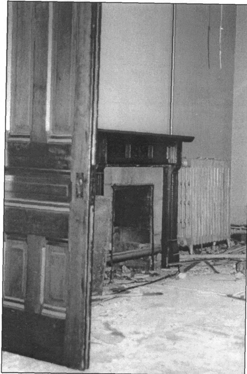
Figure 11: Working fireplace and sliding door, second floor, view northeast
