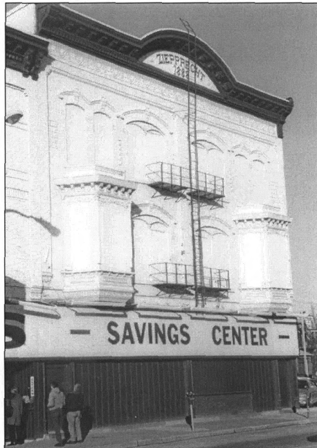
Figure 1: Ziepprecht Block, 1888, view northwest
