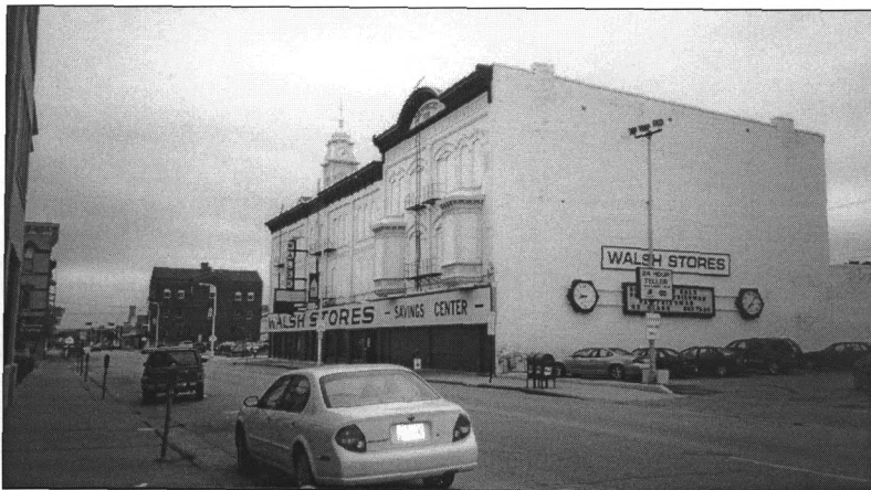
Figure 20: Ziepprecht and German Trust buildings, view to southwest
