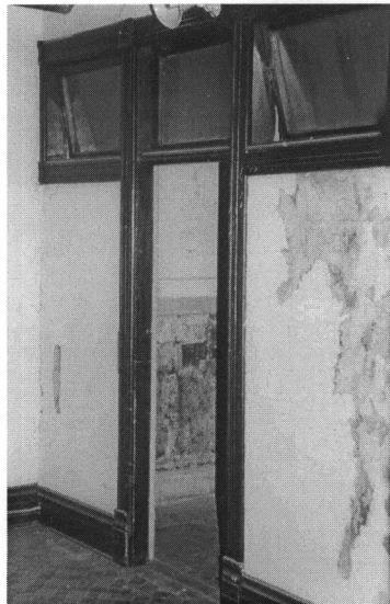
Figure 15: Door with transom lights, third floor, southwest corner of north apartment, view southwest (Photo by J. Jacobsen)
