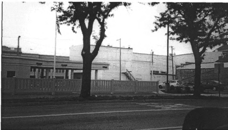
Figure 21: general rear view of building, viewed to southeast.
