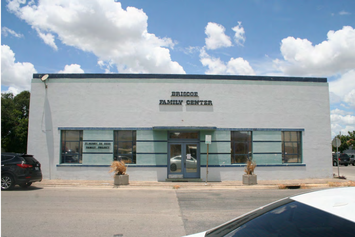
Photo 18: 114 E. Nopal St. (#5), looking north.
