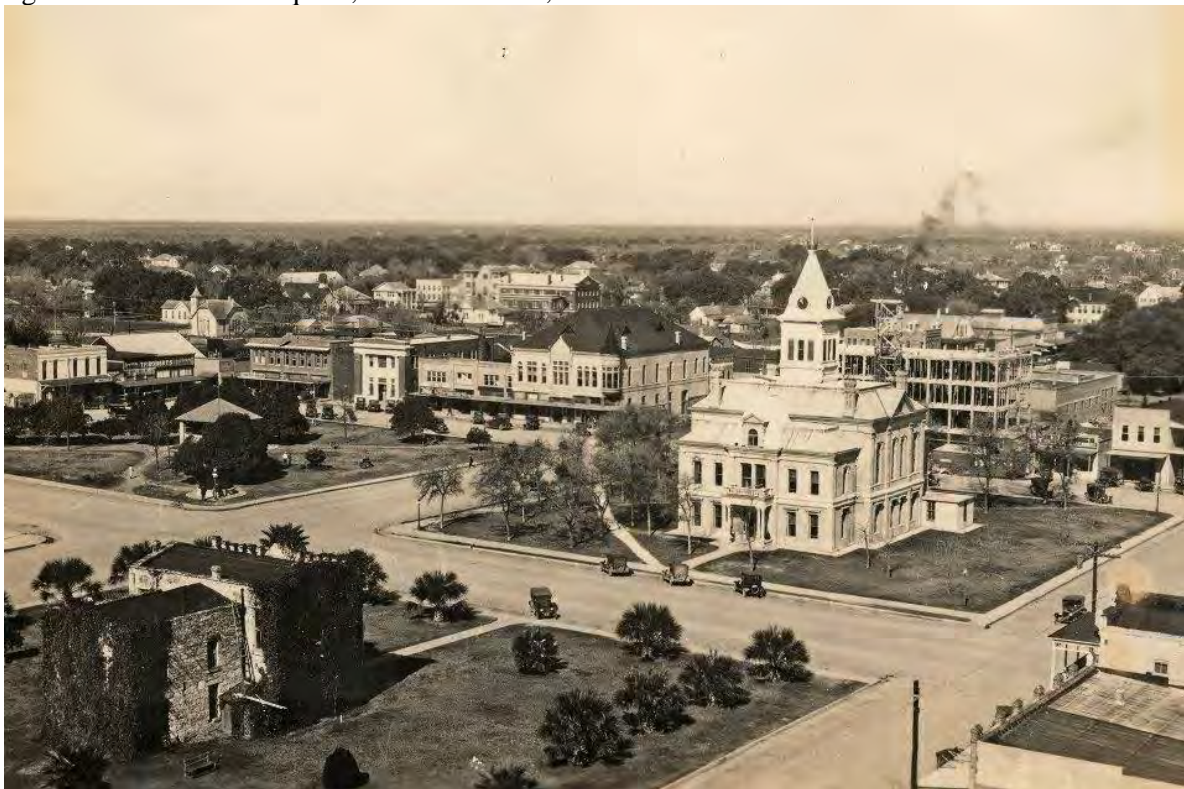
Figure 11: Courthouse Square, view northwest, c.1927.
