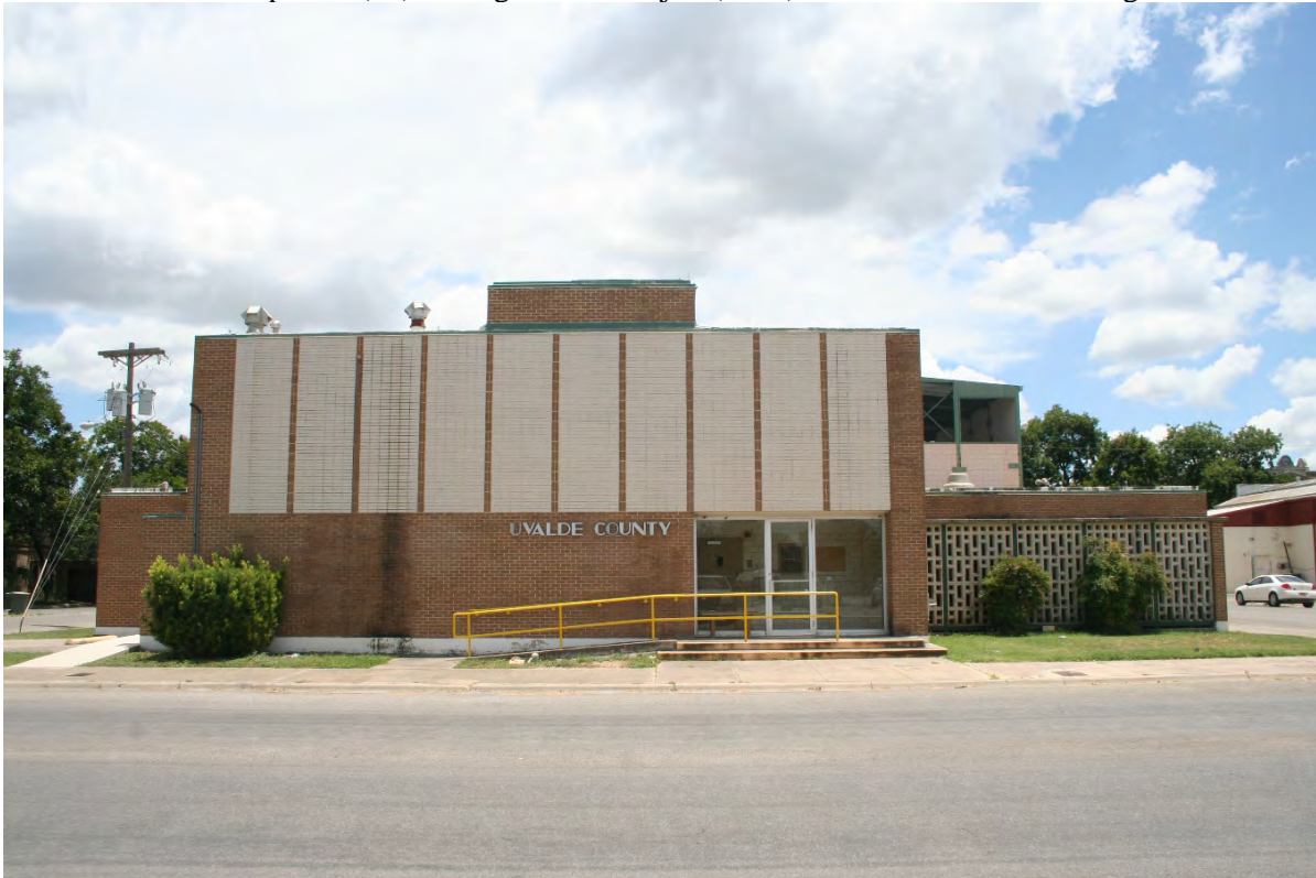
Photo 16: 121 E. Nopal St. (#7), facing south. The jail (1968) is the newest contributing resource in the district.
