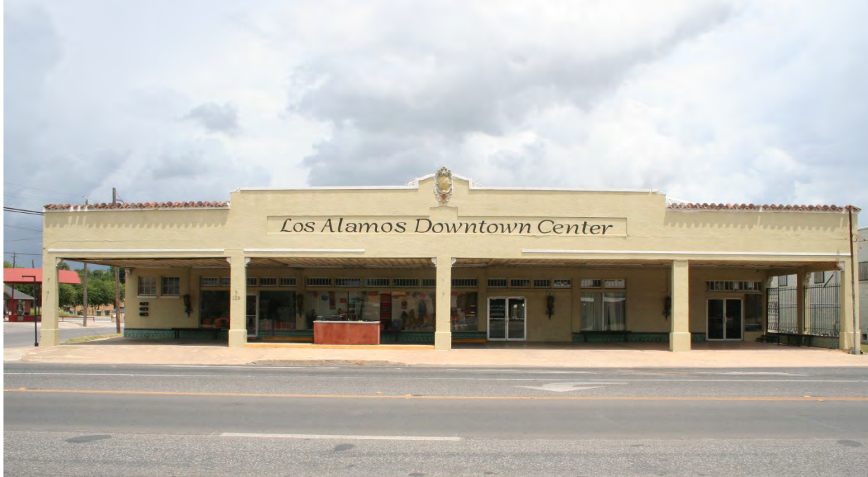
Photo 9: 128 W. Main St. (#78), facing north.
