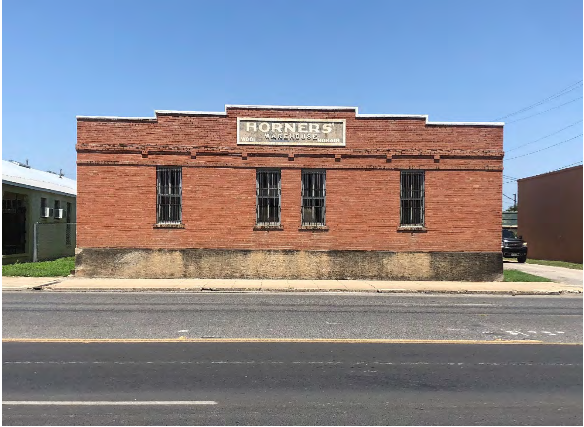
Photo 11: 120 W. Main St. (#77), facing north.
