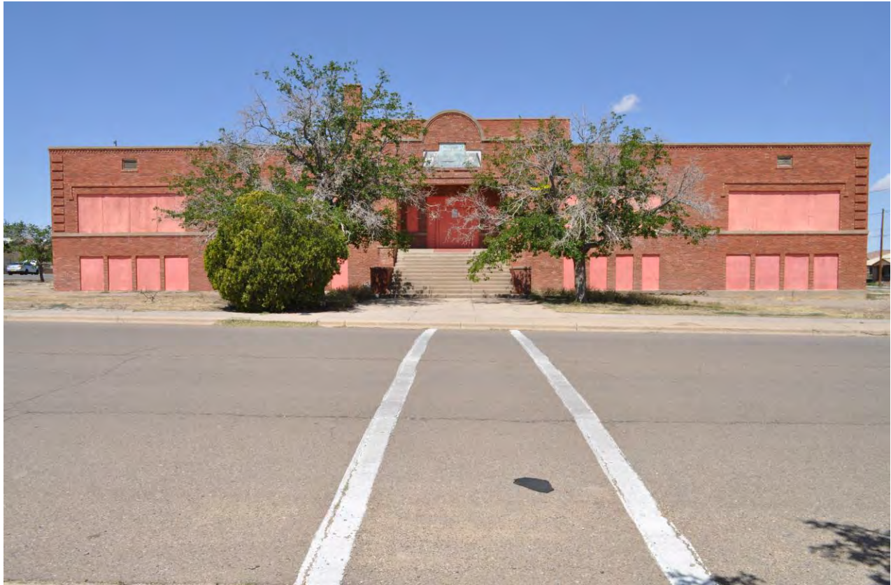
1 of 8. Main façade, photographer facing east
