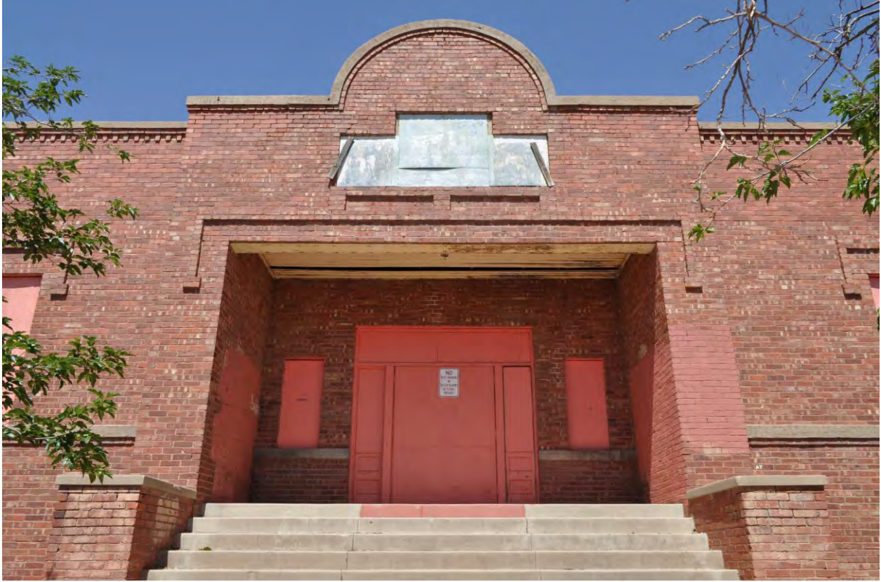
2 of 8. Main entrance, detail, photographer facing northwest.
