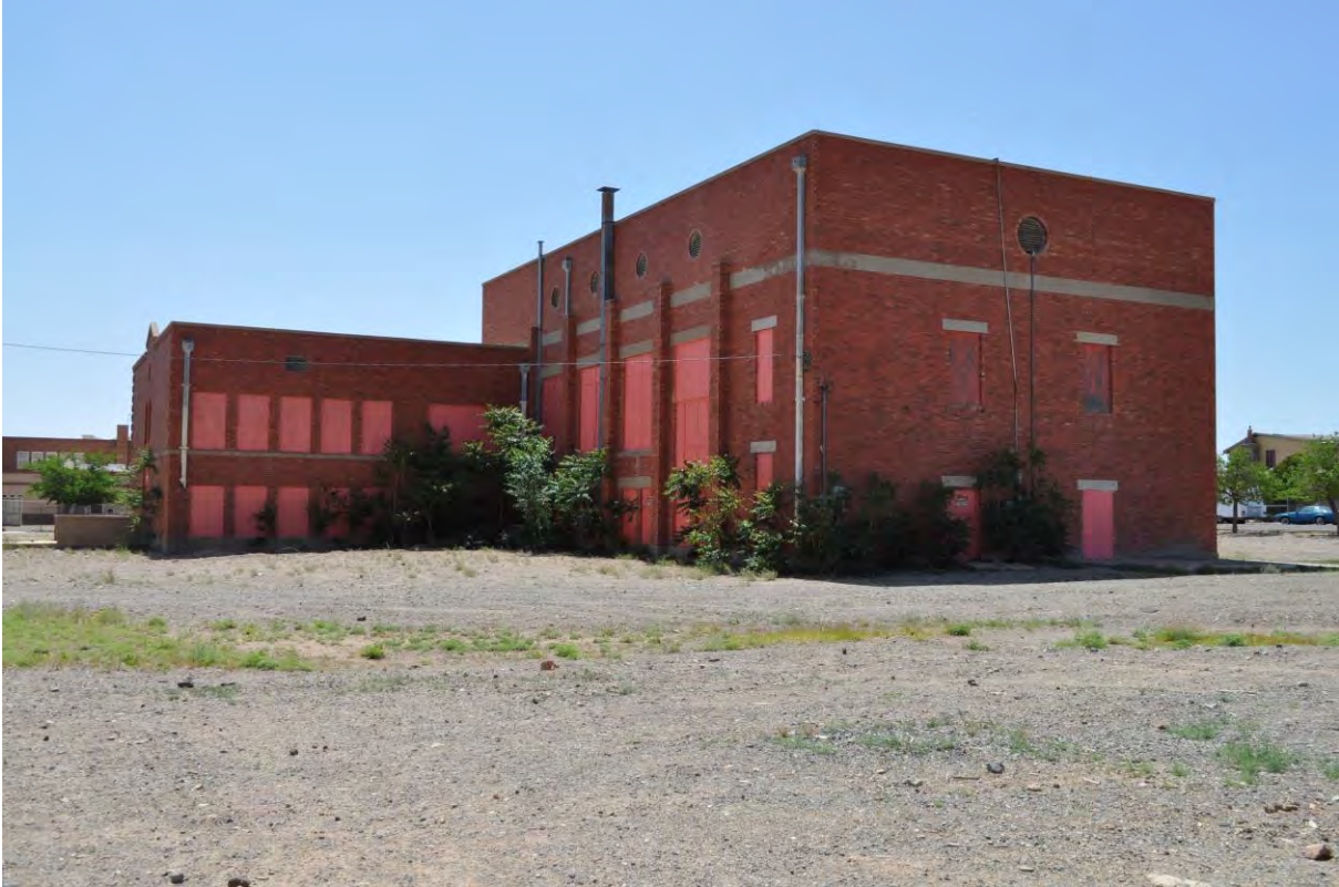
5 of 8. South side and rear addition, photographer facing northeast.
