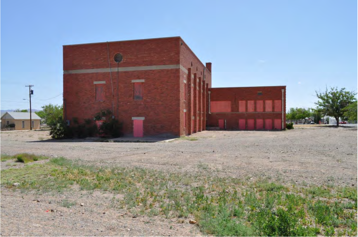
4 of 8. North side and rear addition, photographer facing south.
