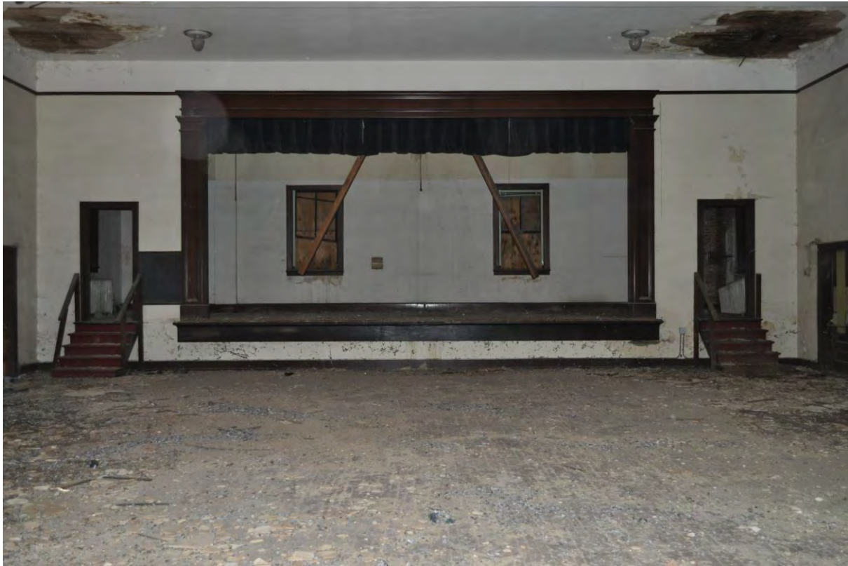
7 of 8. Interior, auditorium, photographer facing east.
