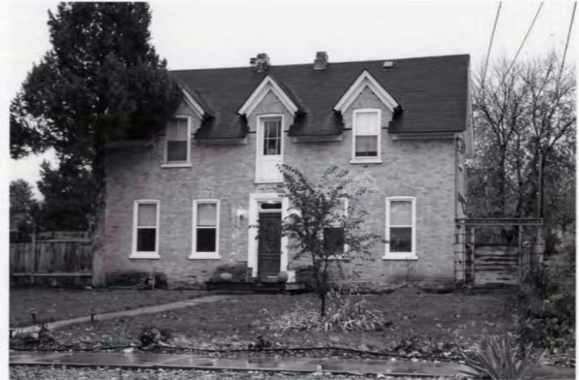
52 N. 100 West Photograph 14
