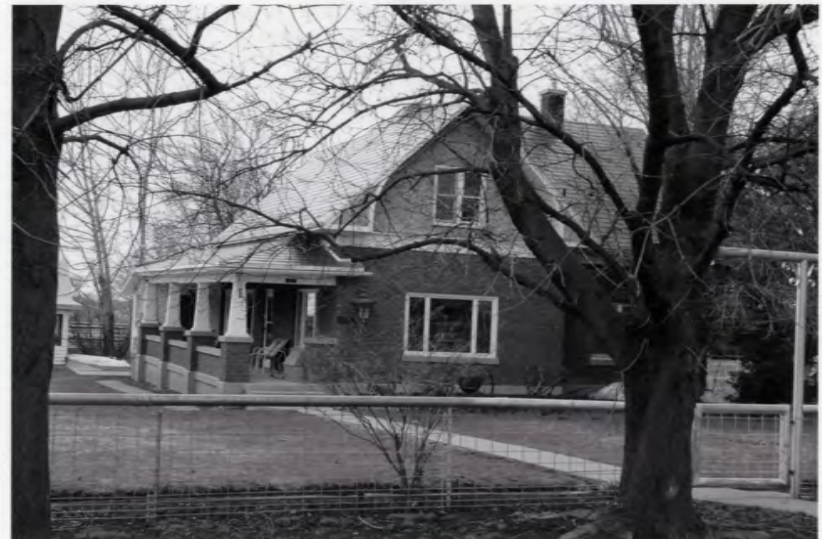
87 S. 200 West Photograph 32
