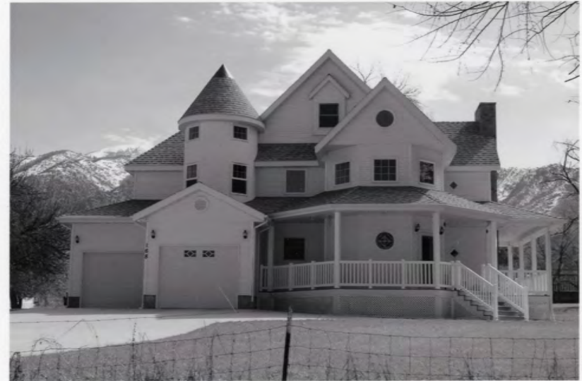
168 S. 200 West Photograph 58
