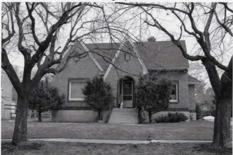
48 N. 100 West Photograph 47
