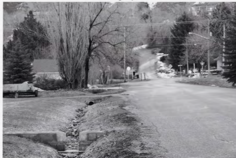
Irrigation ditch at 50 West and 500 South Photograph 8
