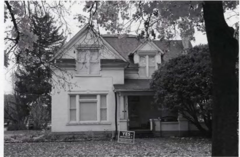
95 S. 100 West Photograph 22
