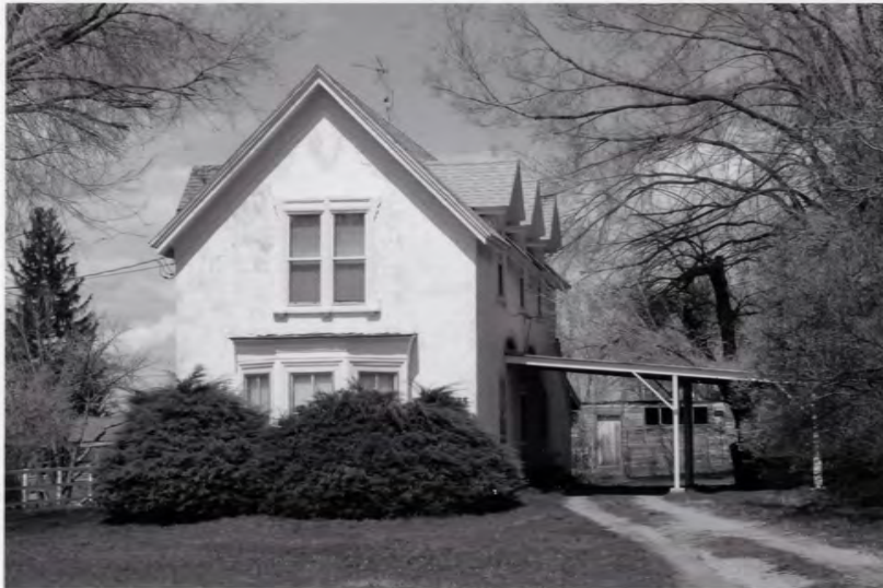
55 E. 100 South Photograph 15
