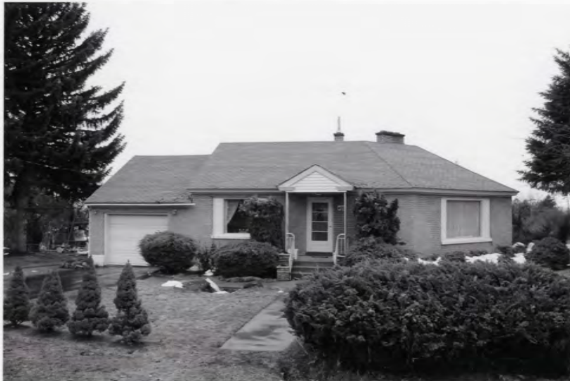
407 S. 100 West Photograph 53
