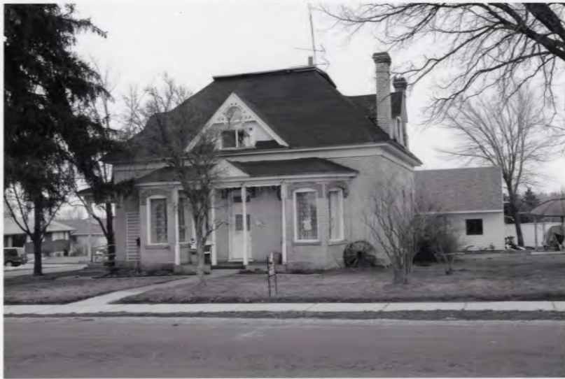
105 E. 200 North Photograph 27
