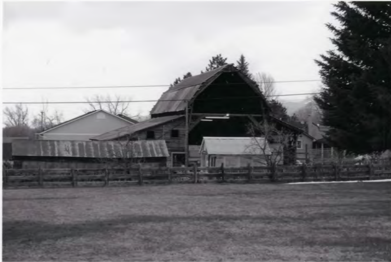
456 S. 100 West (rear) Photograph 21
