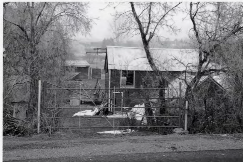
12 N. 300 East (rear) Photograph 44
