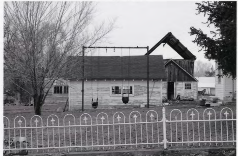
153 E. Center Street (rear) Photograph 24
