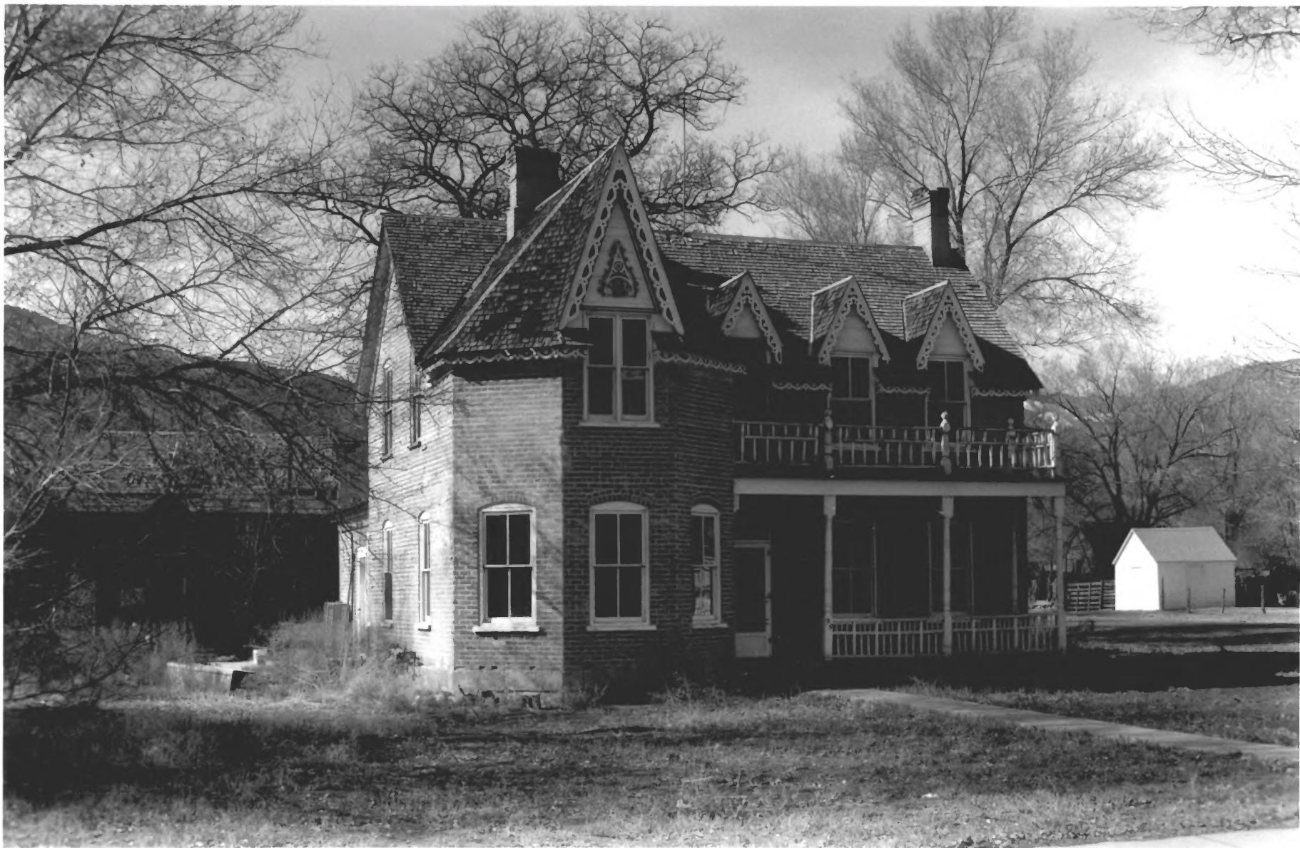
MORRILL, JOHN AND ELLA, HOUSE JUNCTION, PIUTE CO., UTAH PHOTO#1
