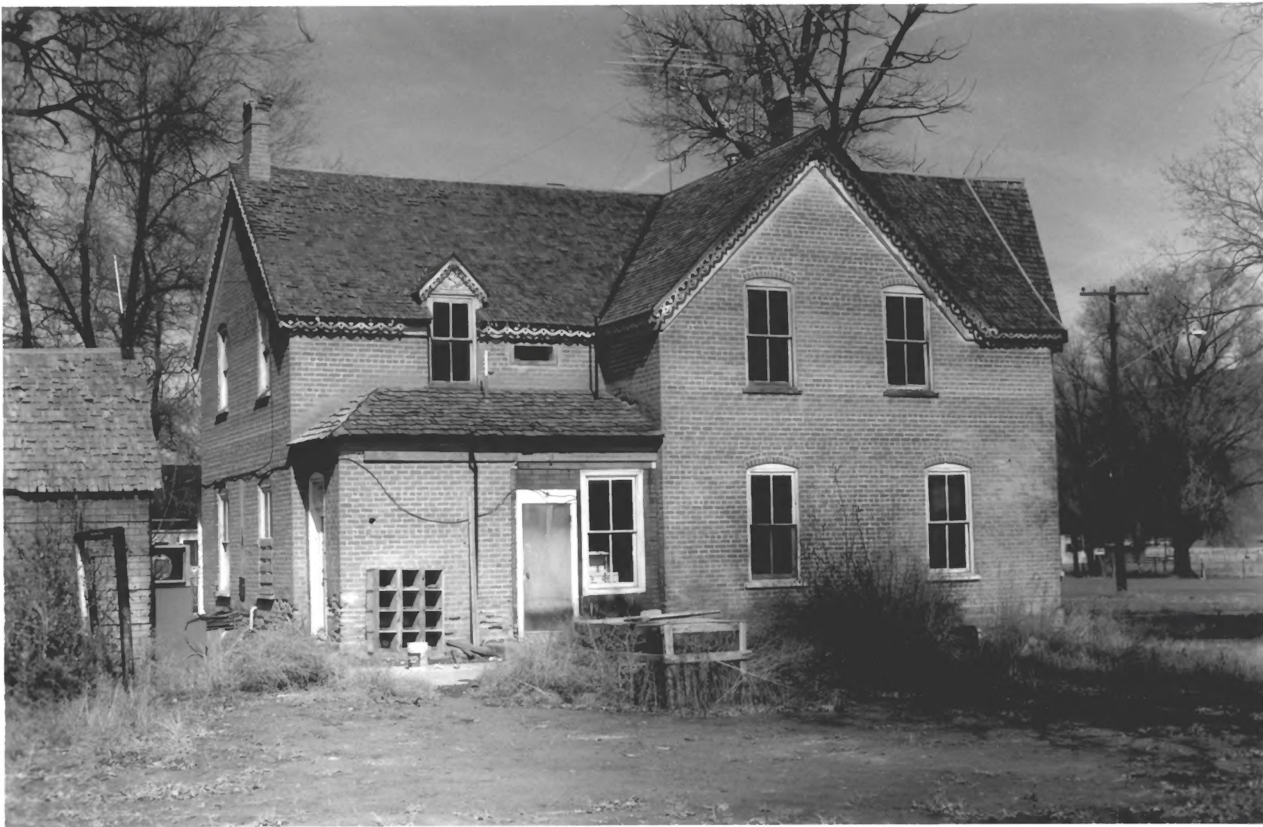
MORRILL, JOHN AND ELLA, HOUSE JUNCTION, PIUTE CO., UTAH PHOTO#2
