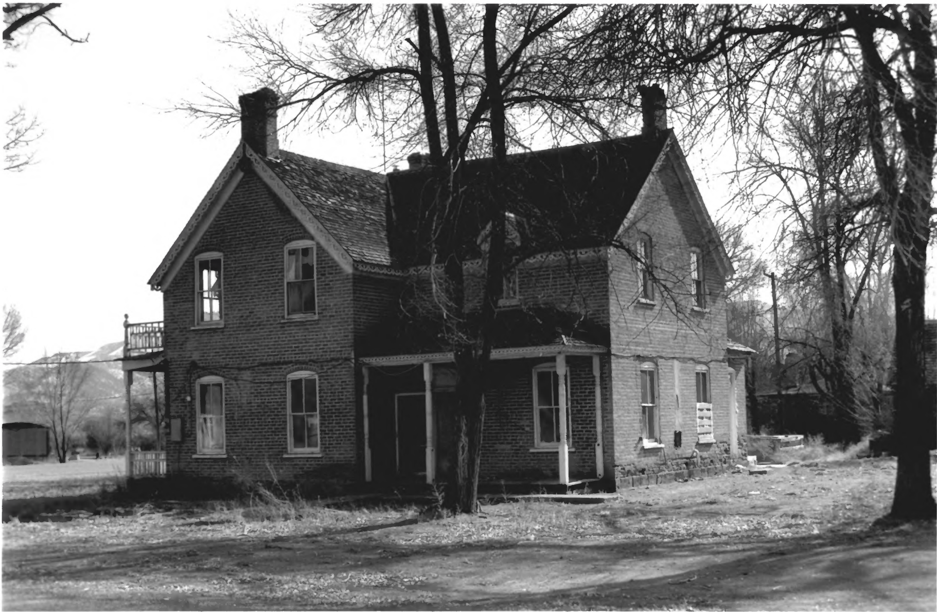
MORRILL, JOHN AND ELLA, HOUSE JUNCTION, PIUTE CO., UTAH PHOTO#3
