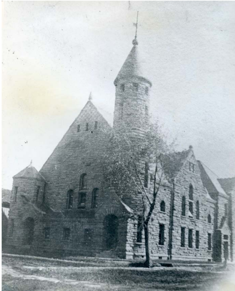
Figure 24: Photograph, c. 1910, showing First Methodist Episcopal Church, North, 119 West Fourth Street
