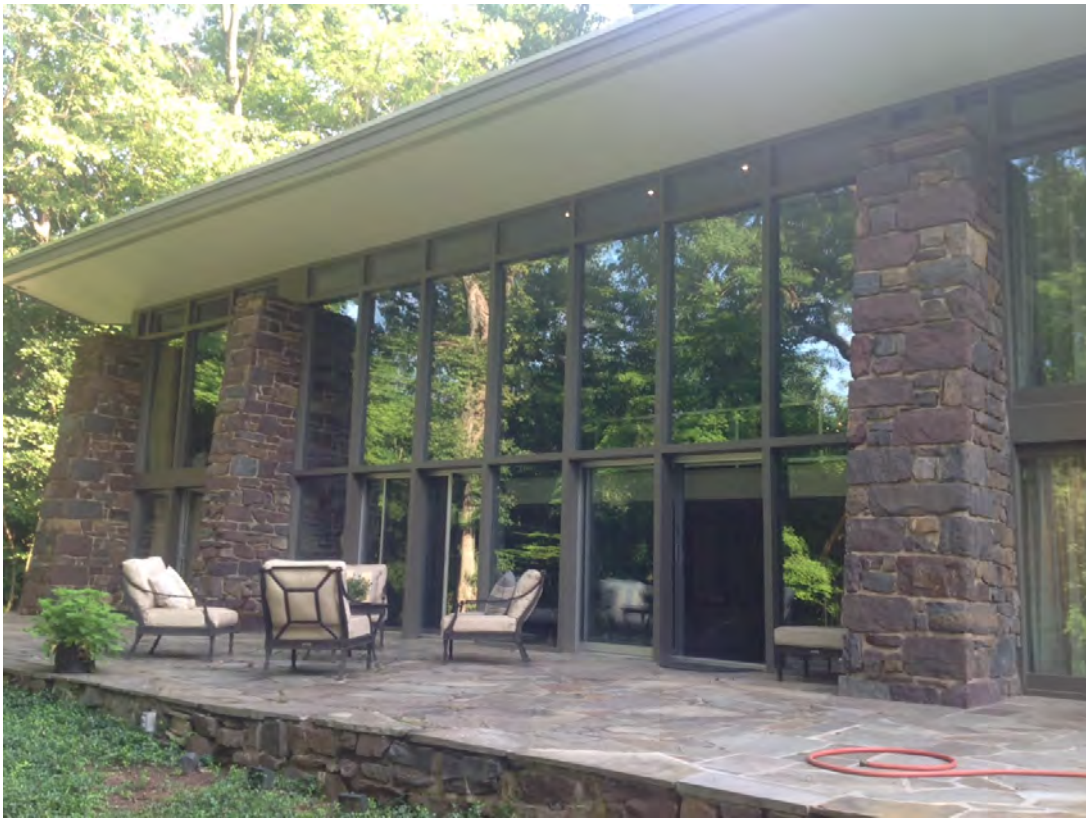
Photo 4. Façade (original sections) facing north
