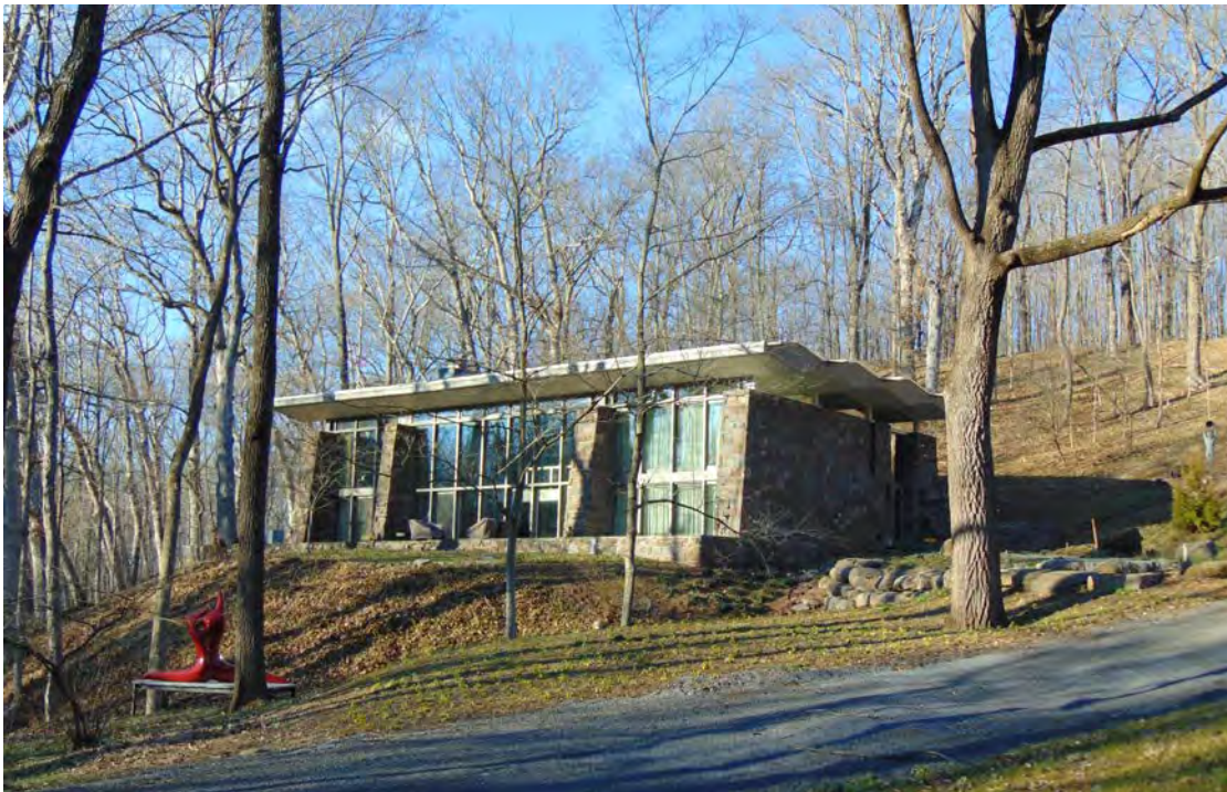
Photo 2. Façade of residence, similar view as above, 2017
