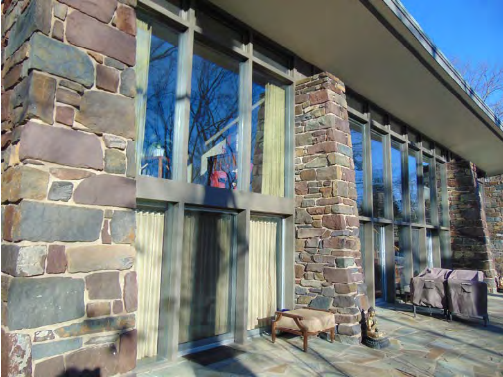
Photo 5. Façade (original sections) facing northeast
