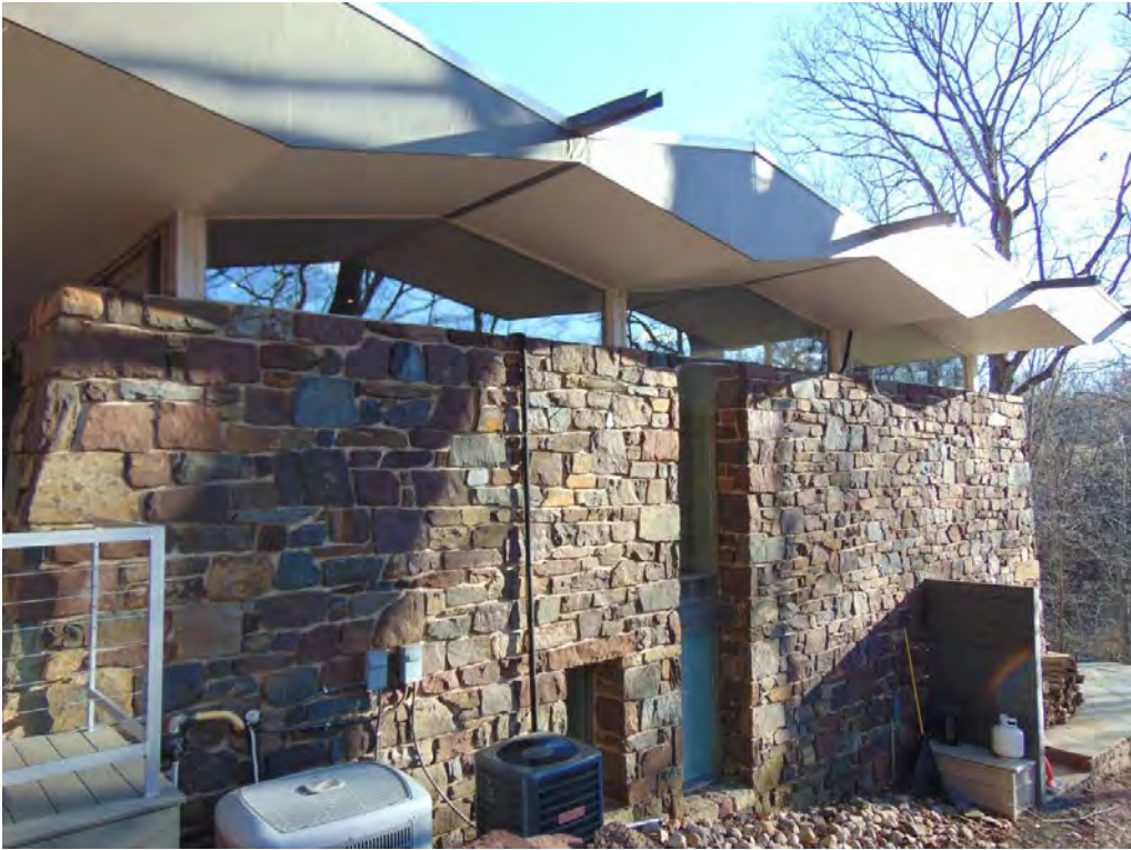
Photo 6. Westerly elevation facing east
