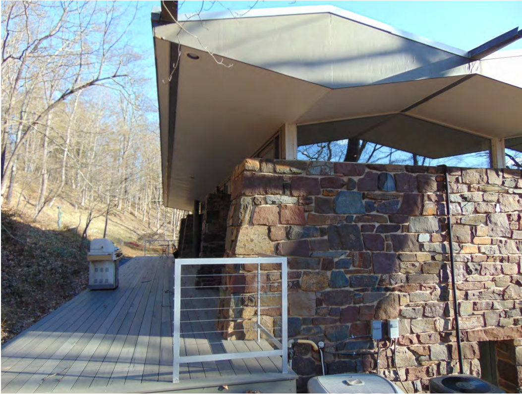
Photo 7. West corner facing northeast
