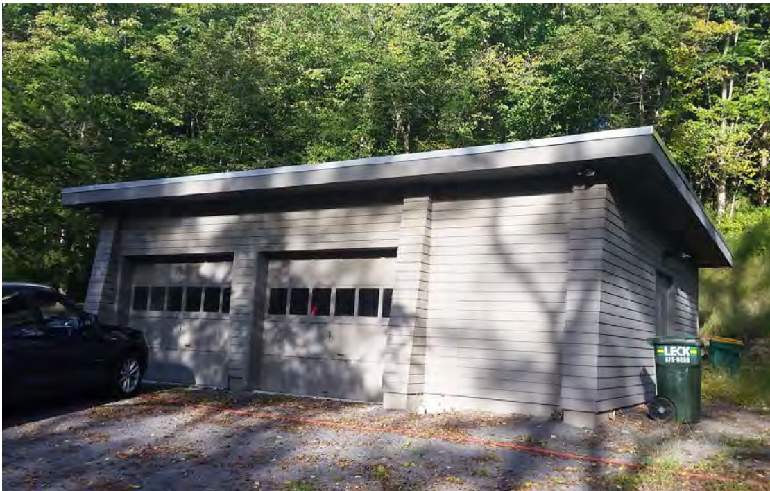
Photo 10 View of garage facing north
