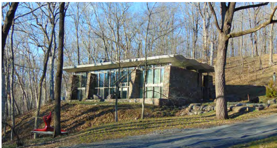
The house with the completed third bay addition.
