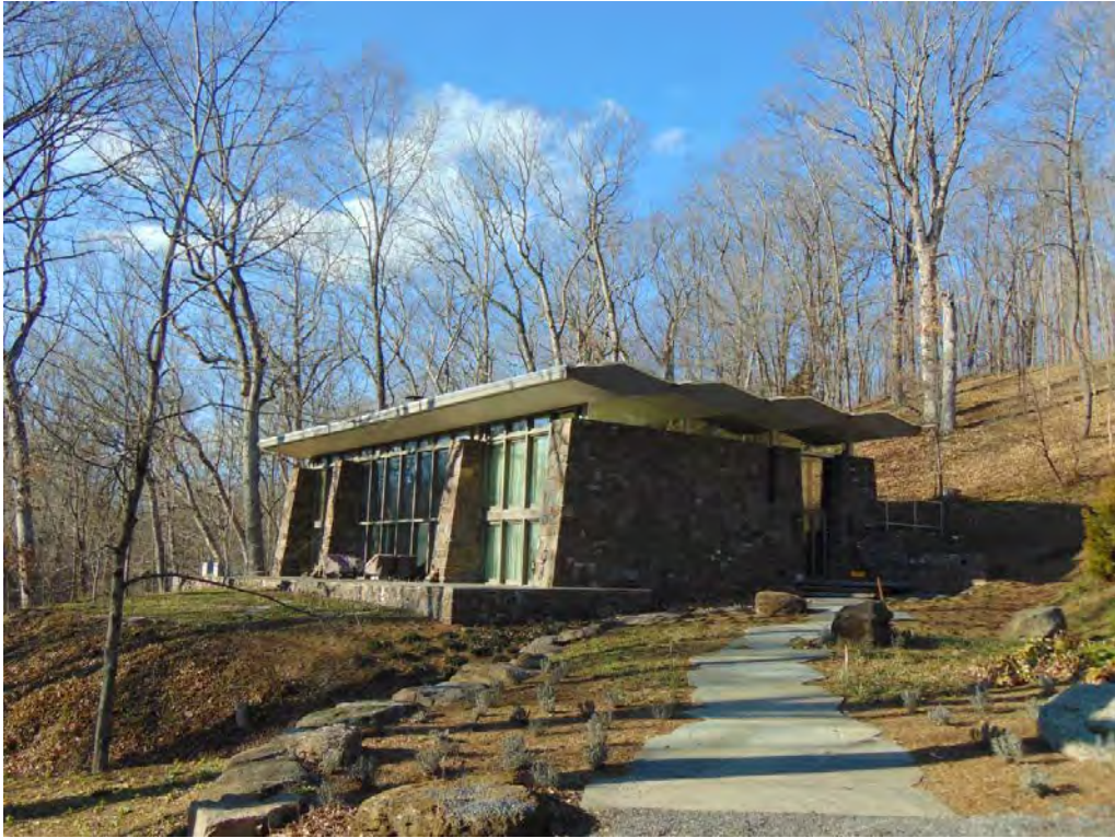
Photo 1. South corner of residence, 2017; recently completed final bay in foreground.
