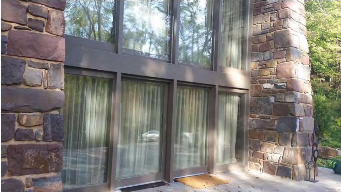
Photo 3. Southeast corner (new section) facing east
