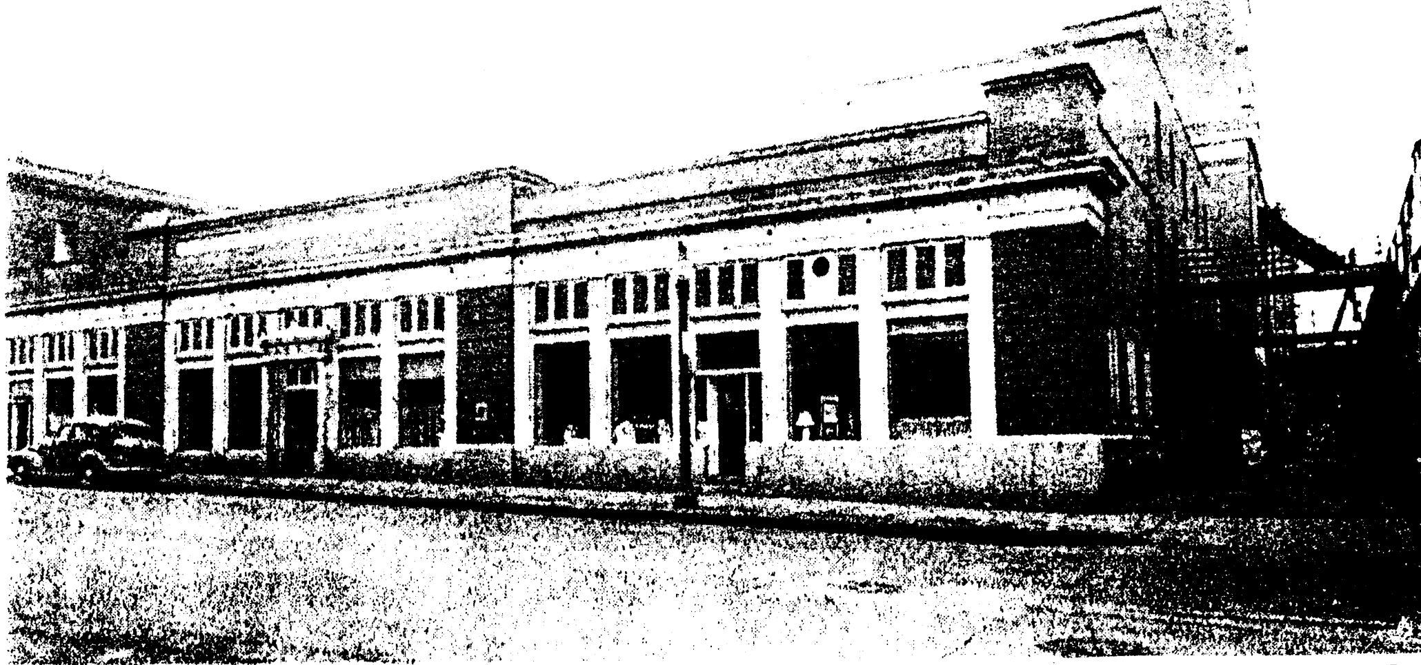
CENTRAL STEAM HEAT PLANT Adjacent Office Building 152-156 S. Post Street Spokane, WA Cutter & Malmgren, 1916 Photocopy: WWP Archives. ca. 1930's
