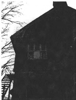
Detail, northwest elevation. Undated photo from www.abandonedbutnotforgotten.com , illustrating windows prior to being covered with plywood.
