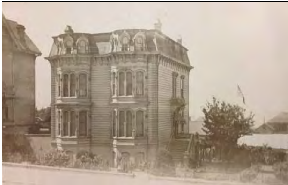
Figure 14. Burr House and garden, n.d. Note that additional windows have been added to bays on mansard roof. Source: Burr-Allyne family papers and photographs, 1839-2012 (bulk 1900-1930), California Historical Society.
