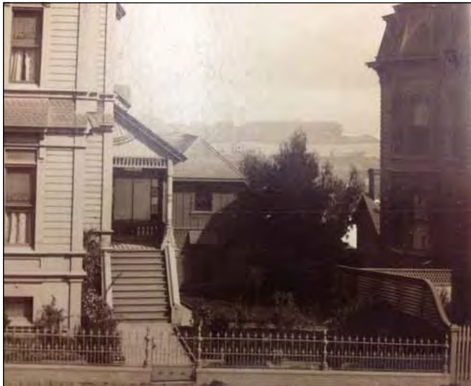
Figure 11. Burr house at right, view north, n.d.. Source: Burr-Allyne family papers and photographs, 1839-2012 (bulk 1900-1930), California Historical Society.
