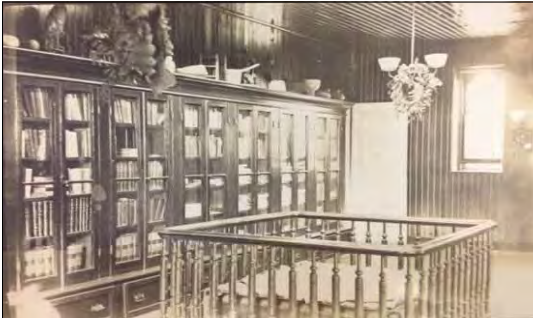
Figure 34. Third floor, n.d. Source: Burr-Allyne family papers and photographs, 1839-2012 (bulk 1900-1930), California Historical Society.
