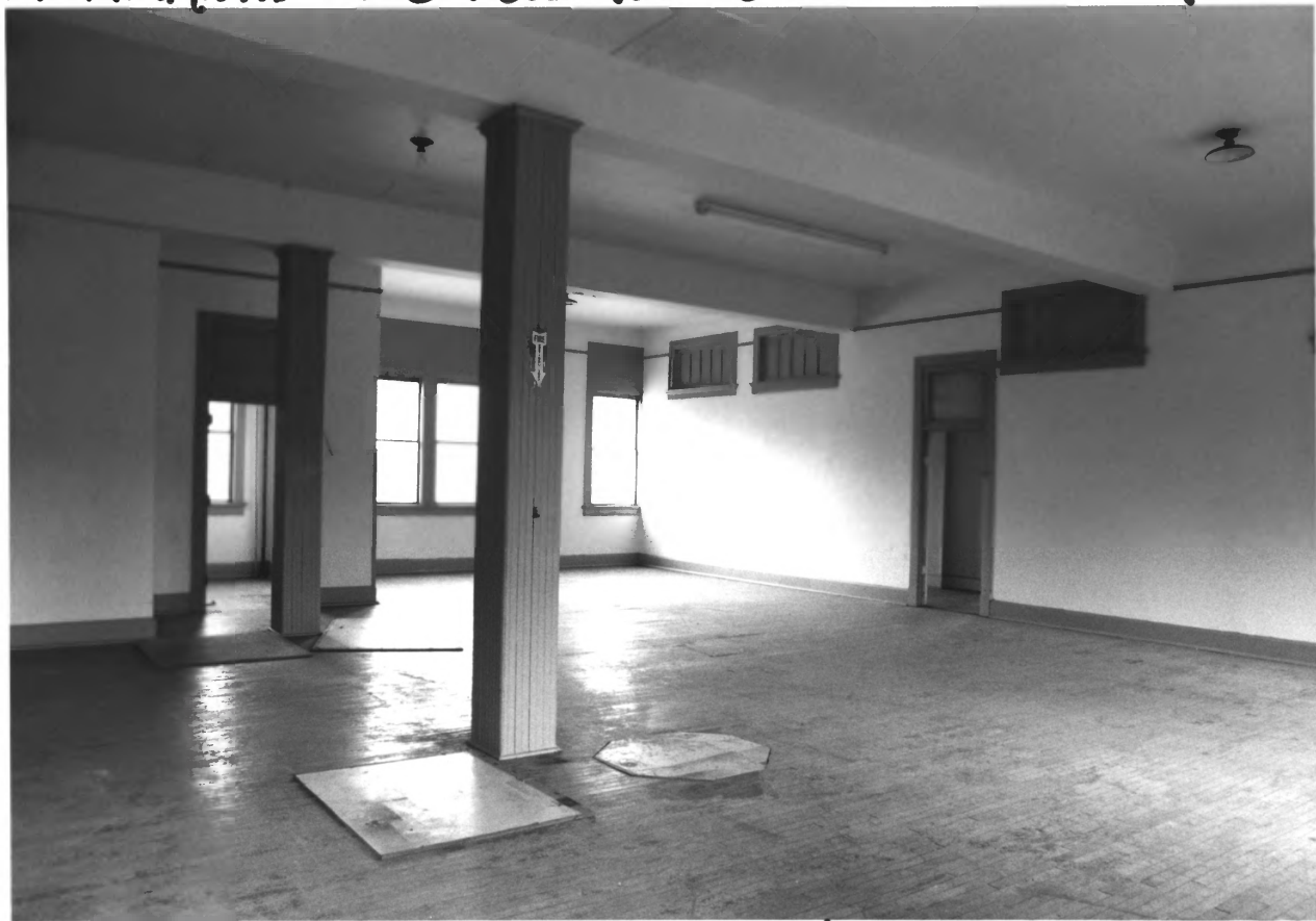
Garage Manton Co, IN photo 11
