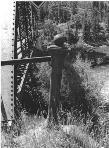
Photograph Number 0004. Detail of guardrail newel post. View to the south.
