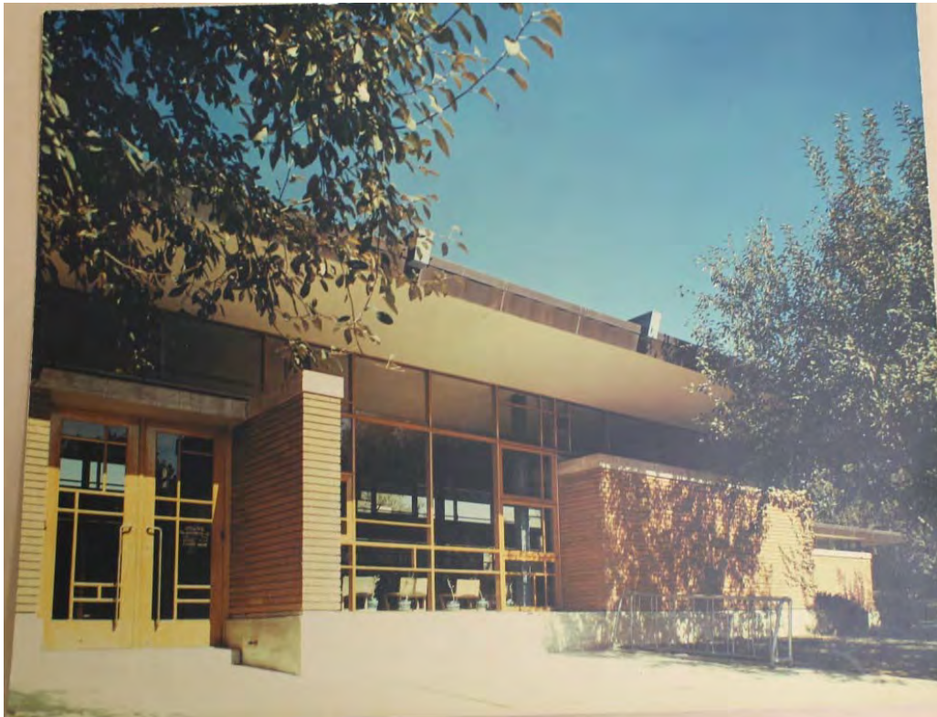
Figure 10: Ross-Broadway Library main entrance. Unknown date, but prior to 1990s alteration and installation of ADA-compliant ramp
