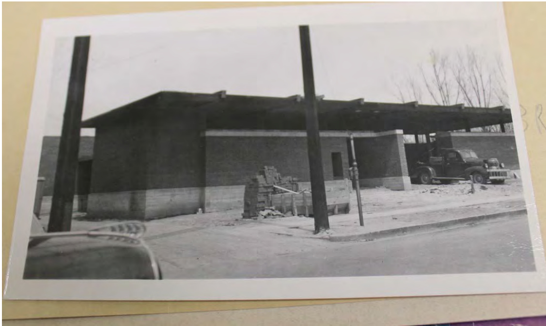
Figure 4: Ross-Broadway Library under construction, 1951.
