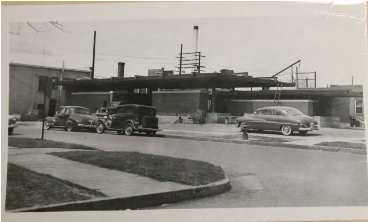
Figure 5: Ross-Broadway Library under construction, 1951.
