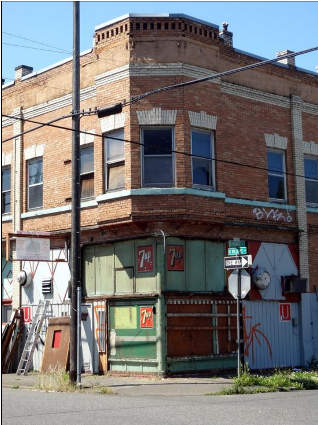
Figure 11: The Rinehart Building, 2013, showing the storefront treatment under the wood cladding.
