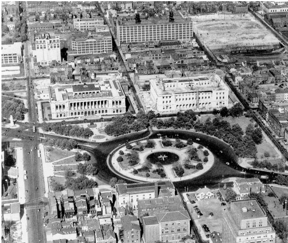
Photograph 38: Logan Circle, with the Municipal Court under construction; October 21, 1939. Free Library of Philadelphia, Print and Picture Department, Dallin, vol. 22, no. 12650. Courtesy of David B. Brownlee.
