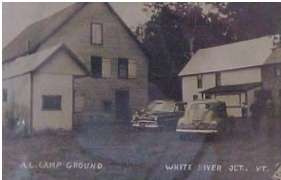
Figure 14. Dormitory, Kitchen and Bookstore
