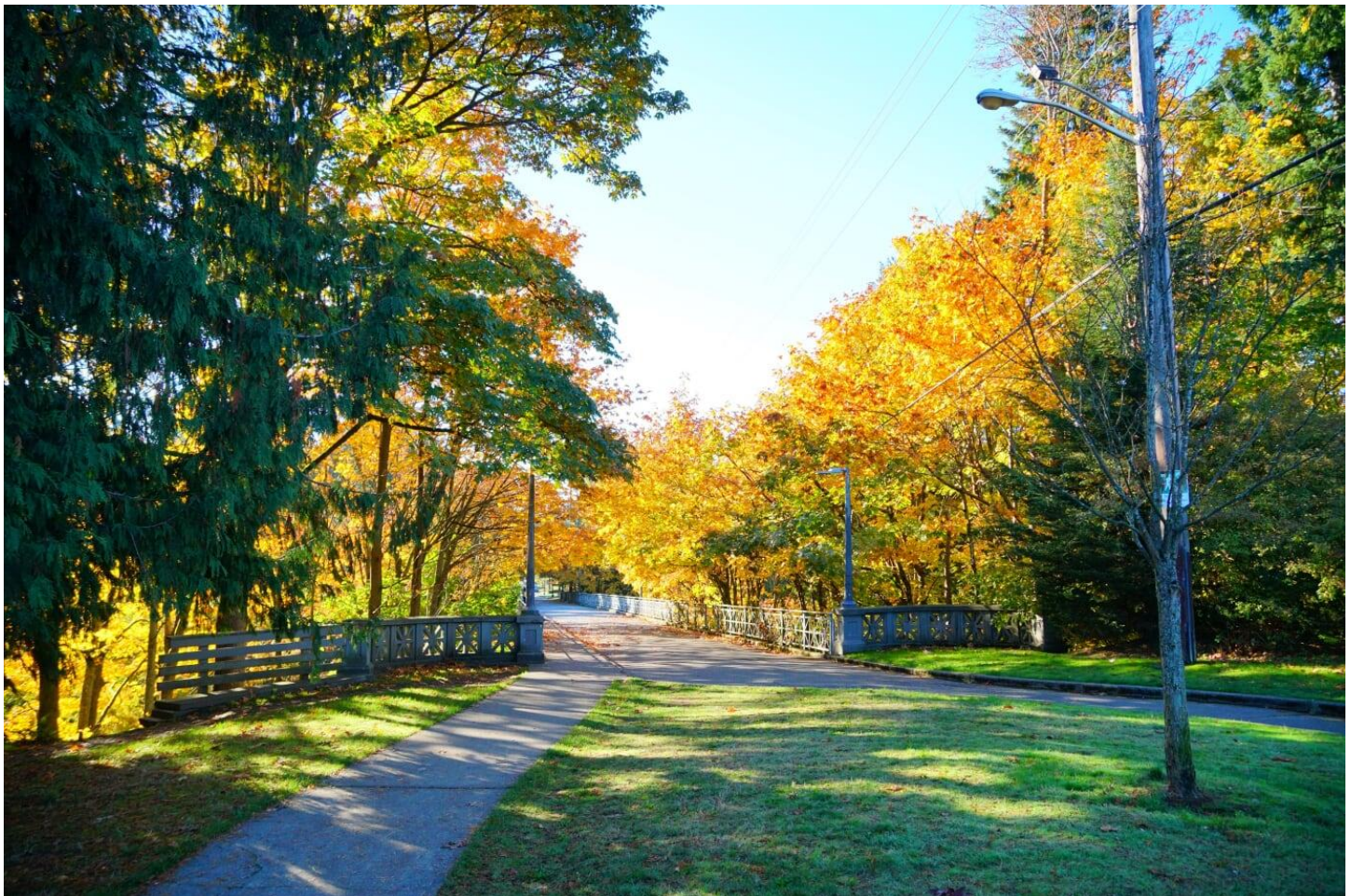
1 of 40 – Ravenna Park Bridge, 20 th Ave NE, view looking south.
