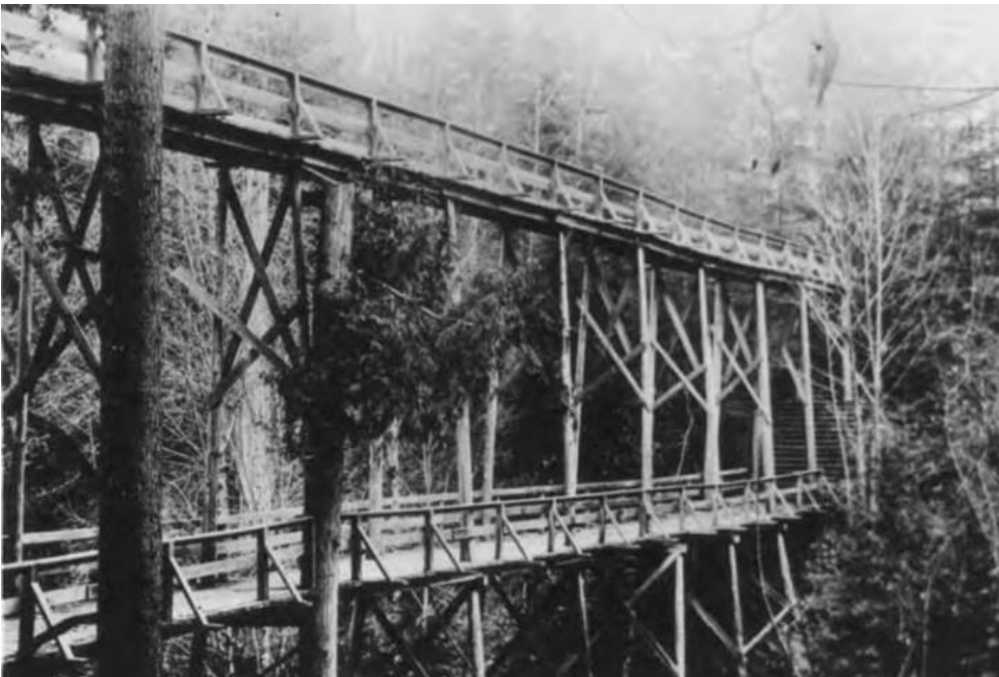
Cowen Park streetcar trestle and footbridge, ca. 1915 (Museum of History and Industry)
