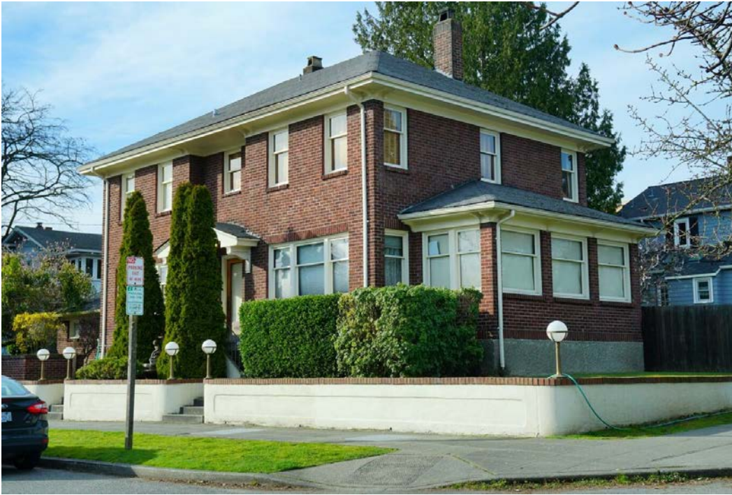
26 of 40 – Thelberg House at 1220 NE 63 rd Street.
