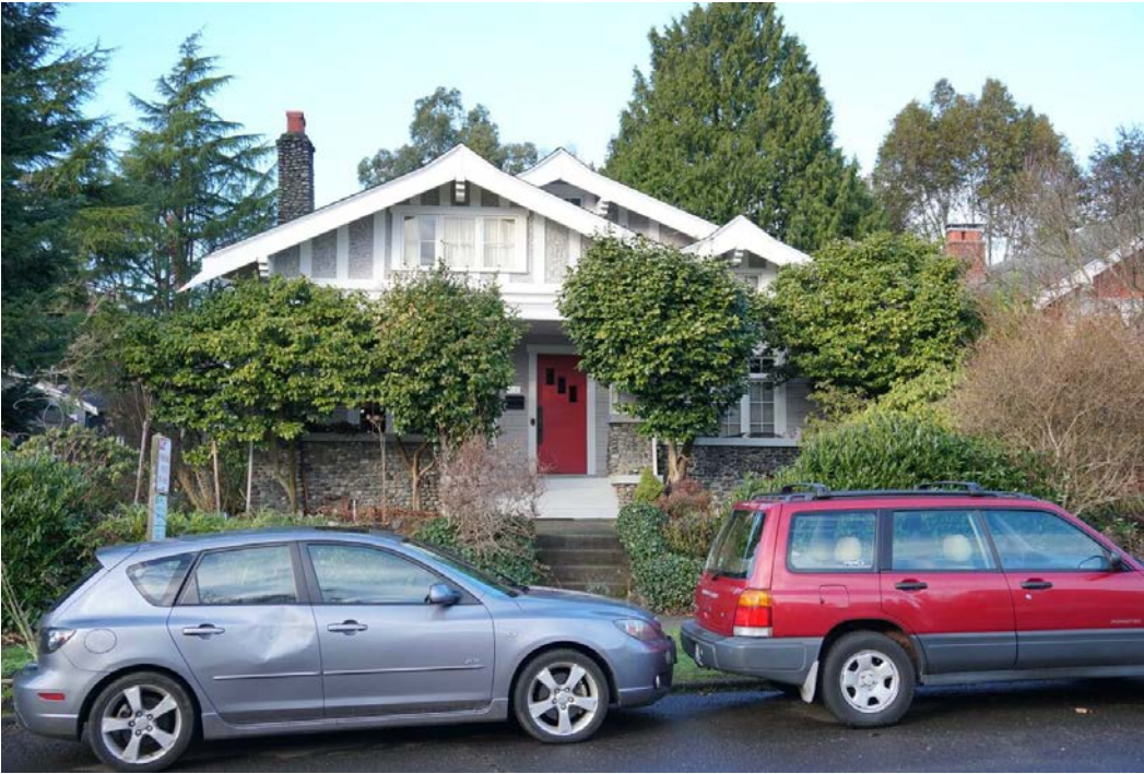
28 of 40 – Porter House at 1304 NE 63 rd Street.
