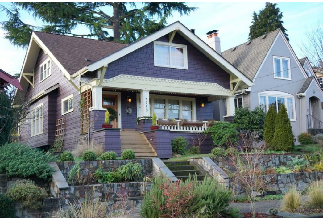
11 of 40 – Herbert Smith House at 6323 19 th Avenue NE.
