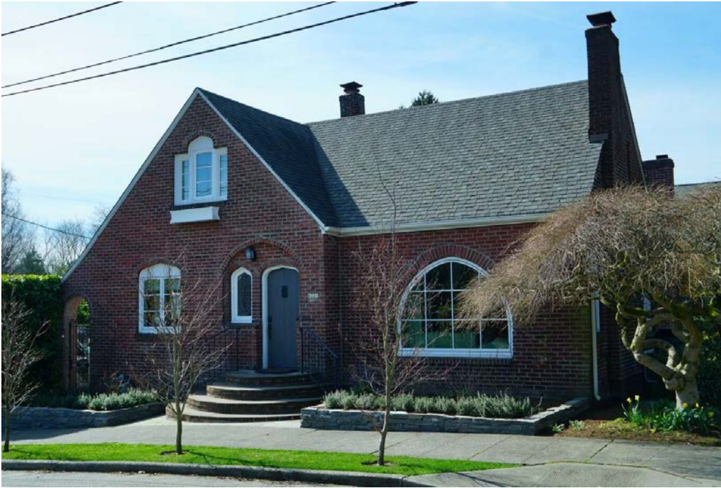
6 of 40 – Andrew Phillips House at 6221 17 th Avenue NE.
