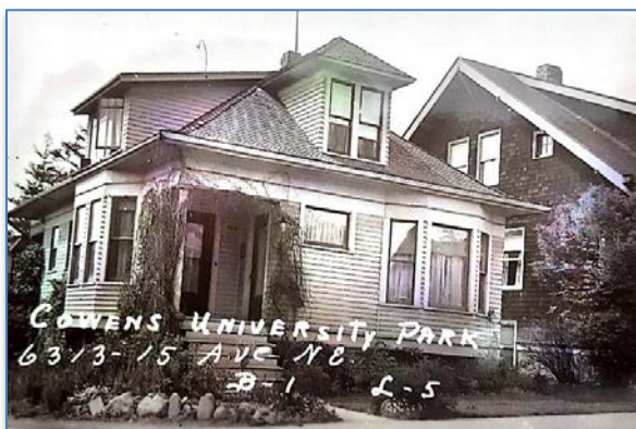
1937 view of 1907 single-family house
