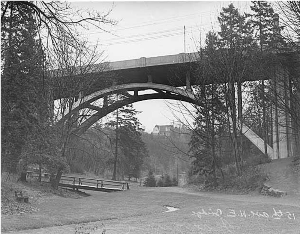
15 th Street Bridge (1937) viewing southwest, 1940 (Museum of History and Industry)
