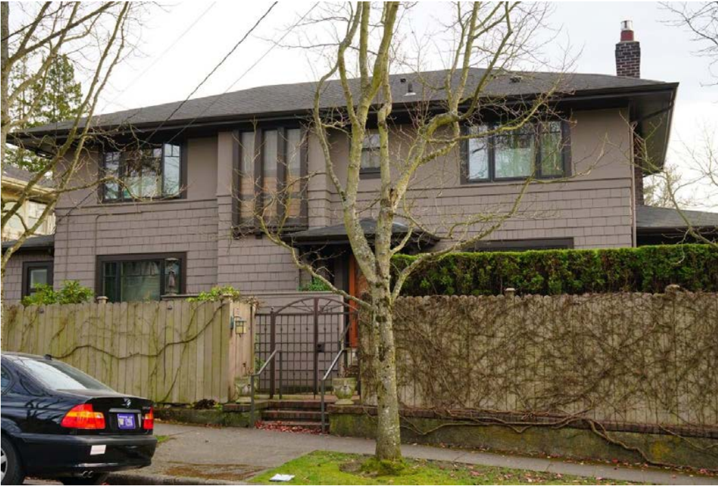
30 of 40 – Vincent House at 1711 NE 63 rd Street.
