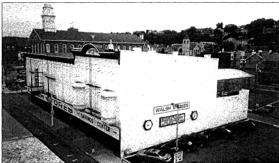
Figure 21: The Bell Block is at left center, view to the southwest with City Hall in the background.
