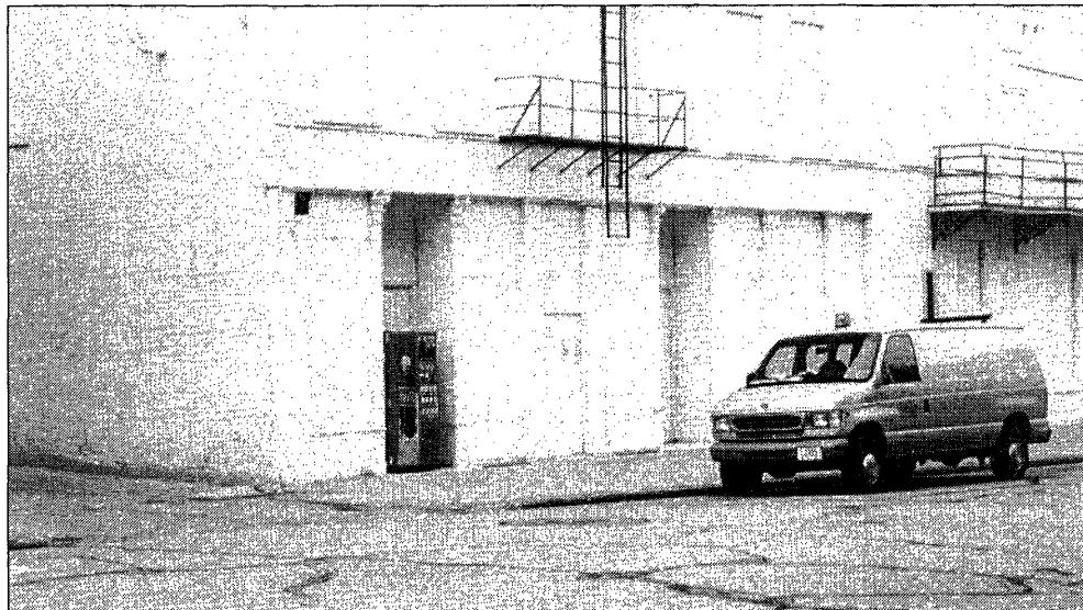
Figure 2: Stone lintel, south storefront, view northwest
