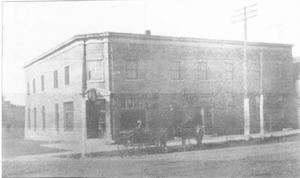
(Photo location #34) Circa 1914 image from Stuart Views . The telephone poles are now painted white to designate the early highway trail. (State Historical Society of Iowa, Iowa City)
