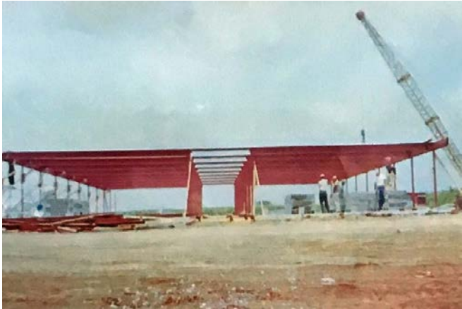
Figure 4. 1963 construction photos. Property of owner.
