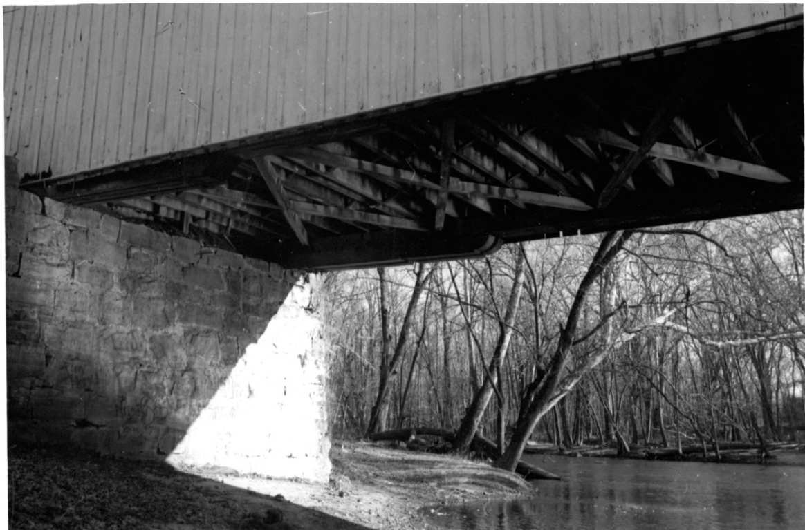
DARLINGTON COVERED BRIDGE - MONTGOMERY COUNTY - INDIANA #10
