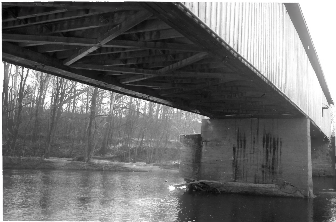
DARLINGTON COVERED BRIDGE-MONTGOMERY COUNTY-INDIANA #9
