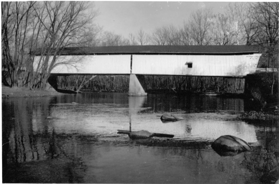
DARLINGTON COVERED BRIDGE- MONTGOMERY COUNTY- INDIANA # 5
