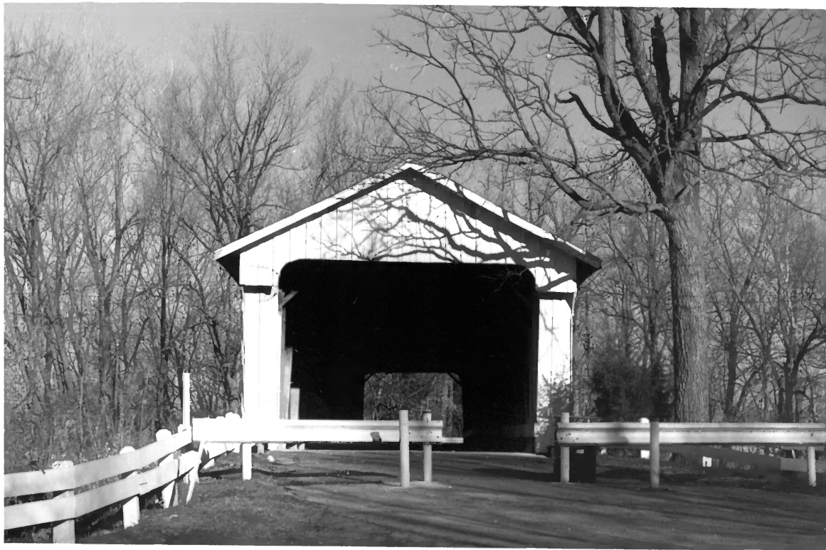
DARLINGTON COVERED BRIDGE - MONTGOMERY COUNTY - INDIANA # 3
