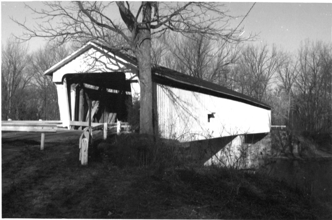
DARLINGTON COVERED BRIDGE - MONTGOMERY COUNTY - INDIANA #2
