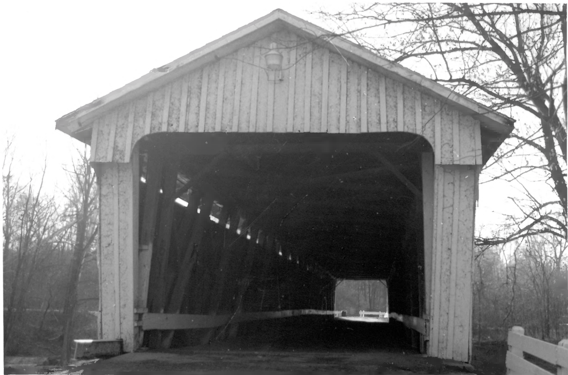
DARLINGTON COVERED BRIDGE - MONTGOMERY COUNTY - INDIANA # 8
