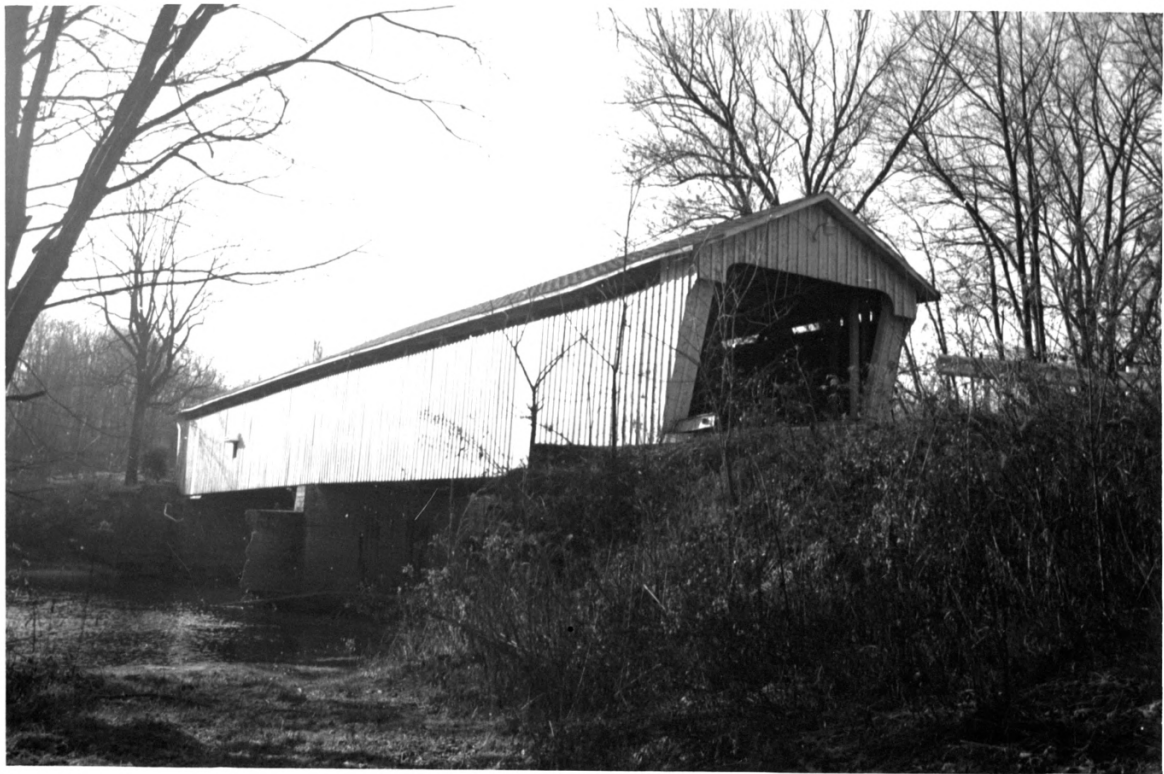
DARLINGTON COVERED BRIDGE-MONTGOMERY COUNTY-INDIANA #6
