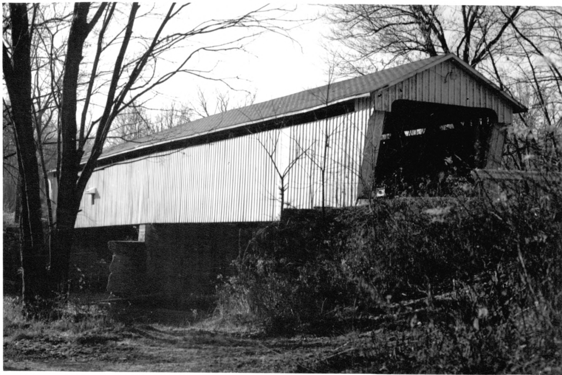
DARLINGTON COVERED BRIDGE-MONTGOMERY COUNTY-INDIANA #7
