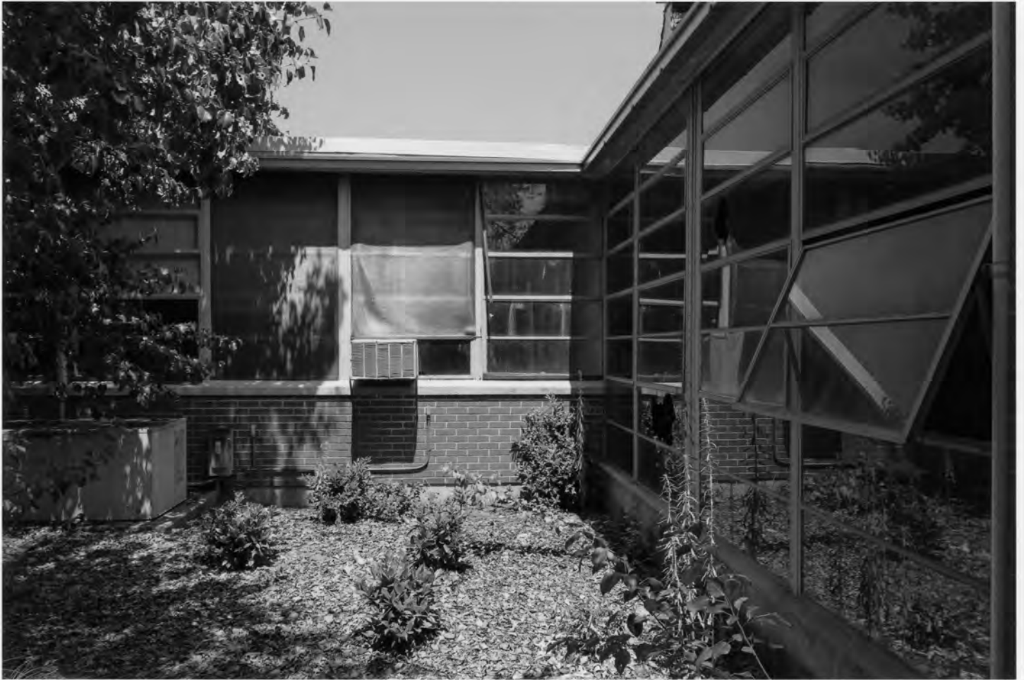
Vienna High and Industrial School Dooly County, Georgia Photograph 34 of 42
