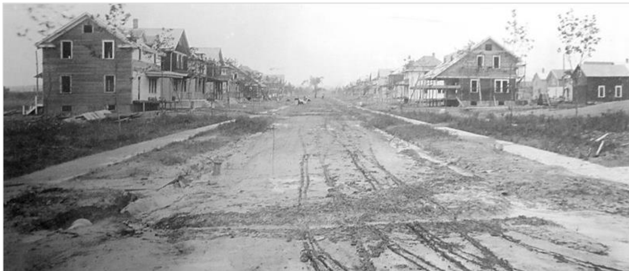
Figure 15b. View looking southerly along Silliman Avenue from Main Street, 1913
