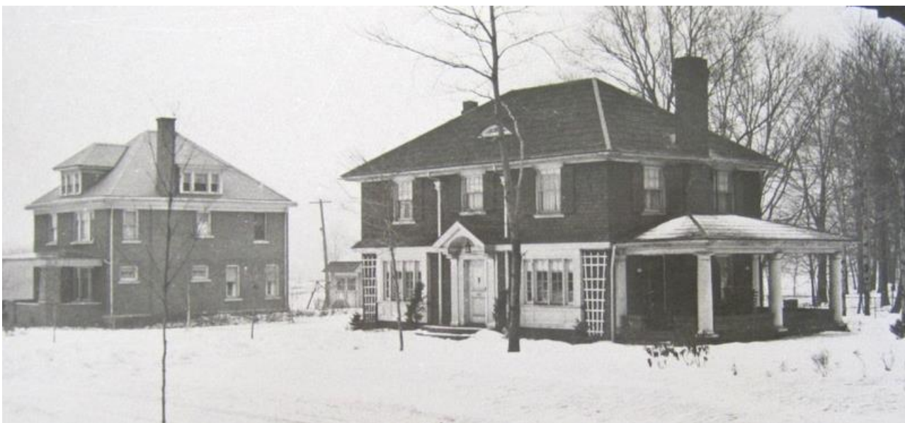
Figure 22b: View looking northeast at 535 Rankine Avenue House (#174) and 591 Rankine Avenue House (#175), Photo undated
