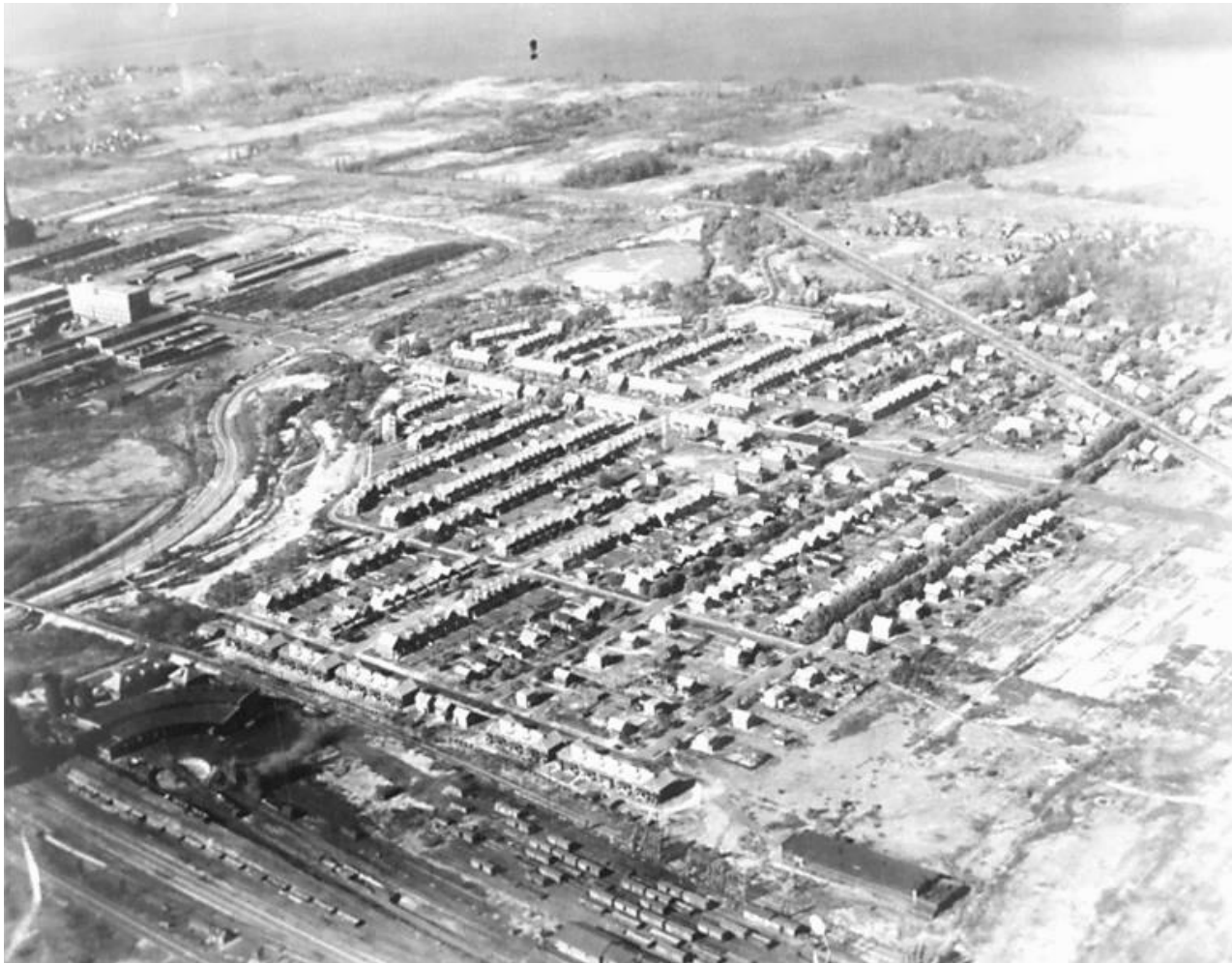
Figure 13. Lawrence Park, view facing northwest. Photo undated
