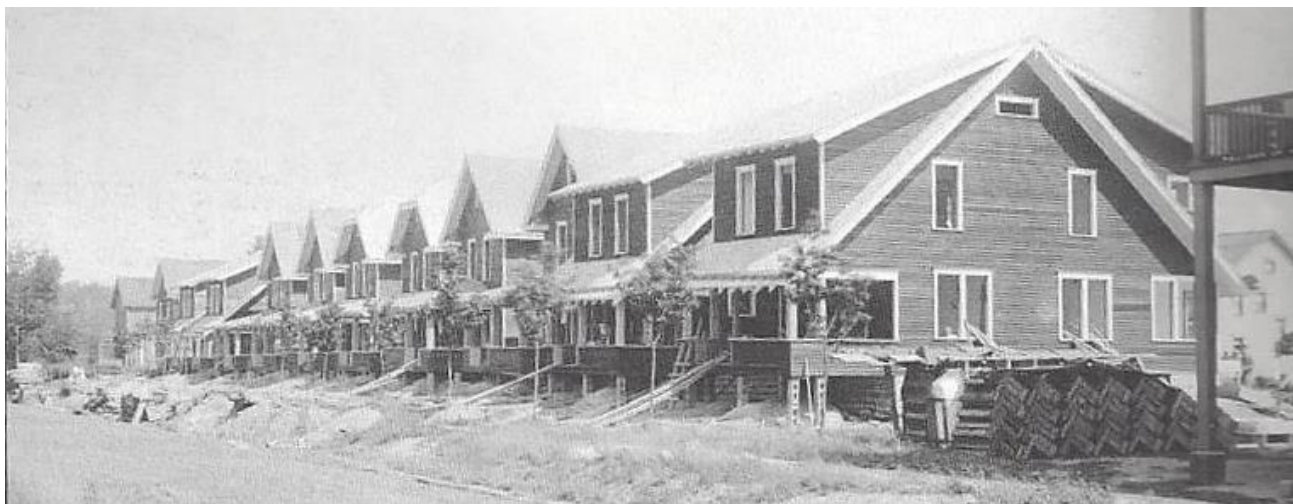
Figure 18a. View looking northerly along Rankine Avenue from Main Street, showing houses under construction by builder Edward B. Lee. Photo 27 August 1917
