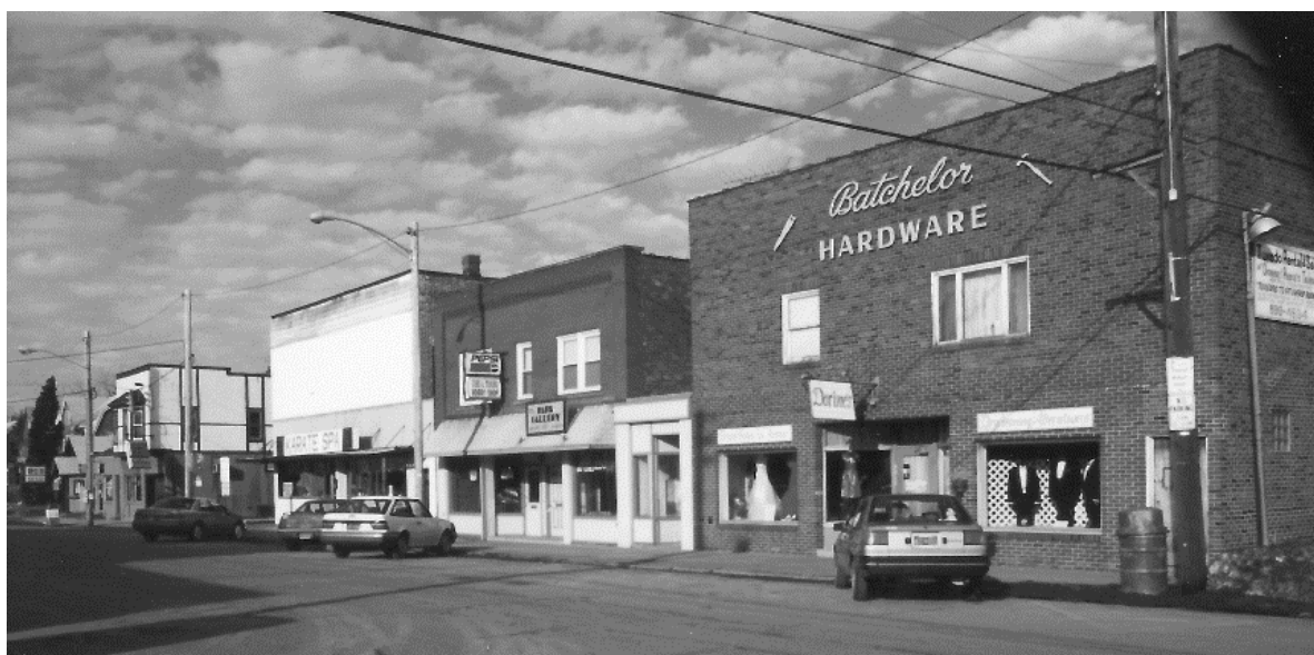
Figure 32b. Streetscape with Batchelor Hardware, 4012 Main Street (#443), 2 nd story addition 1950, Photo undated
