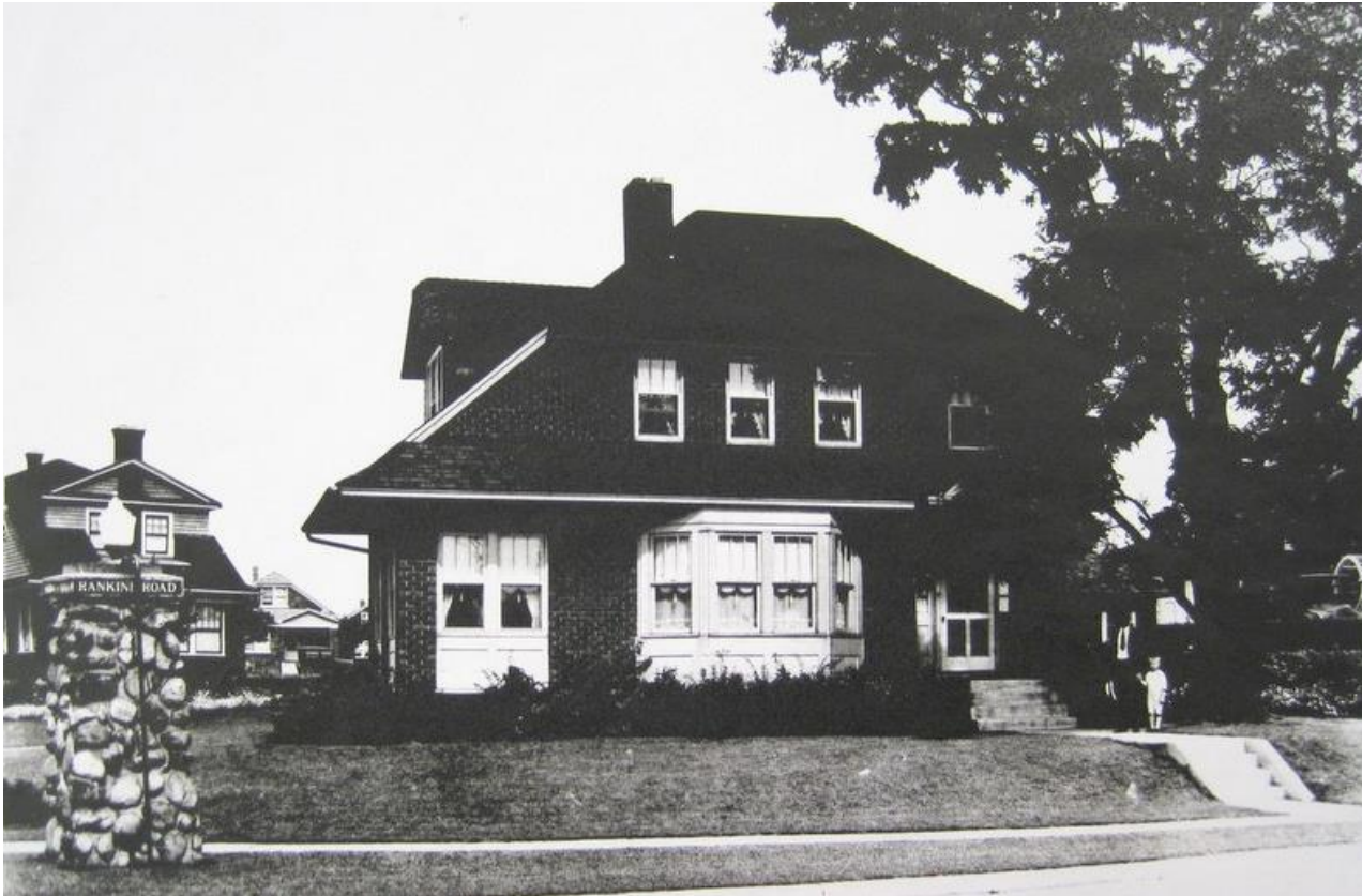
Figure 24. 511 Rankine Avenue House (#170) at East Lake Road showing Stone Piers (#474) with light, Photo 23 August 1928
