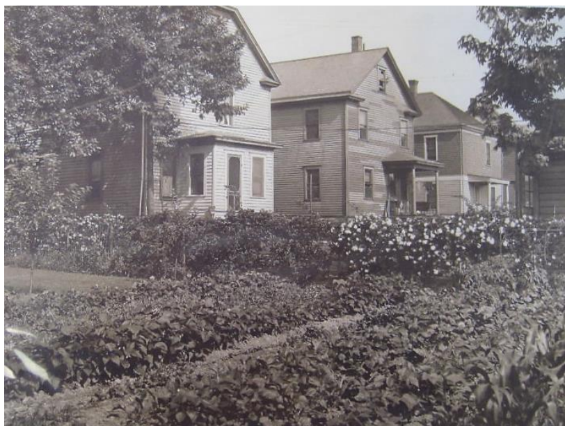
Figure 20b. Backyard of houses with gardens on Rankine Avenue, Photo Summer 1923
