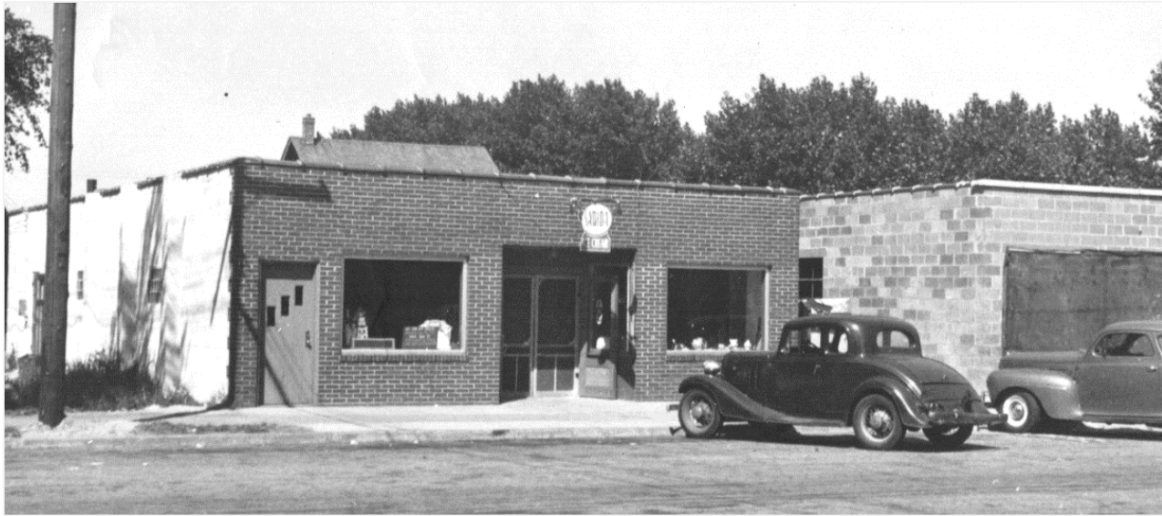
Figure 33. 4108 Main Street (#451), Photo 1940s
