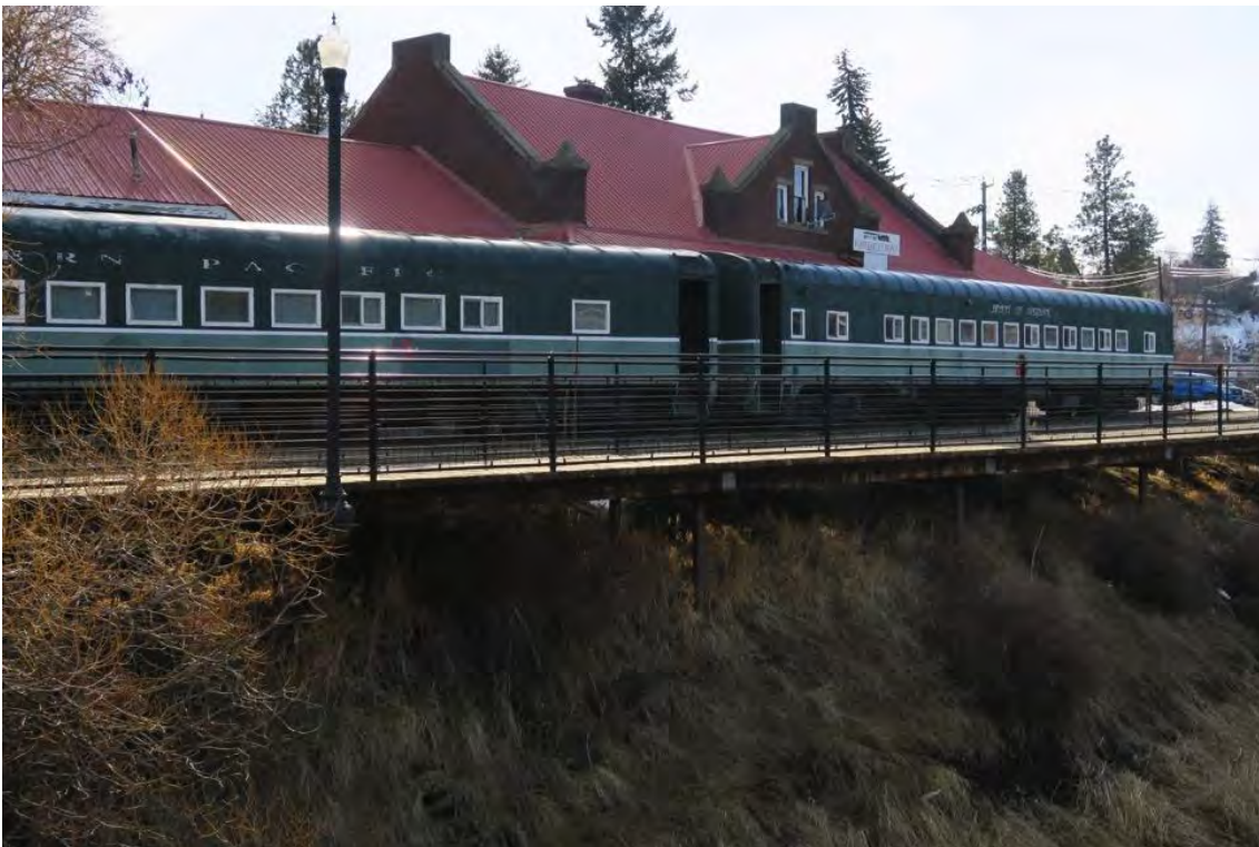
7 of 35: Depot trackside. View of west elevation, two cars slated for removal, camera looking southeast.
