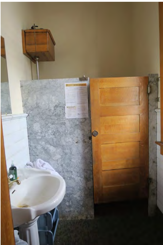
19 of 35: Interior-south end of depot, women's restroom, camera looking north.
