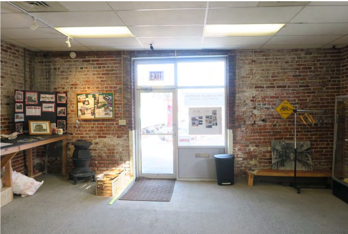
23 of 35: Interior-freight room main entry door, camera looking north.
