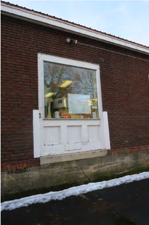
10 of 35: East elevation. Freight Room door opening, camera looking west.
