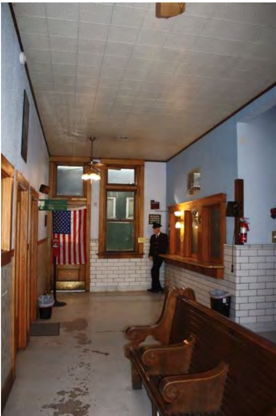
13 of 35: Interior - north end of general waiting room, center section ticket windows, camera looking west.
