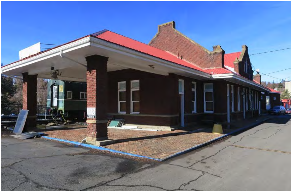
2 of 35: Covered Platform and east elevation. View from south end, camera looking northwest.
