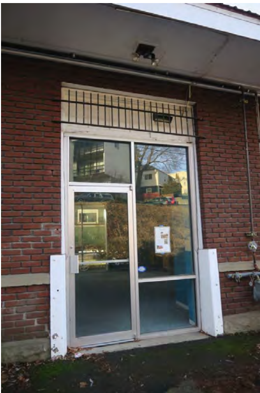
9 of 35: East elevation. Baggage Room door opening, camera looking west.
