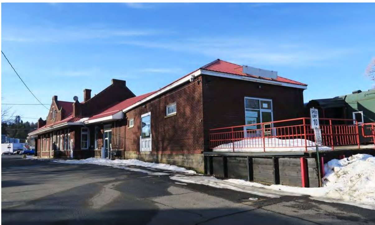
3 of 35: Freight Room platform and east elevation. View from north end, camera looking southwest.
