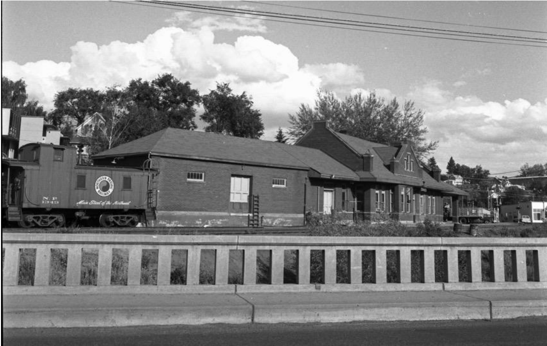
View of Pullman depot freight room looking to the southeast. Robert Johnston Photo, Ainsworth Collection at PNRA. Photographed June 1969.
