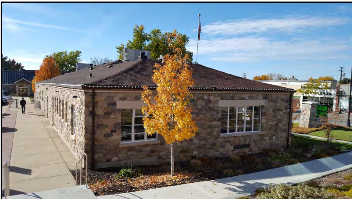
6 of 19. North and east elevations. Camera facing southwest.
