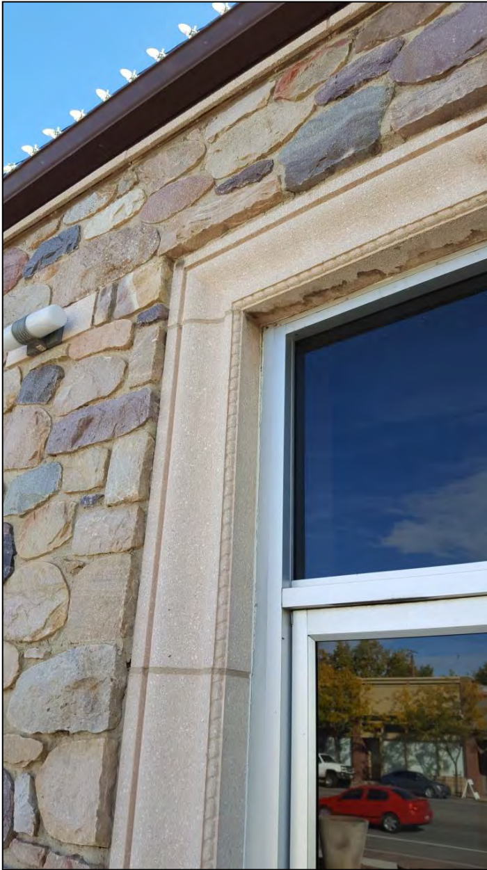
11 of 19. Terra cotta door surround detail. Camera facing northeast.
