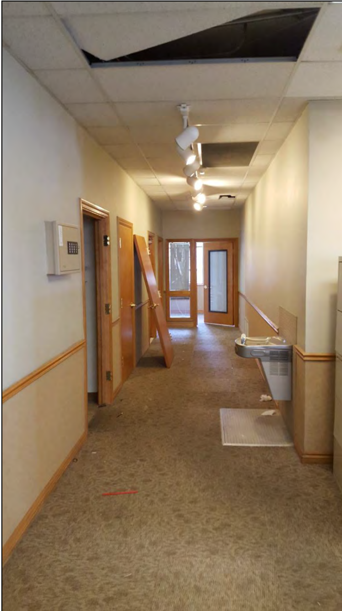
14 of 19. Interior, south hallway. Camera facing south
