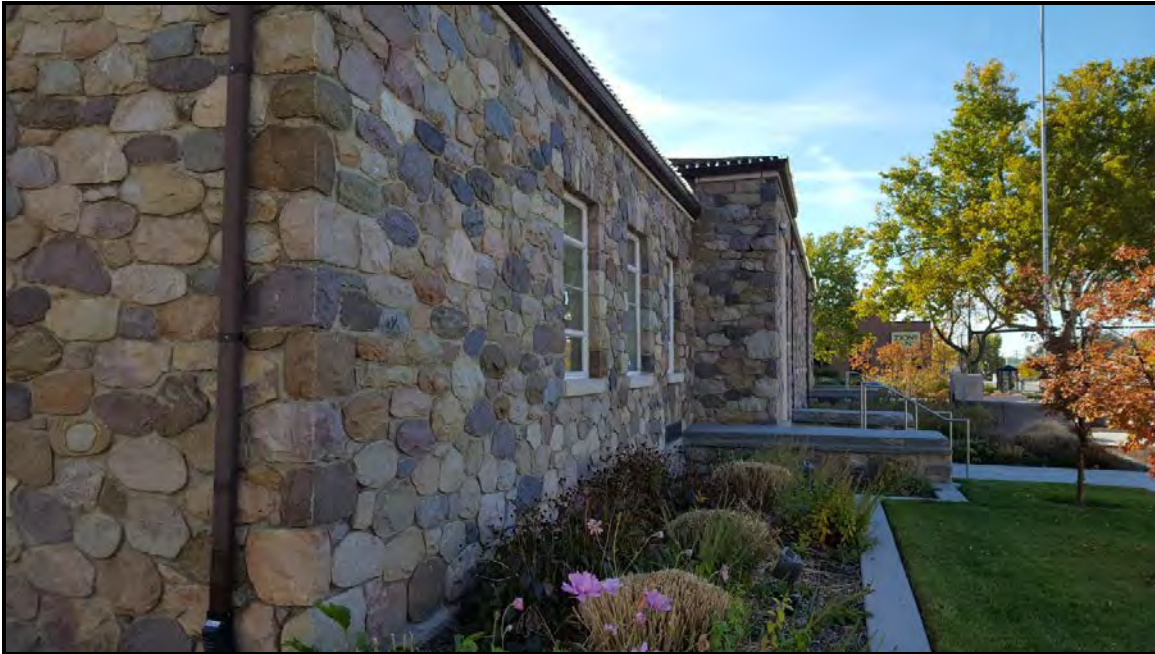
5 of 19. Partial north and west elevations—stonework detail. Camera facing south.
