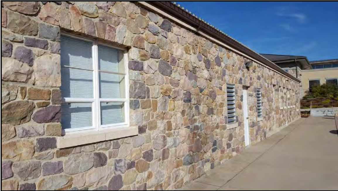
9 of 19. East elevation detail. Camera facing northwest.
