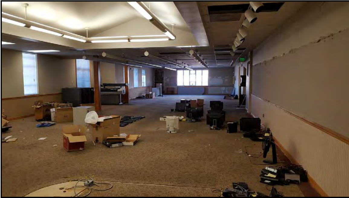
12 of 19. Interior, main space. Camera facing northwest.
