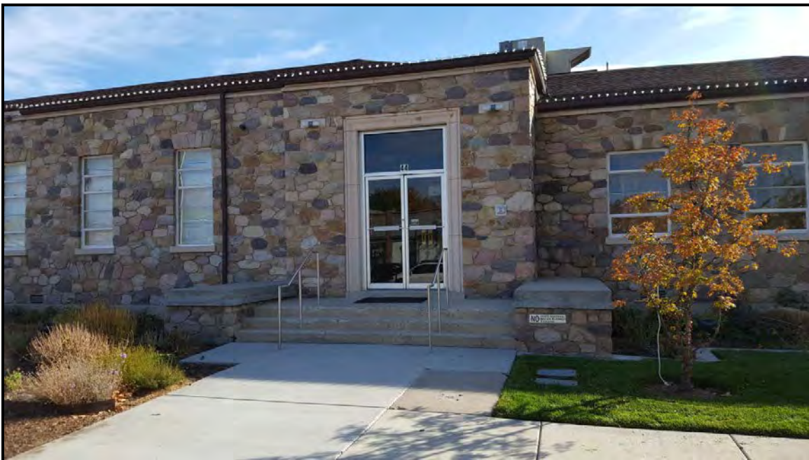
2 of 19. West elevation detail, right (south) entrance. Camera facing northeast.
