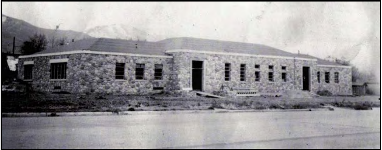
Figure 3. Kaysville City Hall under construction, c. 1940-41. (Photographer unknown).
