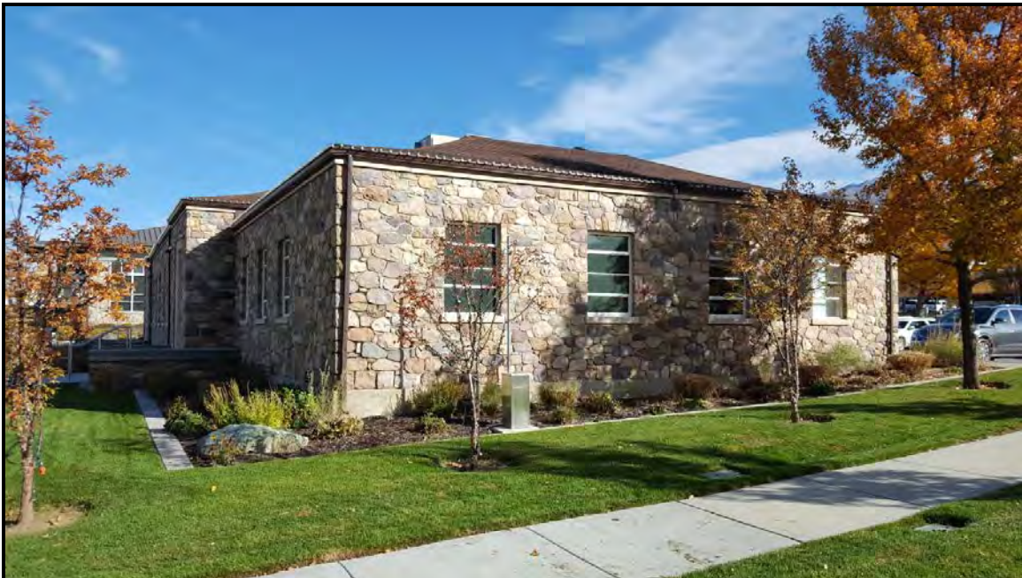
10 of 19. South elevation. Camera facing northeast.
