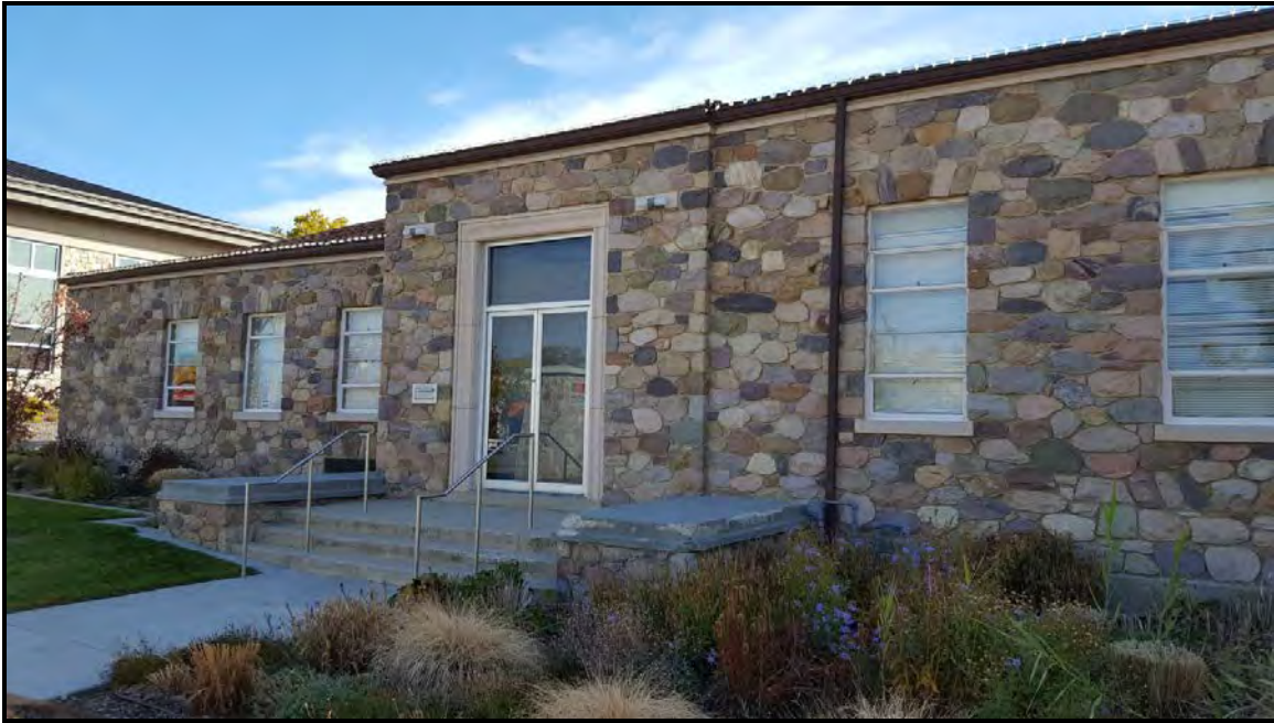
3 of 19. West elevation detail, left (north) entrance. Camera facing northeast.
