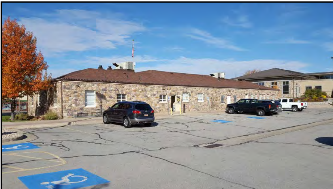
8 of 19. East elevation. Camera facing northwest.
