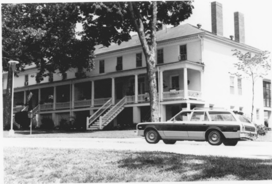
"The Rookery", Bldg. # 19. Built ca. 1834. Oldest building still extant at Fort Leavenworth. The first governor of Kansas, Andrew Reeder, lived in this building in 1854.
