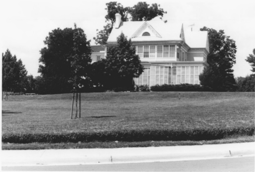
Commanding General's House. Building # 1 was built in 1861 to house the Commanding Officer, Fort Leavenworth Arsenal. Additions and modifications have been made through the years.
